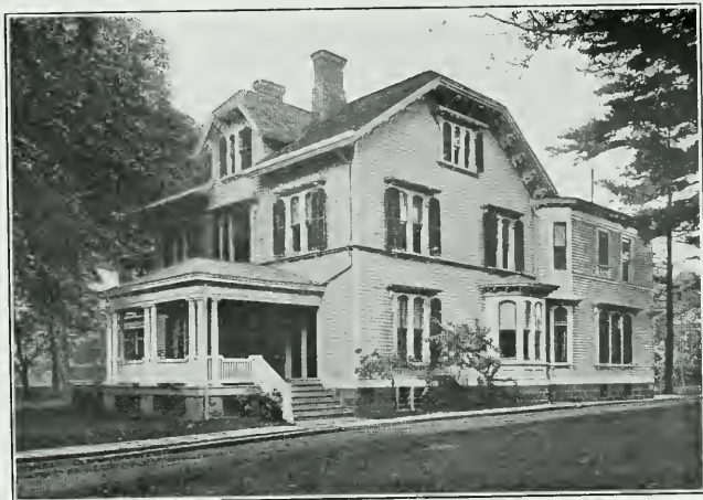
Frame House Before Treatment With the Cement Gun
