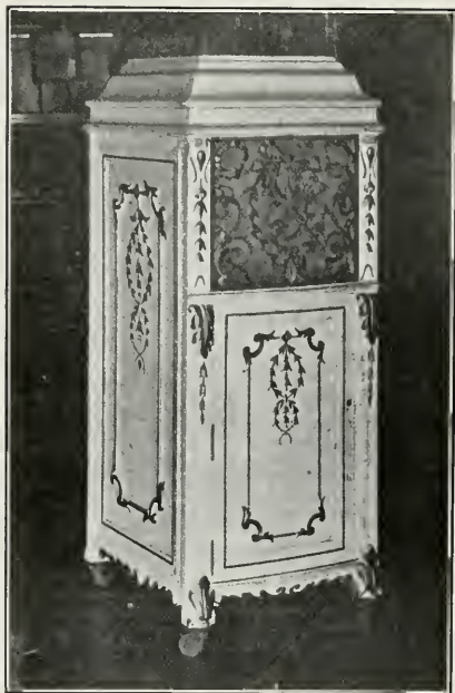
The Edison Phonograph Cabinet of Reinforced Concrete
