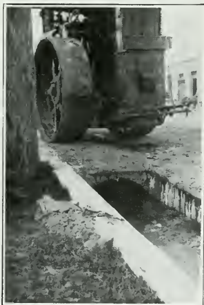
Part circle, with 30-inch base and 7-inch rise at center, made of 14 gauge iron, supporting 14-ton roller. Culvert installed in city of San Bernardino.
