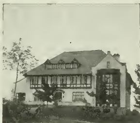
Residence of Mr. Alex. Pantages, Seattle, Wash. Loteless & Wilson, Architects Neponset Waterproof Building Paper Used.
