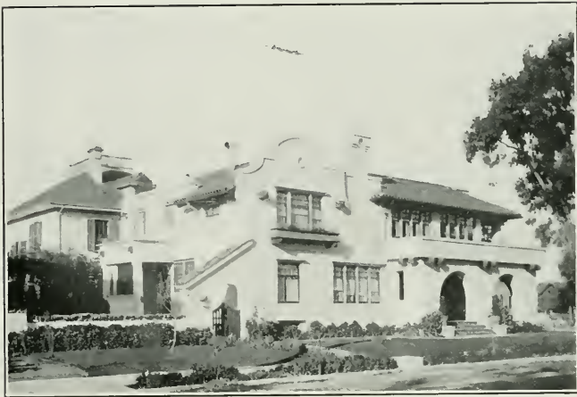
South View, Hartman Residence, San Jose, California Henry C. Smith, Architect
