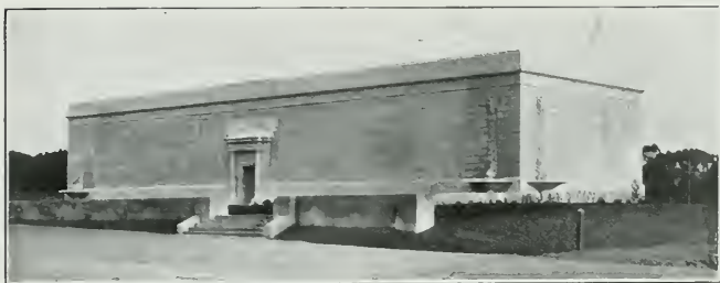
Sloat Boulevard Pumping Station, San Francisco Willis Polk & Co., Architects
