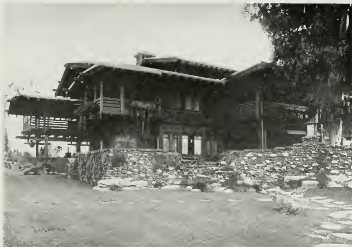
Residence of Mr. D. B. Gamble Greene & Greene, Architects, Pasadena, California
