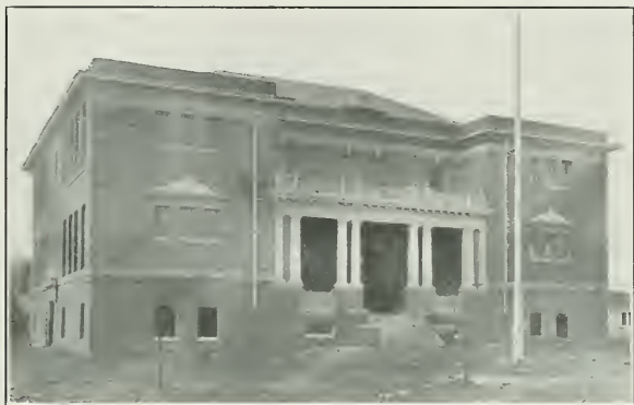
Grammar School, Petaluma, California Designed by Henry C. Smith, Architect
