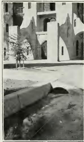
Corrugated iron culvert at Riverside, California, installed in front of famous Glenwood Mission Inn
