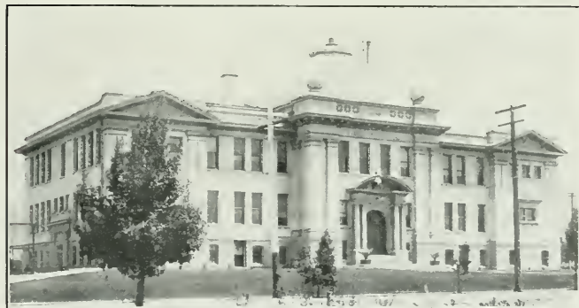
Whittier High School, Whittier, California Designed by Henry C. Smith, Architect
