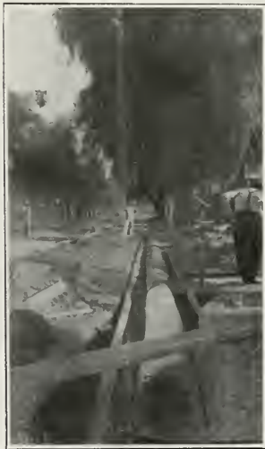
Part circle Culvert, 16 gauge, 14-inch base by 7-inch rise, 68 feet long, with two tees 17 feet long, at Sixth and Lime streets, city of Riverside
