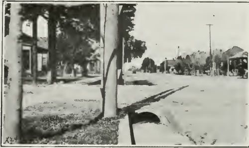
Corrugated culvert, 24 x 10 inches, installed in city of San Bernardino
