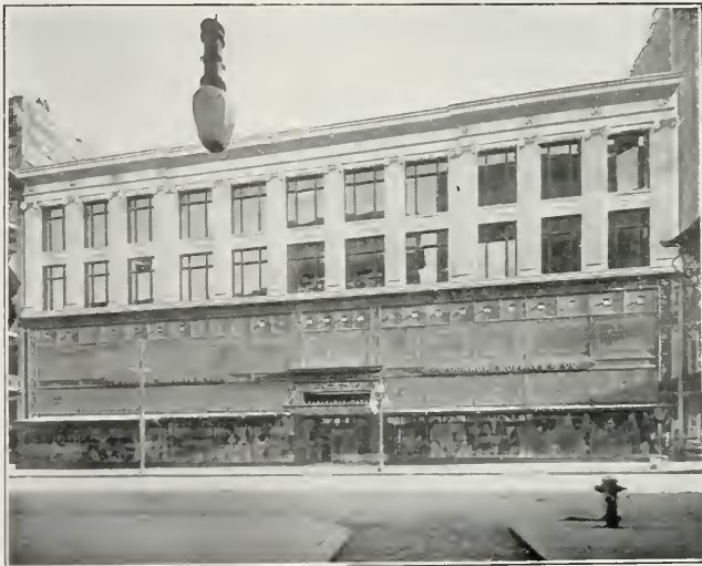
Building for Drexler and Preston Estates, San Francisco Reid Bros., Architects
