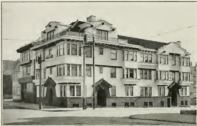
The Lackmann Apartments, San Francisco
