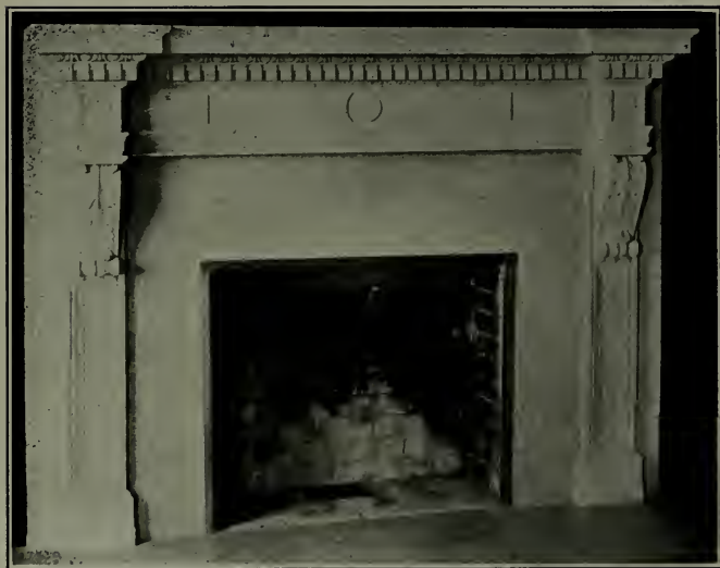
Mantel of Manti Stone and Tavernelle Marble in Home of Attorney Beatty, San Francisco Frederick H. Meyer, Architect
