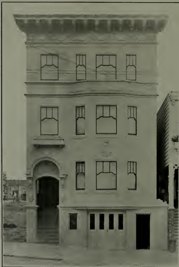
Cement Exterior Residence Flats for Messrs. B. B. and E. R. Golland, San Francisco Milton Lichtenstein, Architect
