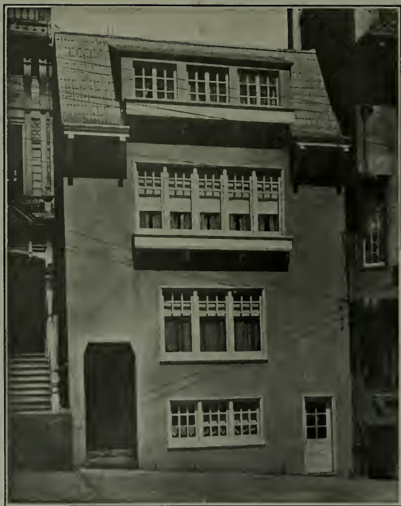
Plats for Mr. Francois Mars, San Francisco, Milton Lichtenstein, Architect Class C Building for Mr. B. H. Lichtenstein, San Francisco
