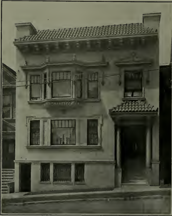
Flats on Cherry Street, near Sacramento, San Francisco Milton Lichtenstein, Architect
