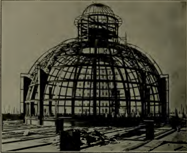
ELLIPTICAL DOME OF KAHN'S DEPARTMENT STORE BUILDING, OAKLAND C. W. DICKEY, Architect
