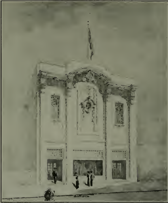
Masonic Temple, Guadalupe, California Welsh & Carey, Architects
