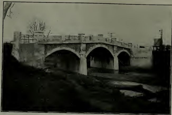
Concrete and Stone Bridge in Santa Clara County J. G. McMillan, Engineer
