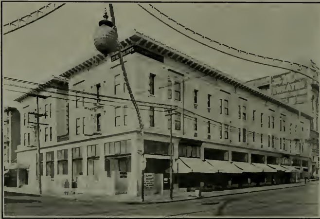
Building at Post and Fillmore Streets, San Francisco. Faced with Sacramento Sandstone Brick Reid Bros., Architects
