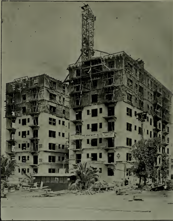
Bryson Apartments Under Construction
