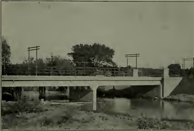
An Attractive Sacramento County Bridge
