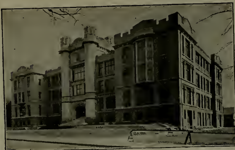
High School, White Plains, New York Basement waterproofed with CERESIT.
