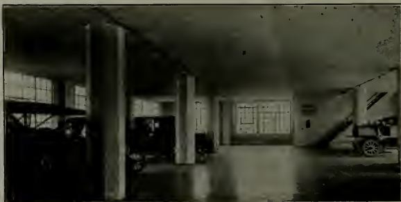
PACKARD SERVICE BUILDING, LOS ANGELES, CAL.
