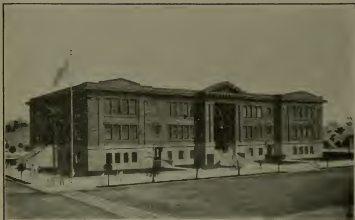
Richmond School Building, Roofed by the Mackenzie Roof Company of Oakland
