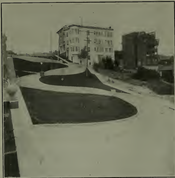
Fig. 1. Concrete Retaining Walls for Terracing Greenwich Street, San Francisco.
