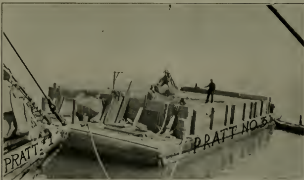
Unloading part of a 5,000 yard (equal to 200 car loads) order of washed gravel with clam shell bucket at Bolinas Bay for the J. G. White Engineering Corporation
