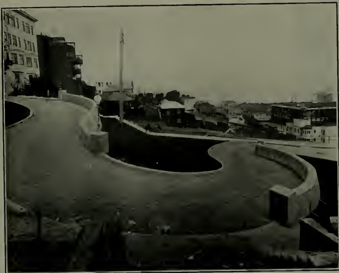
Fig. 2. Showing Sharp but Graceful Curves to Concrete Retaining Walls Greenwich Street, San Francisco
