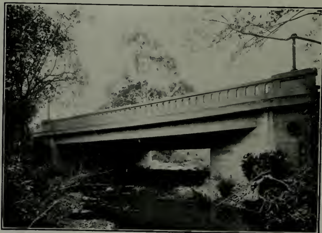
Marsh Street Bridge, San Luis Obispo, California Geo. Story, Engineer
