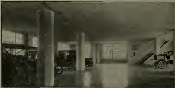
PACKARD SERVICE BUILDING, LOS ANGELES, CAL. Parkinson & Bergstrom, Archts. F. O. Engstrom Co., Contrs. Flat Ceiling of Floredome Construction. Daylighted Throughout with United Steel Sash.
