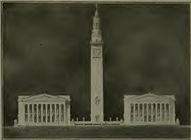
Municipal Group, Springfield, Mass. Tower Equipped With Howard Clock
