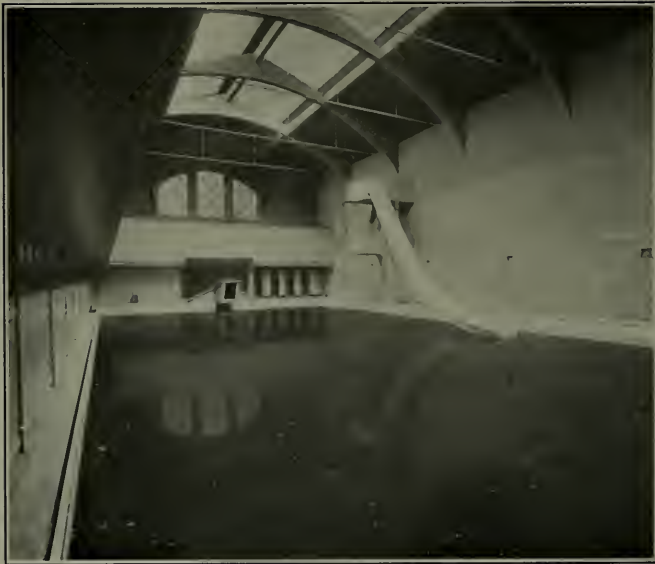
Fig. 5. View of Swimming Pool, Municipal Natatorium, San Jose Note Concrete Slide on the Right
