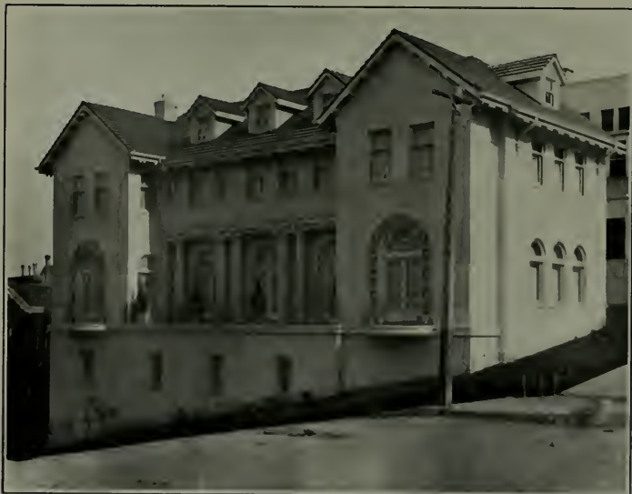
Residence of Mrs. Fred S. Knight, San Francisco Hard & Blohme, Architects
