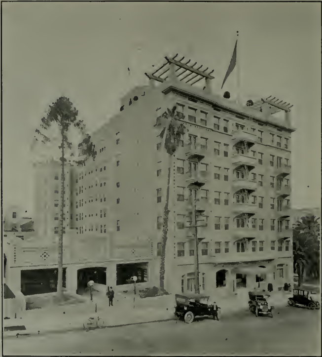
Rex Arms Apartments, Los Angeles, the Most Completely Equipped Apartment House on the Pacific Coast. Note Garage Annex on the Left F. O. Engstrum, Owner. Paul C. Pope, Architect
