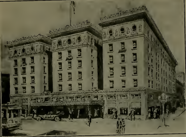
TRAVELERS' HOTEL, SACRAMENTO, CALIFORNIA Washington J. Miller, Architect
