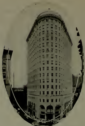
TURK'S HEAD BUILDING Providence, R. I.
