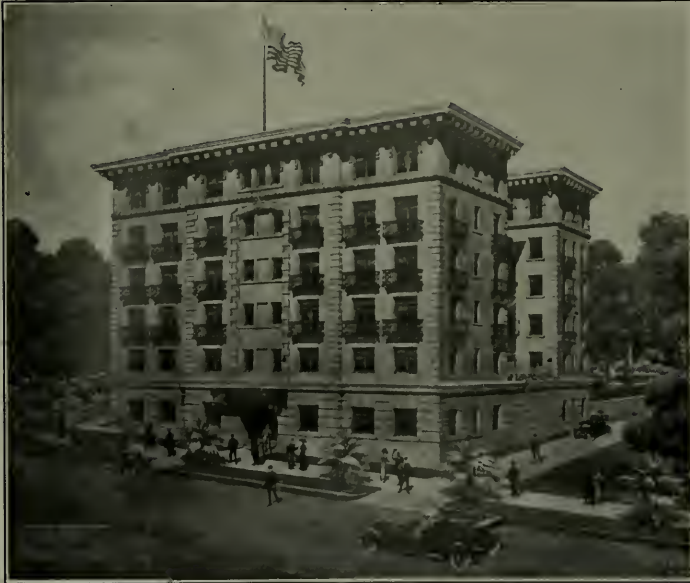
Westonia Apartments, Los Angeles, Fred E. Engstrom, Owner R. B. Young & Sons, Architects
