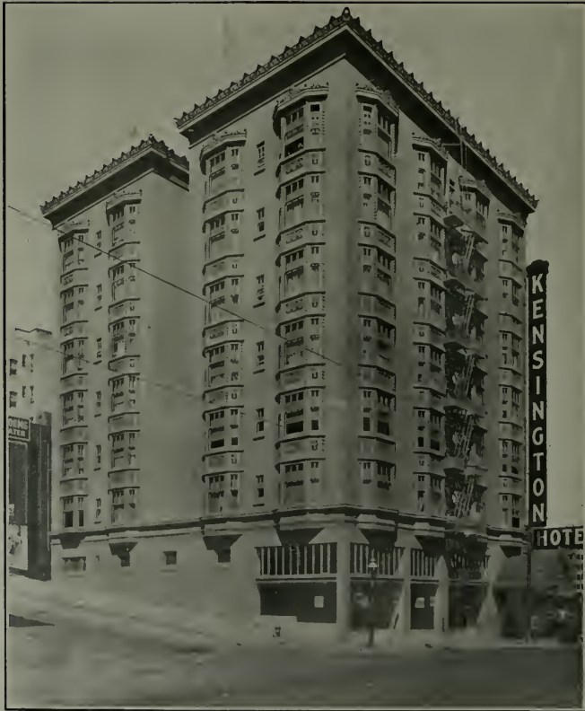
Hotel for S. & G. Gump Realty Company, San Francisco Milton Lichtenstein, Architect
