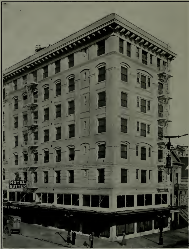
The New Hotel Sutter, Sacramento, California. Faced With Sacramento Sandstone Brick Scadler & Hoen, Architects
