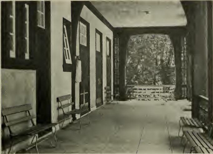
CORRIDOR, JOHN MUIR SCHOOL, BERKELEY
