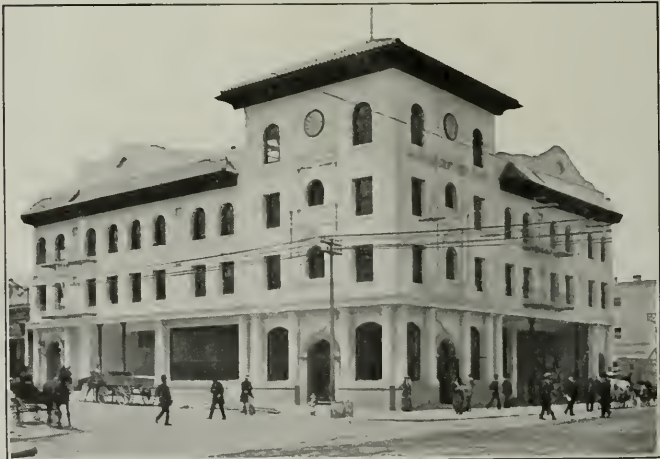
MISSION SAVINGS BANK BUILDING, SAN FRANCISCO Crim & Scott, Architects
