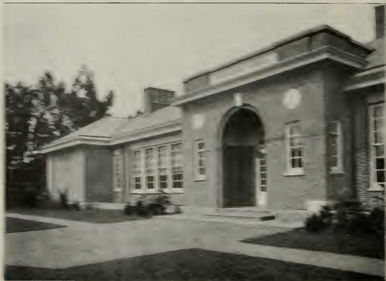
DETAIL OF ENTRANCE, LIVING & DINING ROOMS, 1917-18
