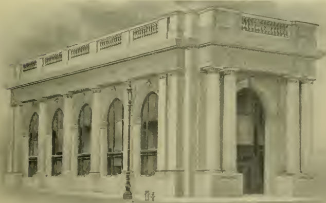
ANGLO AND LONDON PARIS NATIONAL BANK Albert Pissis, Architect
