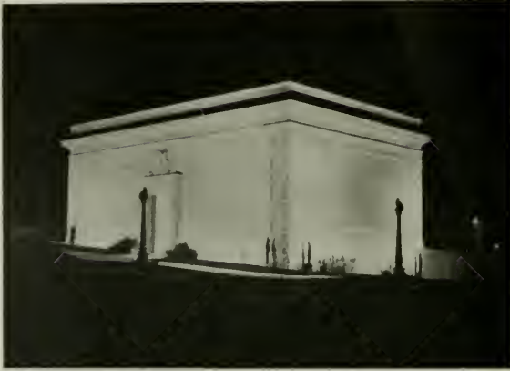
Effect secured when flood lighting is used. By this method of lighting, the finer architectural details are brought out, rather than merely the general outline, as would be the case with outline lighting.
