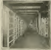
Storage Tanks, San Francisco Warehouse
