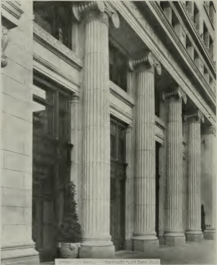
SPRING STREET DETAIL, MERCHANTS NATIONAL BANK, LOS ANGELES W.M. CURLETT & SON, ARCHITECTS
