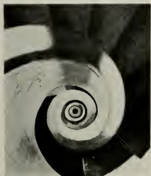
How the "Snail-Shell" Stairway Gets Its Name—Looking Down Four Flights of Uninterrupted Concrete Spiral
