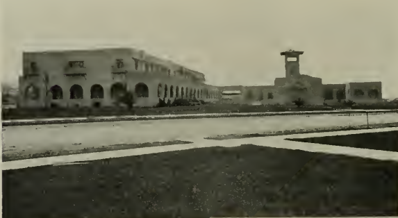
The Irving J. Gill Type of Building, Which the Designer Says Has the True Western Feeling
