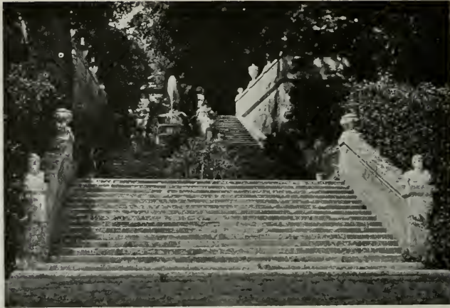
RETAINING WALLS AND ACCESSORIES IN AN ITALIAN GARDEN
