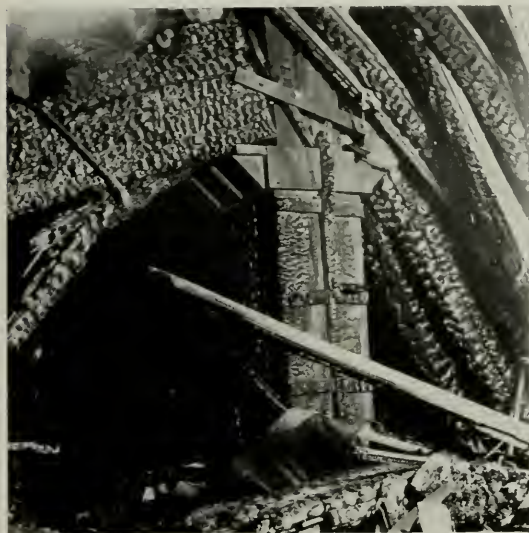
Double Beams and Fire
