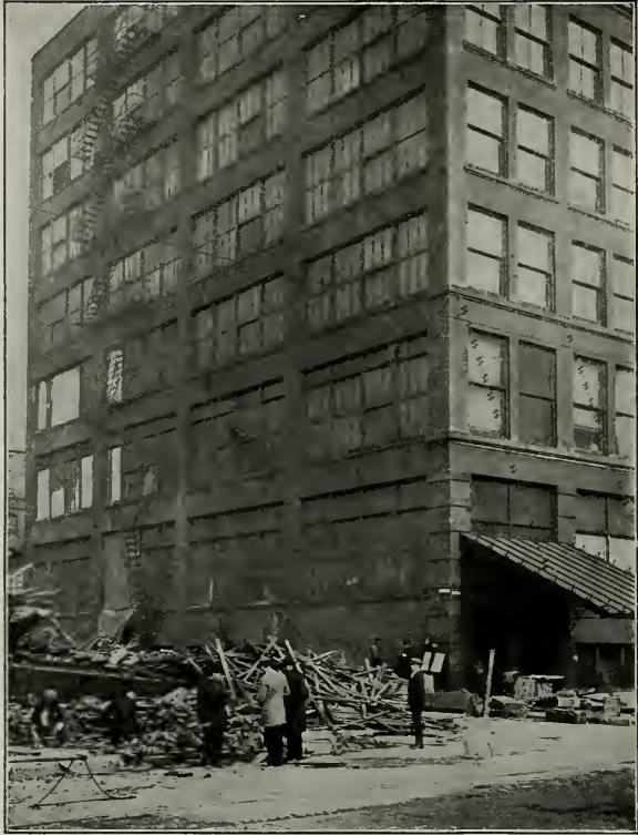
A Successful Fire Stop.—Showing satisfactory fire retardant service of wired glass in metal window frames. Warehouse across twenty-foot alley was totally destroyed. Windows toward rear shown boarded up were broken when side wall of burning building fell.
