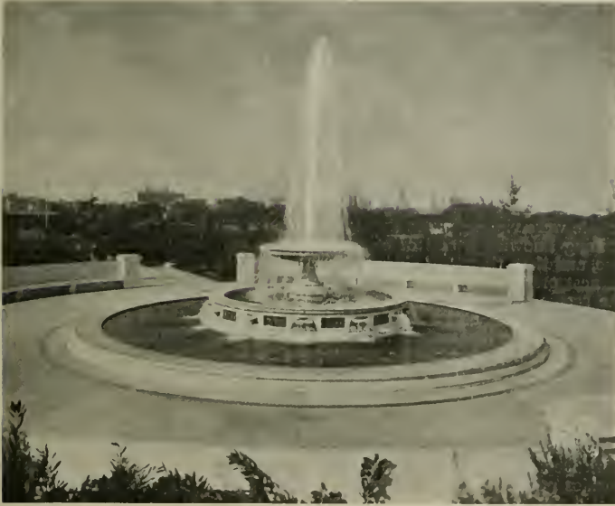
FOUNTAIN, WITH CONCRETE WALK AND SEATS, LAKE MERRITT, OAKLAND Walter D. Reed, Architect
