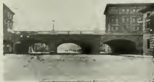
New bridge, replacing former structure, obtained because this city has given its Art Jury power to insist upon decent appearing street improvements.
