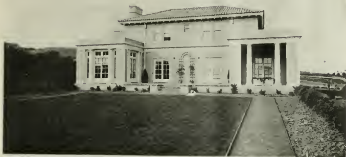
RESIDENCE OF MR. H. T. JAMES, BURLINGAME HILLS Chas. Peter Weeks, Architect
