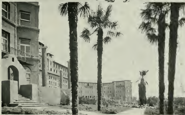
HOTEL HUNTINGTON, OAK KNOLL, PASADENA Additions and Alterations MYRON HUNT, ARCHITECT
