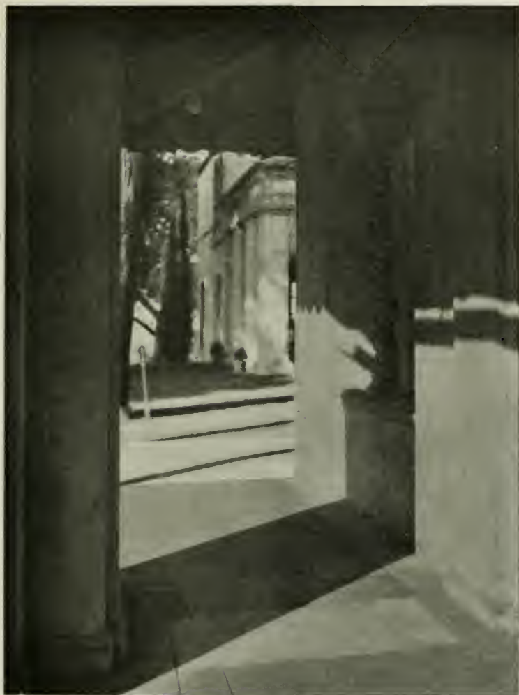
WEST LOGGIA—AN INTIMATE VIEW (NOTE DIVERSITY OF DETAIL), VILLA OF MR. CHARLES D. BLANEY SARATOGA, CALIFORNIA. WILLIS POLK & CO., ARCHITECTS
