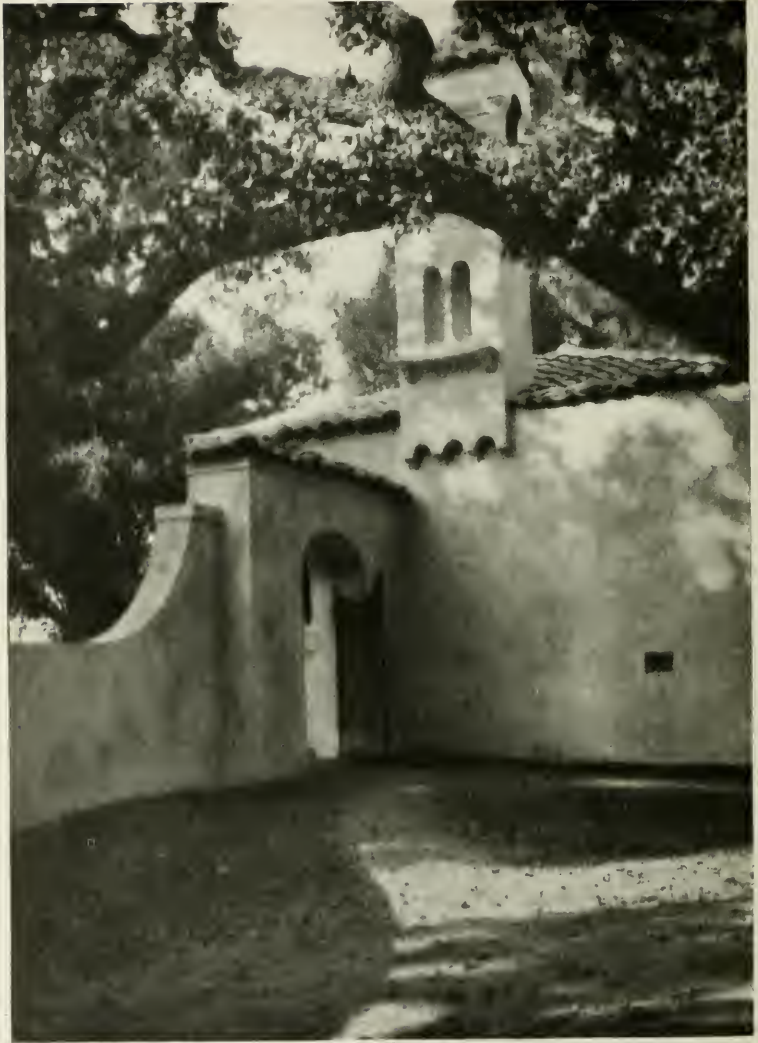
GATEWAY FROM KITCHEN YARD TO WEST GARDEN, VILLA OF MR. CHARLES D. BLANEY, SARATOGA, CALIFORNIA. WILLIS POLK & CO., ARCHITECTS
