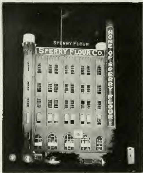
A FACTORY AT STOCKTON, CALIFORNIA
