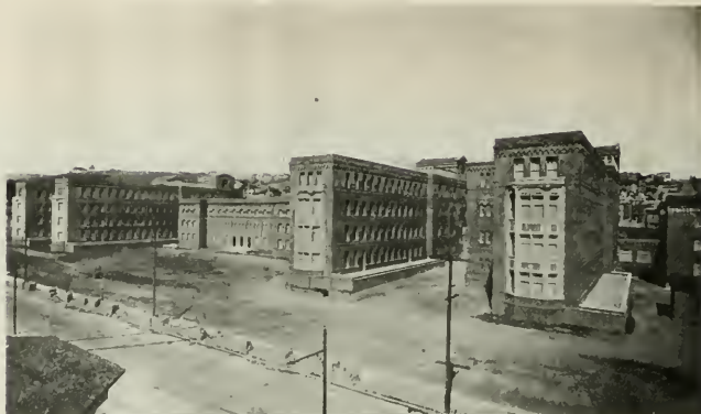
CITY AND COUNTY HOSPITAL, SAN FRANCISCO Constructed entirely of red pressed brick
