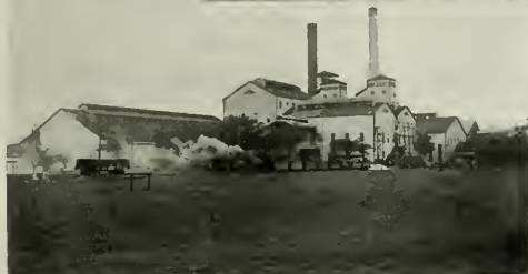
OAHU SUGAR COMPANY'S MILL BUILDINGS WAIKAPU, T. H. HAWAIIAN ISLANDS Armco Iron Corrugated roofing and siding.
