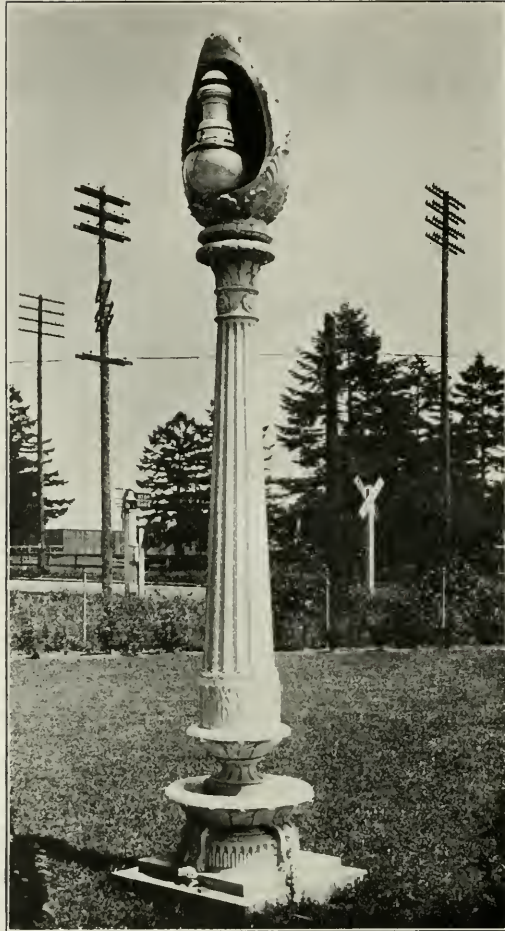
CONCRETE ELECTRIC FLOOD LIGHTING POST
