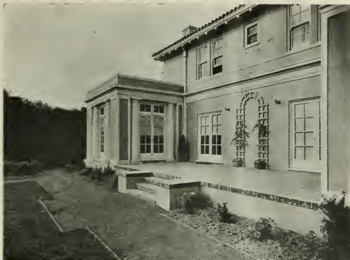
RESIDENCE OF MR. H. T. JAMES, BURLINGAME HILLS Chas. Peter Weeks, Architect
