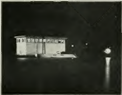
THE HALSEY POWER HOUSE
