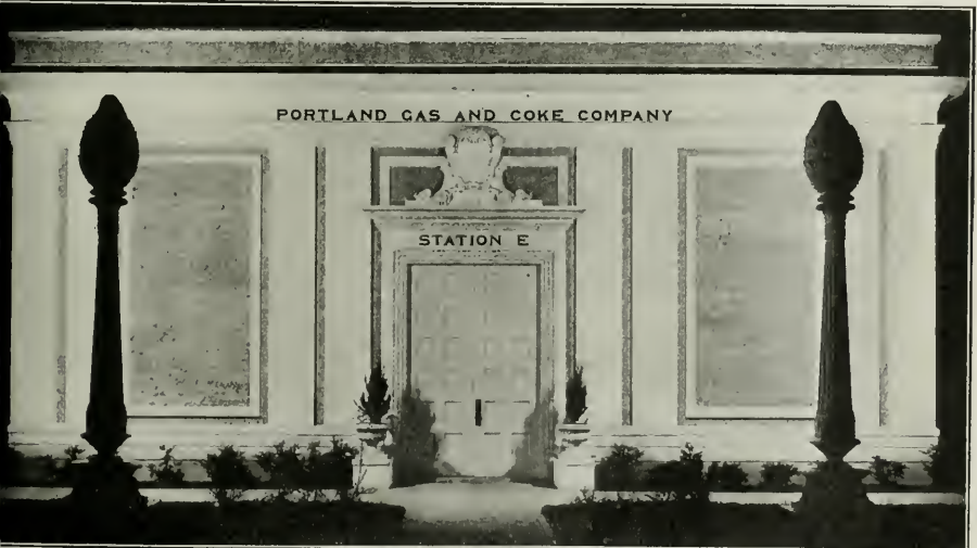
NIGHT VIEW, STATION E, PORTLAND GAS & COKE COMPANY, PORTLAND, OREGON
