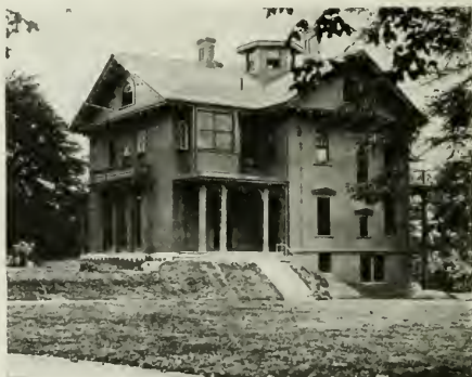
Fig. 4. The Charlex Choate Memorial Hospital as produced by the first modification of the Choate homestead.
