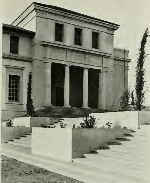
ENTRANCE DETAIL. FOWLER HALL, OCCIDENTAL COLLEGE, LOS ANGELES Myron Hunt, Architect
