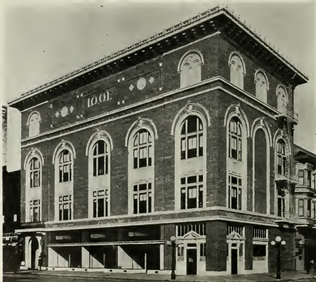
I. O. O. F. BUILDING, OAKLAND J. Henry Boehrer, Architect
