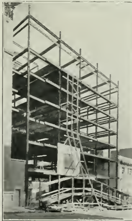
STEEL FRAME Y. W. C. A. BUILDING, SAN FRANCISCO
