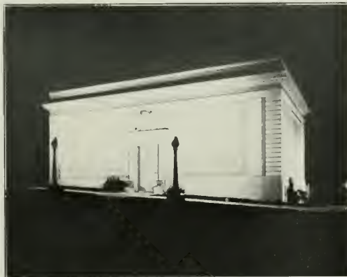
A CITY SUBSTATION
