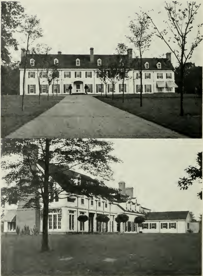
RESIDENCE OF MRS. GRAHAM BABCOCK, TEXAFLY, N. J. MYRON HUNT, ARCHITECT
