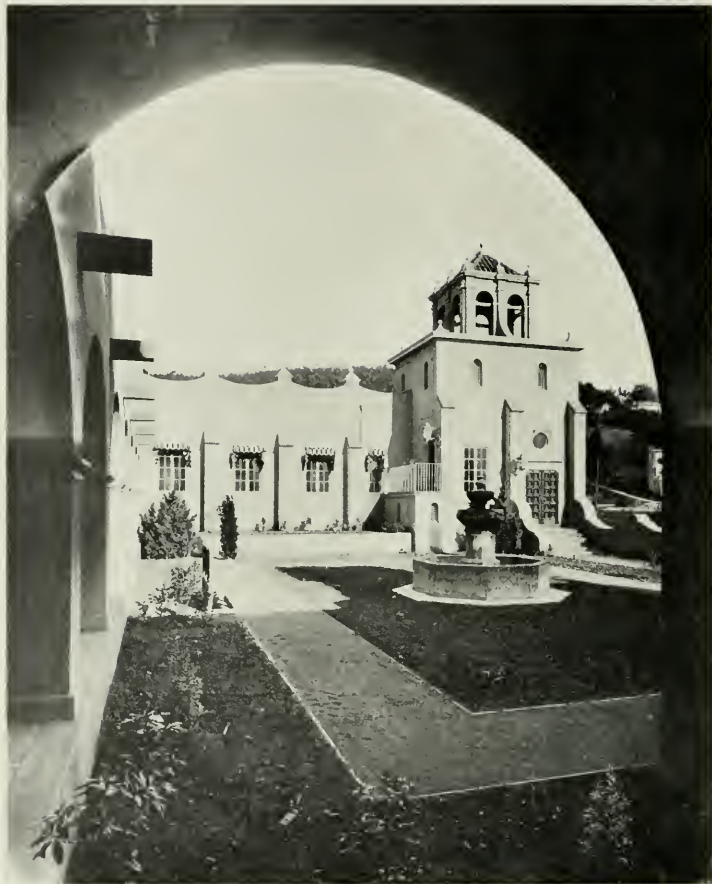
PATIO LOOKING TOWARDS THE OPEN AIR STAGE, PIEDMONT CHURCH ALBERT FARR, ARCHITECT
