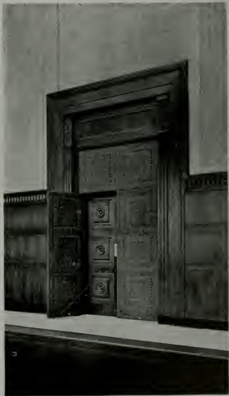
ENTRANCE DOOR TO SUPERVISORS' CHAMBER
