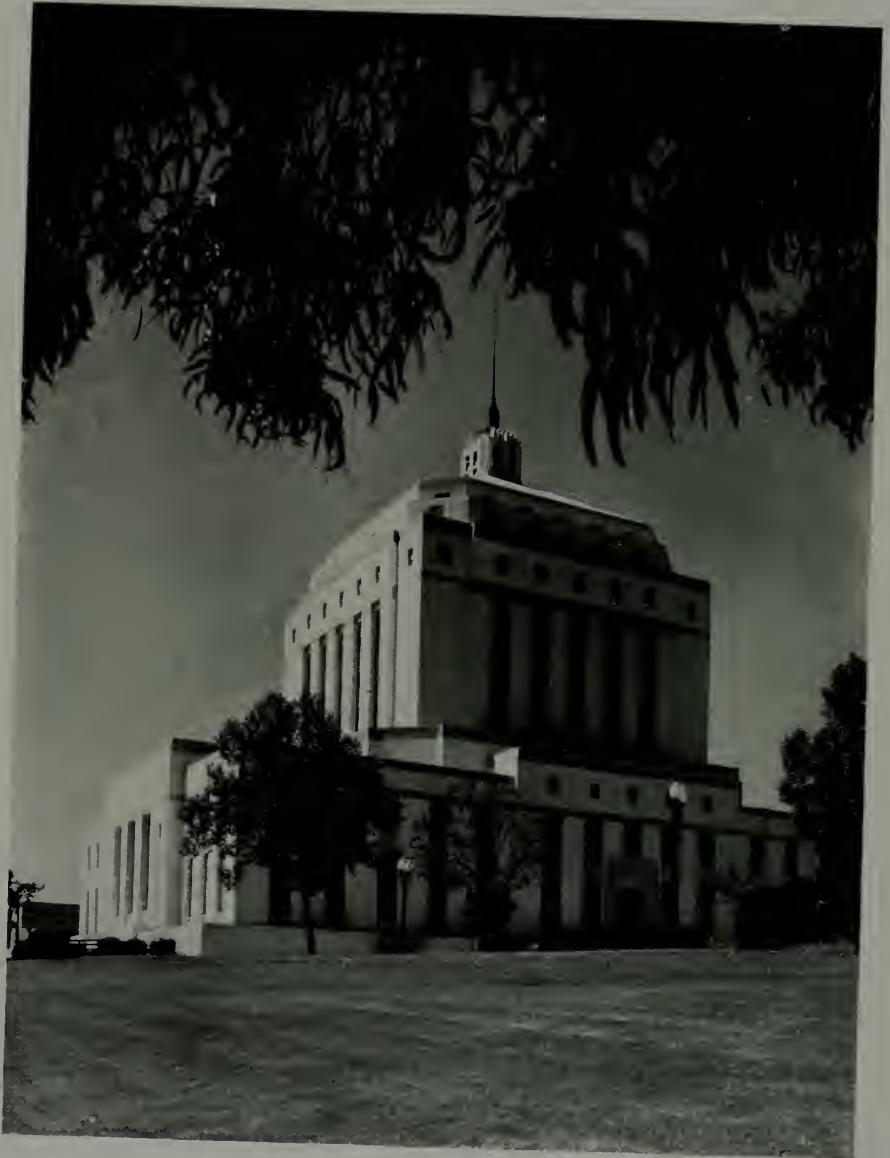
GEORGE WAGNER AND K. E. PARKER COMPANY, GENERAL CONTRACTORS COURT HOUSE AND HALL OF RECORDS, OAKLAND, CALIFORNIA W. G. CORLETT, J. W. PLACHEK, H. A. MINTON, W. E. SCHIRMER AND CARL WERNER, ARCHITECTS
