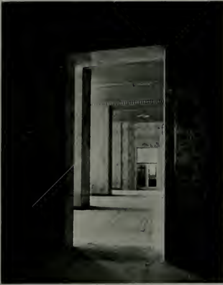
MAIN ENTRANCE LOBBY FROM SUPERVISORS' STAIRWAY
