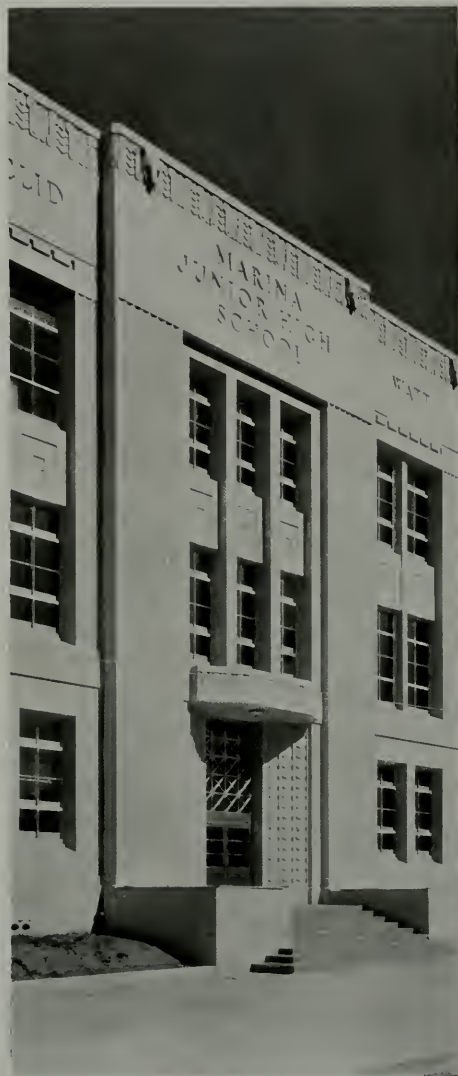
DETAIL, MARINA JUNIOR HIGH SCHOOL, SAN FRANCISCO Geo. W. Kelham and W. P. Day, Architects
