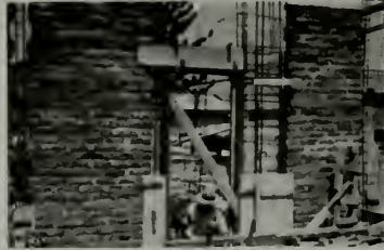
BUILDING WITH BRICK AND HOLLOW TILE IN SAN SALVADOR
