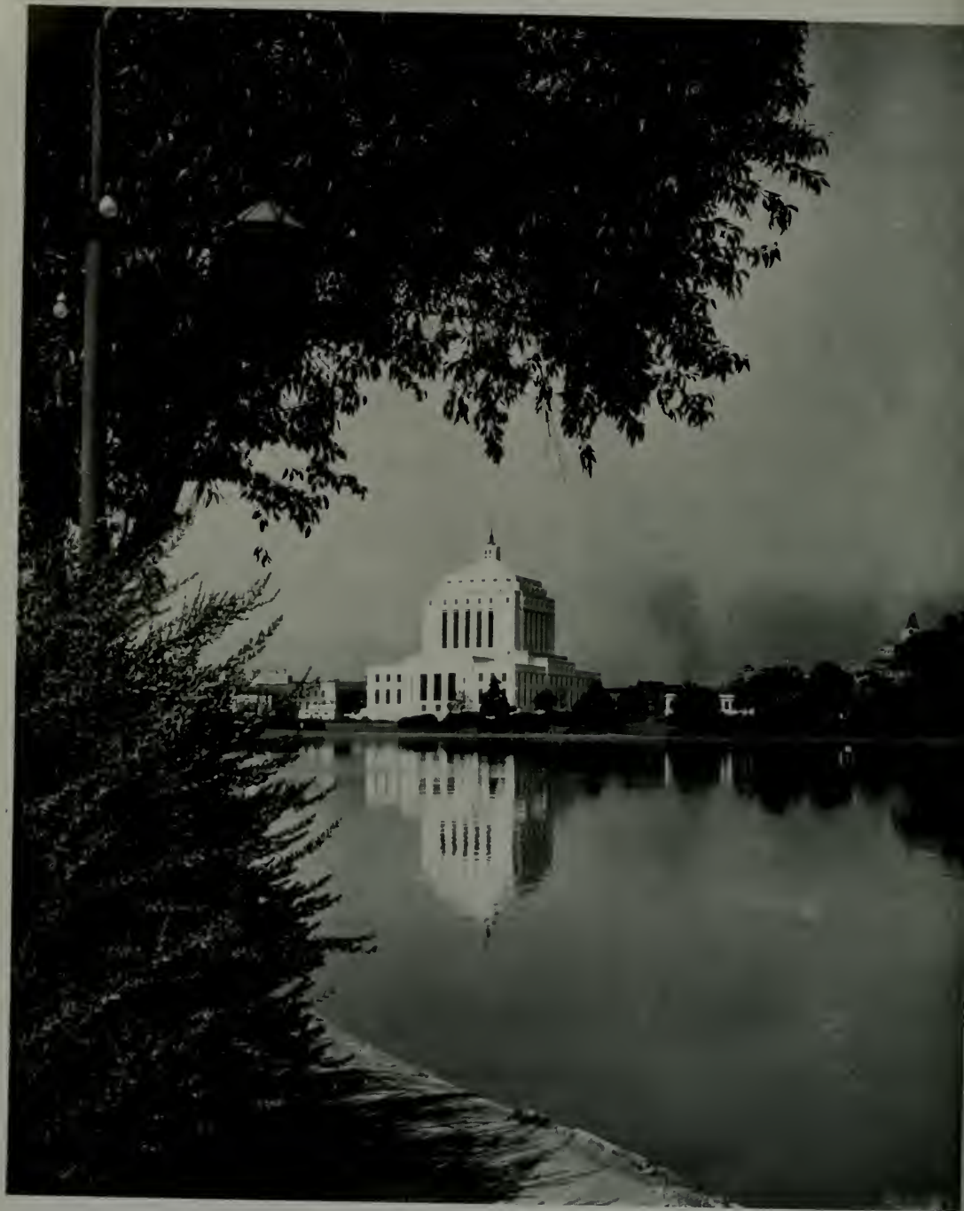
COURT HOUSE AND HALL OF RECORDS, OAKLAND, CALIFORNIA, LOOKING ACROSS LAKE MERRITT
