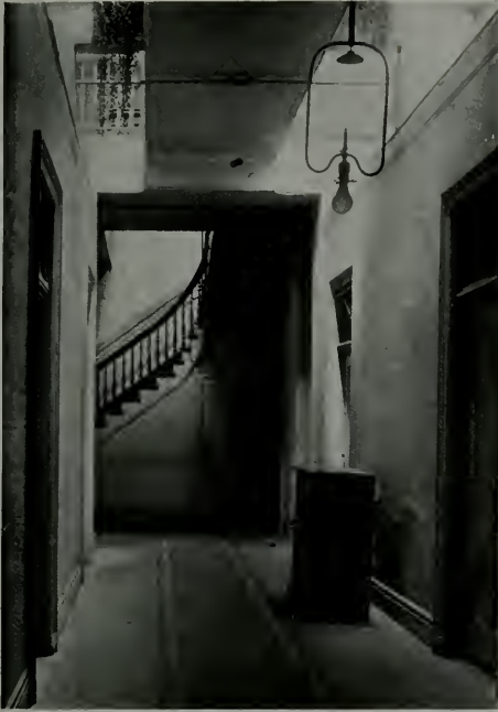
CORRIDOR OF SECOND FLOOR OFFICES, VICTORY BUILDING, SAN JOSE, BEFORE ALTERATIONS.
