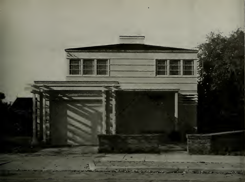
FRONT ELEVATION, HOUSE FOR MR. OTIS R. MARSTON, BERKELEY Eldridge T. Spencer, Architect
