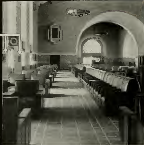
The architects for the Union Passenger Terminal, Los Angeles, have protected the Johnson room thermostats, in the main waiting room, by designing special protective housings, so that there will be no interference with their important functions.
