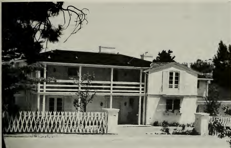
PARTIAL FRONT ELEVATION, HOUSE FOR MR. AND MRS. ROY C. POWERS, HILLSBOROUGH, CALIFORNIA
