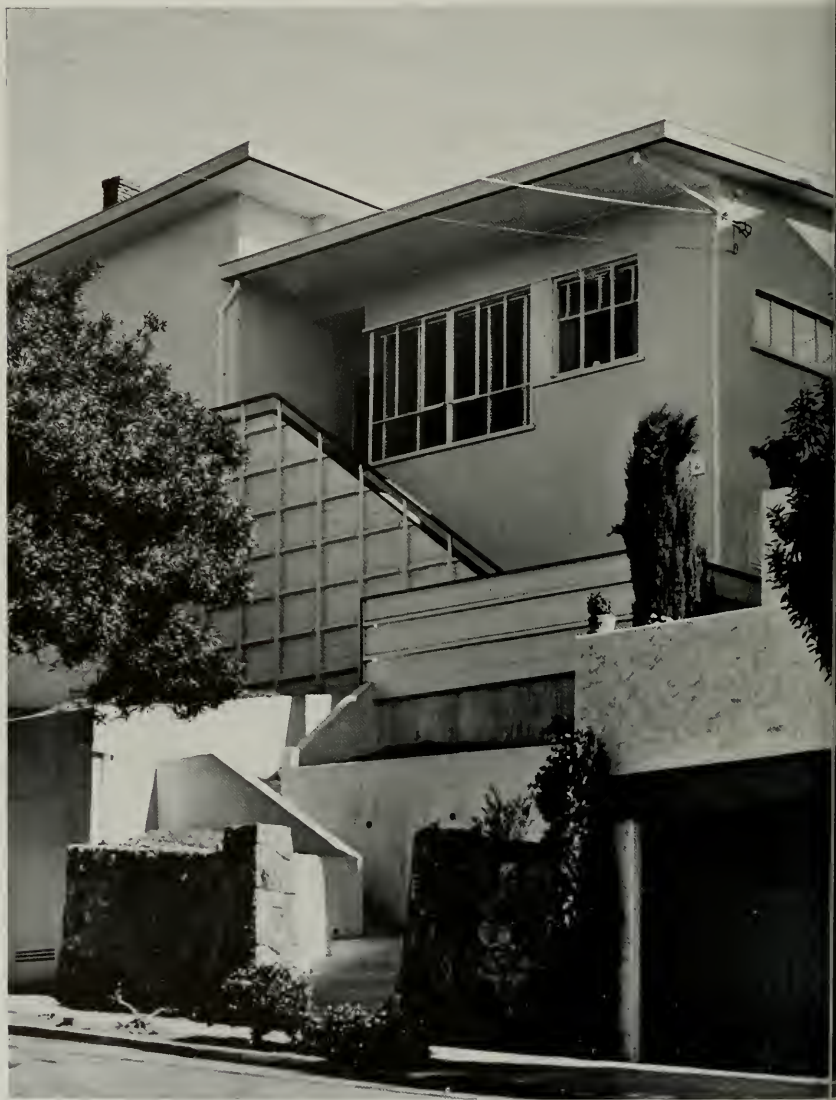
HILLSIDE APPROACH FROM STREET
