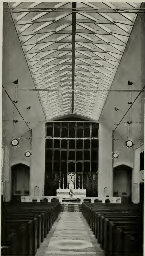
ALL SOULS CHURCH, ALHAMBRA, CALIFORNIA HENRY CARLTON NEWTON, ARCHITECT, J. EARL TRUDEAU, ASSOCIATE R. HOWARD ANNIN, STRUCTURAL ENGINEER
