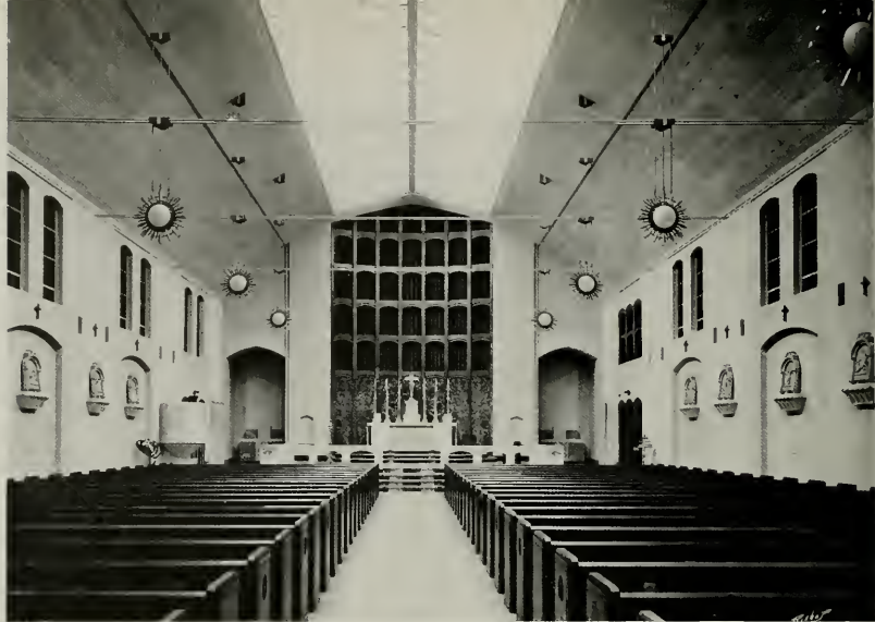
Lighting Fixtures by Wagner-Woodruff
