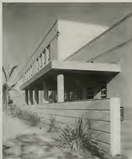
ENTRANCE DETAIL, SANTA MONICA BOULEVARD SCHOOL, LOS ANGELES LEFT—DETAIL
