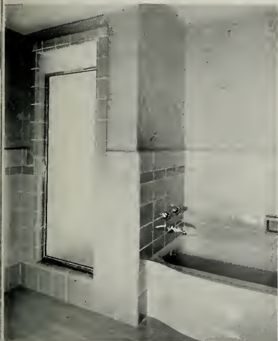
FULLY TILED STALL SHOWER AND RECESS BATHTUB
