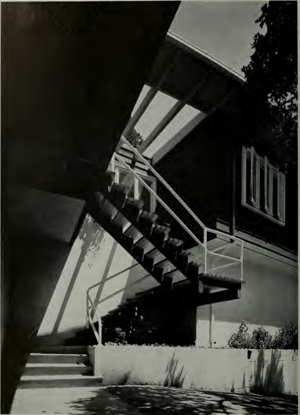
RESIDENCE OF CHARLES BAKER, SLEEPY HOLLOW ACRES, FAIRFAX, CALIFORNIA FRANCIS E. LLOYD, ARCHITECT
