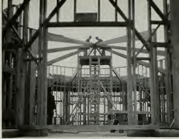
PLACING LAMINATED WOOD ARCH RIBS, PENTHOUSE THEATER, UNIVERSITY OF WASHINGTON, SEATTLE.
