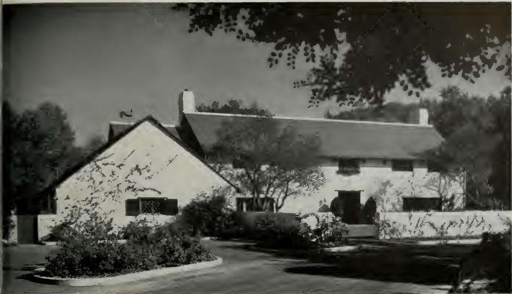
GENERAL VIEW OF GEORGE MILLER RESIDENCE, BEL-AIR, CALIFORNIA
