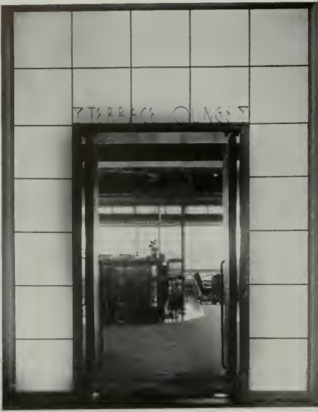
DETAIL OF ENTRANCE TO BAR AND TERRACE LOUNGE, HOTEL CLAREMONT, BERKELEY, CALIFORNIA FREDERICK L. CONFER, ARCHITECT
