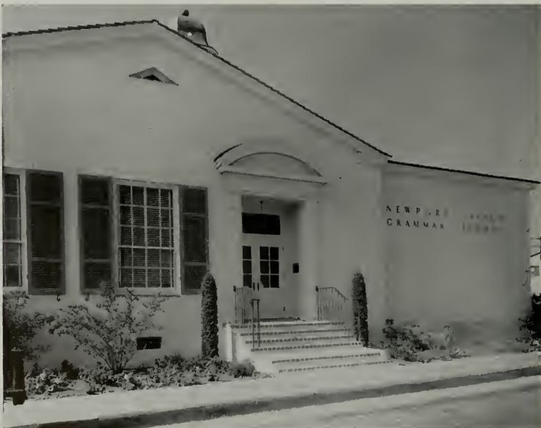
DETAIL OF ENTRANCE
