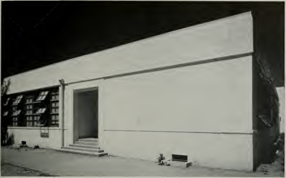
STREET ENTRANCE TO CLASS ROOM UNIT, DEER VALLEY UNION SCHOOL, BRENTWOOD, CALIFORNIA
