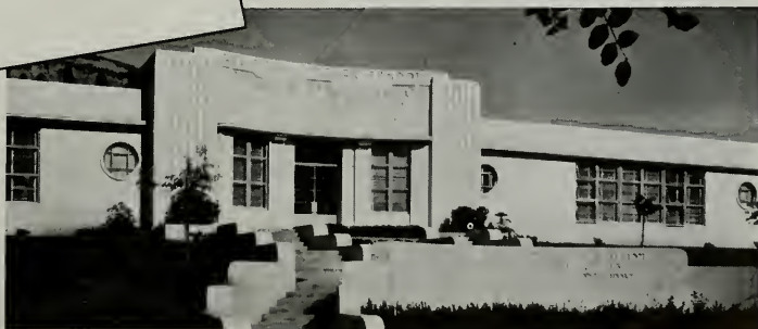
Wm. H. Harrison, architect, designed these two interesting concrete schools. Paul E. Jeffers, structural engineer. Whittier Union High School Auditorium (above) built by J. K. Thomas. Lou Henry Hoover School (right) by J. & B. Construction Co.
