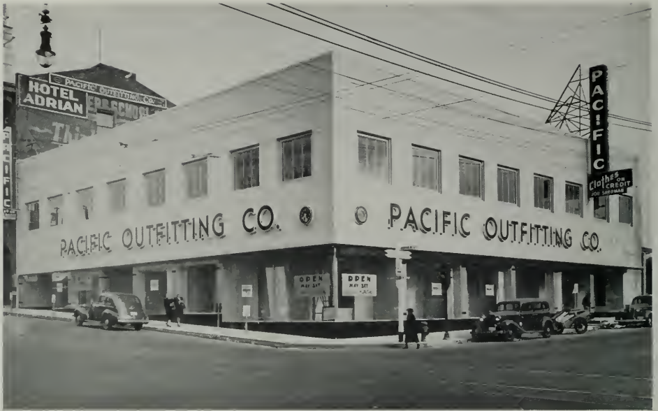
ALTERATIONS, PACIFIC OUTFITTING CO. BUILDING, PORTLAND, OREGON Bernard Heims & L. L. Dougan, Associate Architects
