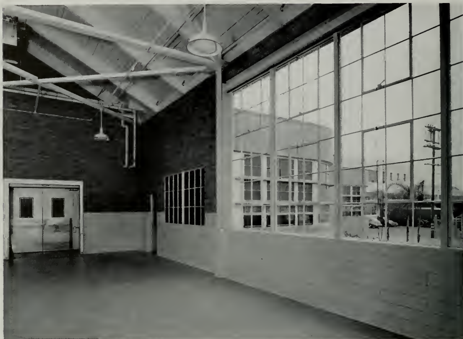
INTERIOR OF PAPER MILK-CONTAINER PLANT OF AMERICAN CAN COMPANY, LOS ANGELES
