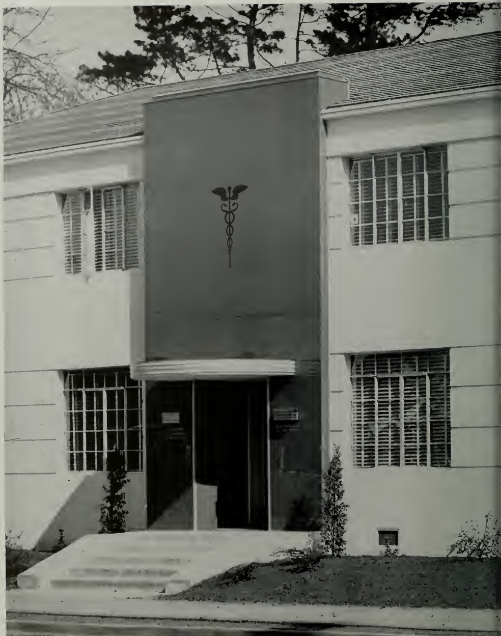
ENTRANCE DETAIL, MEDICO-DENTAL BUILDING FOR DR. R. E. HAMLIN, SANTA ROSA, CALIFORNIA
