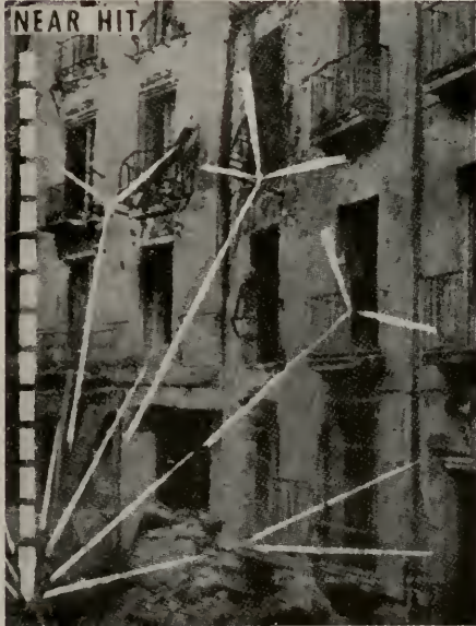
Contact burst on street exerted no earth shock but fragments riddled walls.
