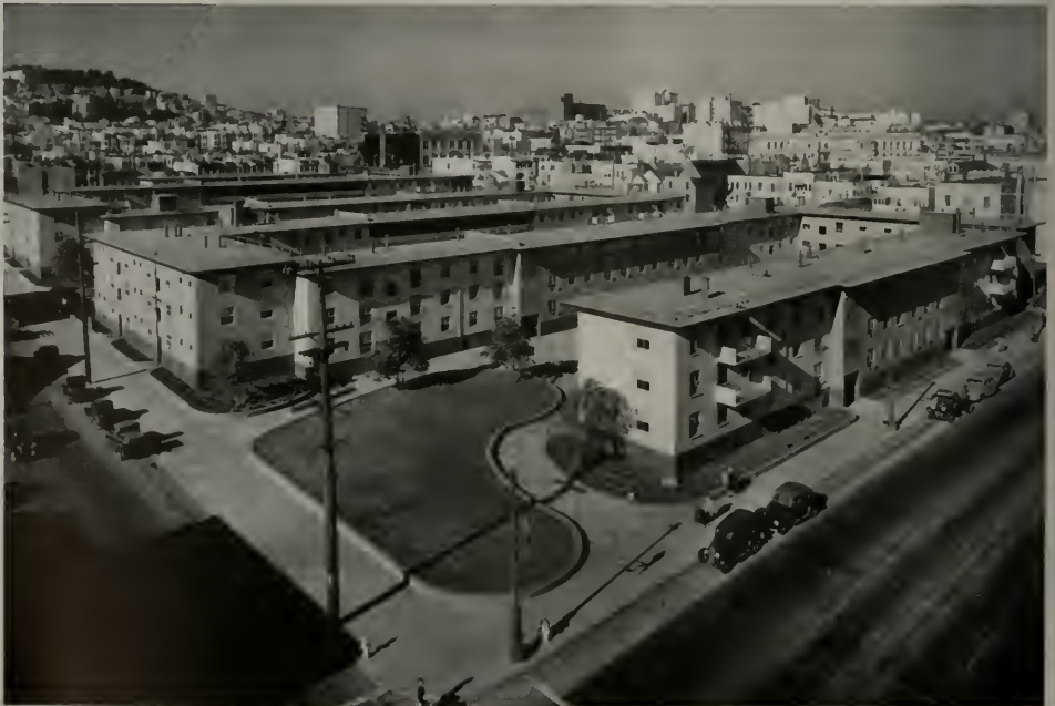
VALENCIA AND FIFTEENTH STREETS, SHOWING LANDSCAPING AND ARRANGEMENT OF COURTS
