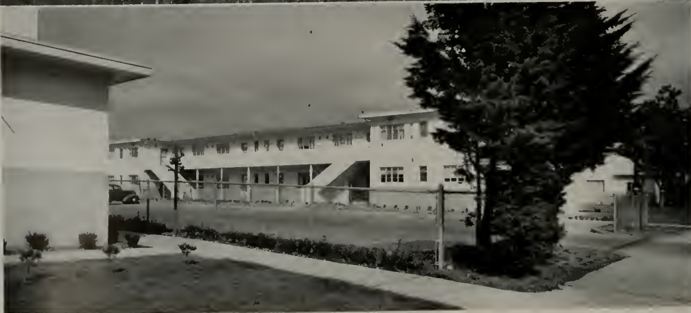
THREE VIEWS OF PERALTA PROJECT SHOWING FLAT BUILDINGS IN LOWER PICTURE NOTE OUTSIDE BALCONY FOR ENTRANCE TO SECOND STORY FLATS
