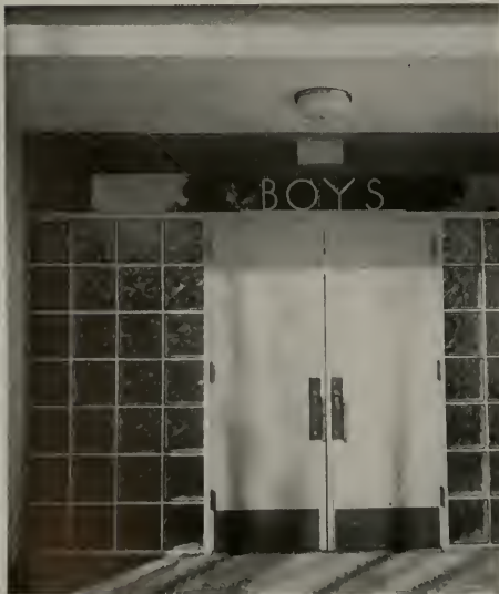
ENTRANCE TO BOYS' LOCKER AND SHOWER ROOM
