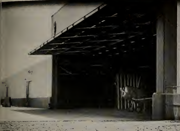
MODERN APPEARANCE Steel panels offer a wide variety of designs... fluted, corrugated or V-crimped. With proper insulation, they offer good protection against heat or cold.
