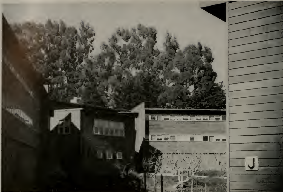
SAUSALITO: Dormitory of permanent construction. (Note fire-wall separating wing from utilities section.)
