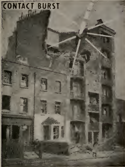
With fuse set for contact, bomb exploded the instant it penetrated roof.
