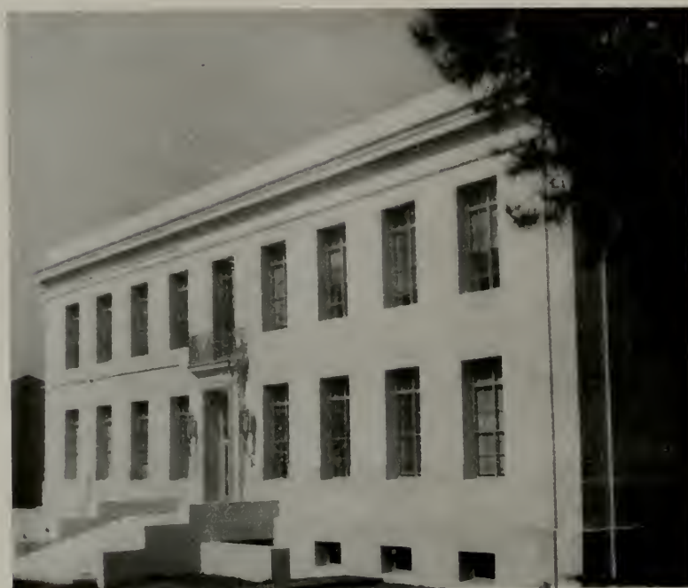
Upper—BARROWS STREET FRONT. Lower—BANCROFT AVENUE
