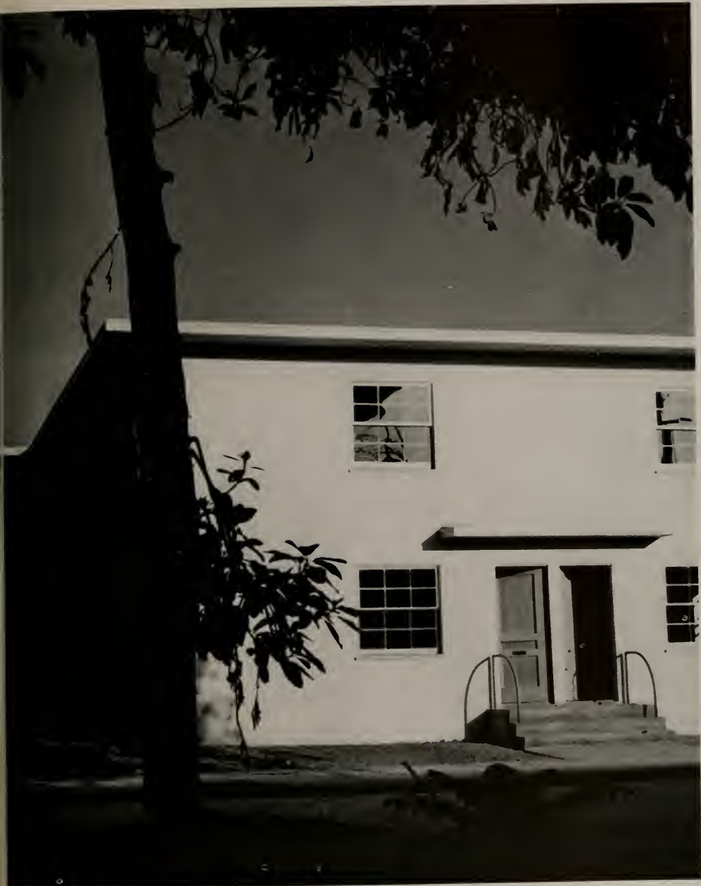
TYPICAL ENTRANCE TO TWO STORY APARTMENTS. THERE ARE ELEVEN OF THESE BUILDINGS, EACH CONTAINING 14 APARTMENTS. CONSTRUCTION IS FRAME AND STUCCO WITH REINFORCED CONCRETE GROUND FLOORS
