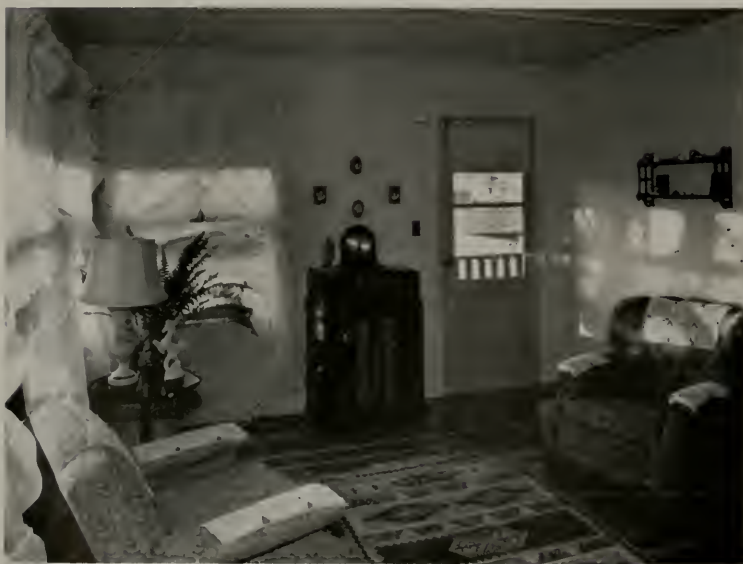
Each wall was factory-built as a unit, complete with windows, doors, electric fixtures, interior and exterior finishes. Floor sections were delivered with underpinnings, ceiling sections with roof sheathing.
