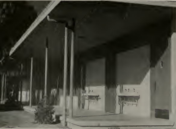
Above: Exterior corridor detail. Note continuous corridor windows.
