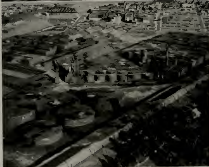
Here, disruptive painting with low-visibility, infrared resistant camouflage paints has altered the scene. A simple train shed effect can be accomplished with painted chicken wire stretched over framework.
