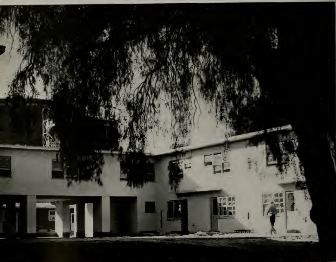
"H" Type Apartments. Note Ramada Type of Construction (Open Passages Connecting Wings on Either Side of Court) Second Story Rests on Transverse Beams Supported by Piers
