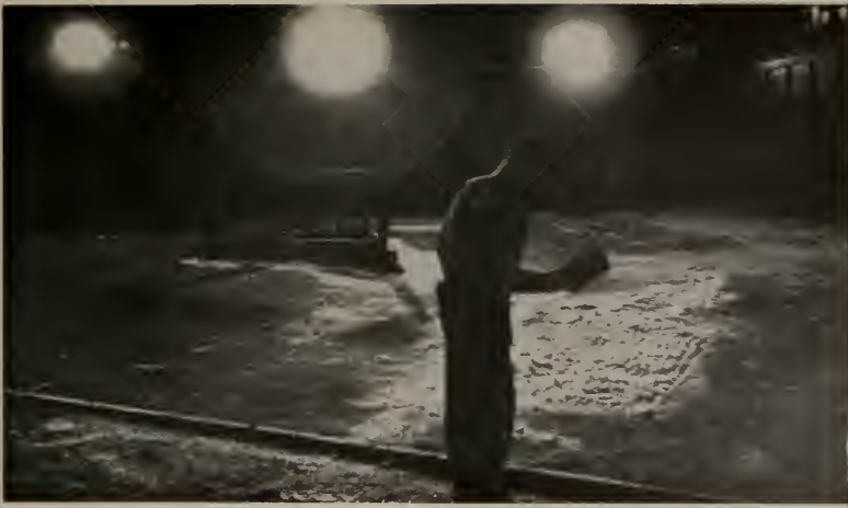
A saboteur, attempting to enter a correctly lighted industrial property, is blinded by the direct beams of the protective lighting system.
