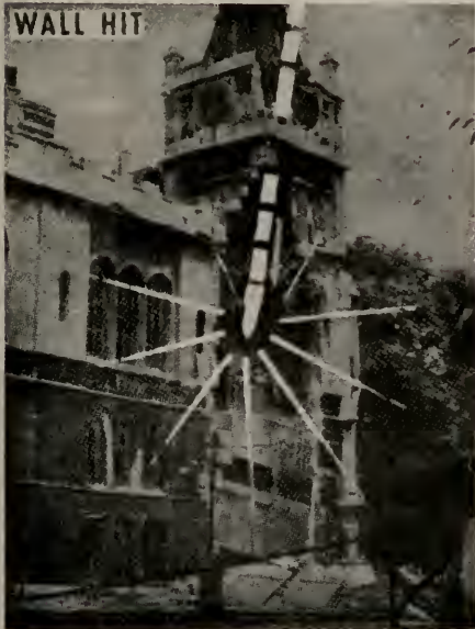
Bomb, in curving flight, went through side wall and blew up on third floor.
