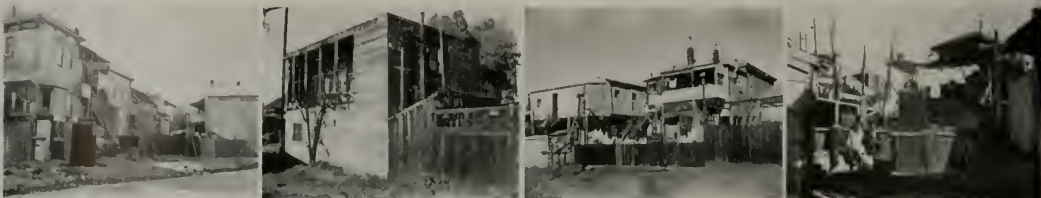
These views show sub-standard housing conditions before the Peralta and Campbell projects were started. Congestion, insanitation and fire menace are apparent in all four pictures.
