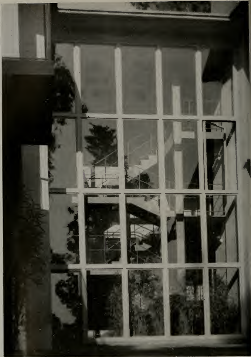
GLASS-ENCLOSED STAIRWAY, STERN HALL, NEW GIRLS' DORMITORY, UNIVERSITY OF CALIFORNIA, BERKELEY CORBETT & MacMURRAY AND W. W. WURSTER, ARCHITECTS, ASSOCIATED
