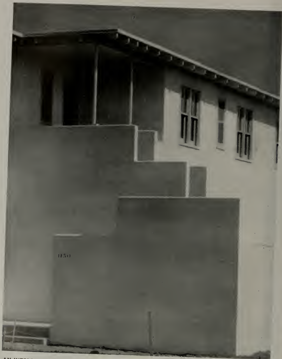
AN INTERESTING DETAIL, LOCKWOOD GARDENS LOW RENT HOUSING PROJECT, OAKLAND, CALIFORNIA
