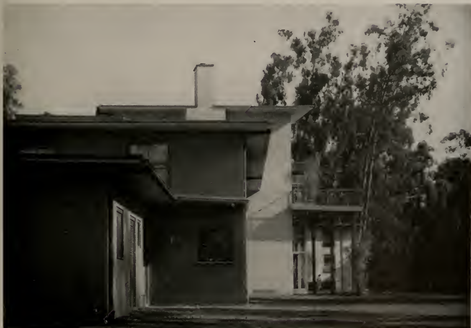
SERVICE WING AT HEARST STREET END OF DORMITORY
