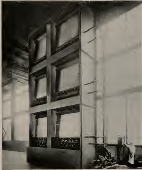
One of the exhaust units in the fabricating shop, prior to installation
