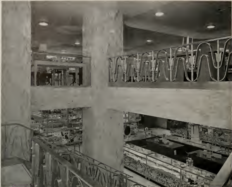
MEZZANINE FLOOR of straight grain bleached oak, lacquered and mirrored. Ample lighting from spacious stairway and indirect, subdued lighting fixtures. Designed for Gift Shop and Beauty Salon.
