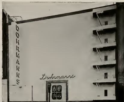
DOHRMANN'S Union Square San Francisco, Calif. Albert R. Williams and Associates Architects
