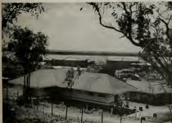
Administrative Offices and oil tanks
