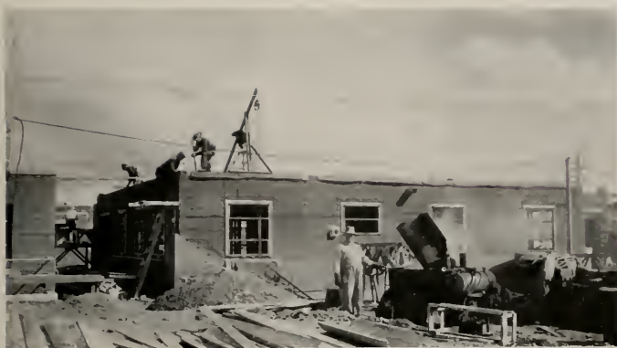
One of Medical Buildings Under Constructions
