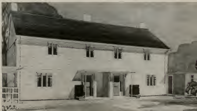
THE AIREY HOUSE. Of pre-cast concrete construction, this is one of the new types of houses designed by the British Iron and Steel Federation suitable for rural areas in groups of 50 or more.
