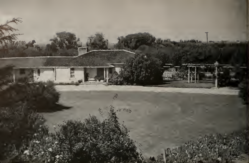
View from Sacramento River Bank
