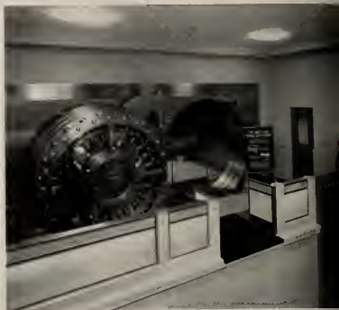
Giant modern Vault Door in the safe deposit department of the new Anglo California National Bank in Oakland. The door is 22 inches thick, 9 feet in diameter, and weighs 70,000 pounds.
