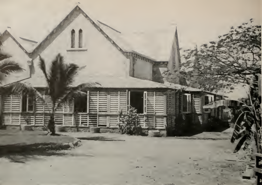
Above: The Residency, Official Home of the Administrator
