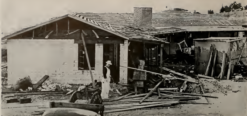
HOME BEING CONSTRUCTED AT SAN JOSE, CALIFORNIA
