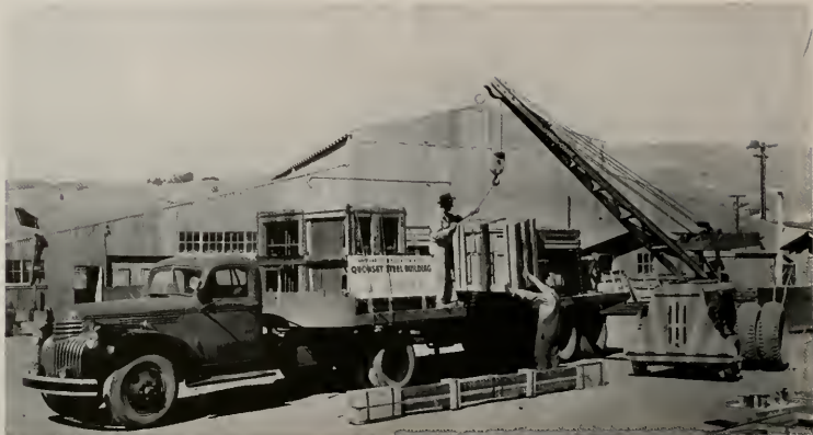
DESTINED FOR ARABIA, these export-packaged Stran-Steel "Quonset" buildings start the long journey from Kraftfile Company's Niles, California, warehouse. "Quonsets" totaling more than 100,000 square feet of floor space have been purchased for use in Arabian construction operation. (Kraftfile Co. Photo)
