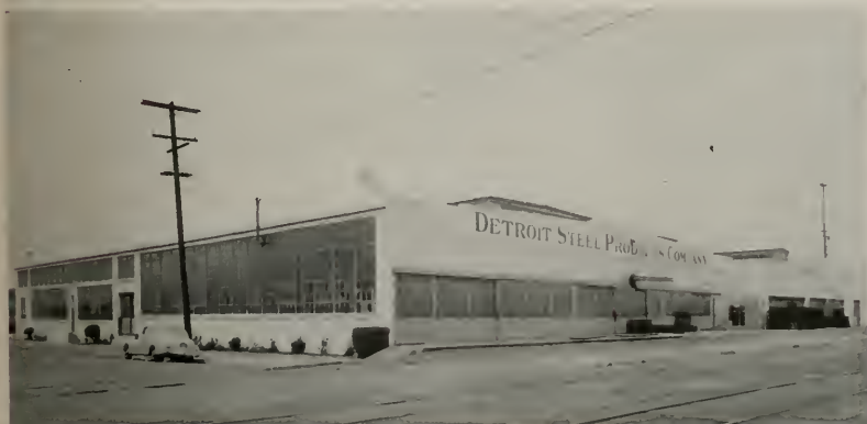
Emeryville, California, Plant prior to Remodeling
