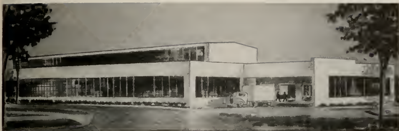
Newly Completed Addition to Emeryville Plant
