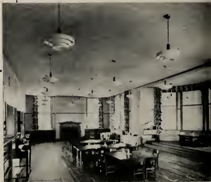
Ultra-modern kindergarten, Meeker Grade School, Puyallup, Washington, showing Simpson Acoustical Tile installation. Similar installations were also made in all other classrooms and corridors in the new school addition.
