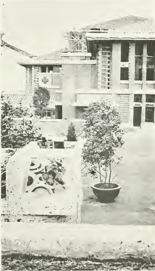
On the roof of the center unit, viewing the rear superstructure, containing the banquet hall and the theater
