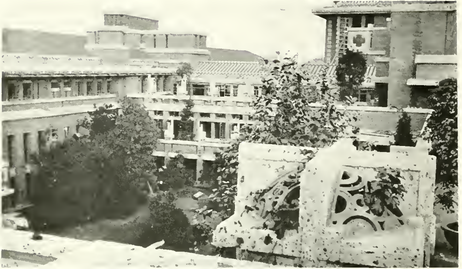
An inner court between the left wing and the center unit; the manifestations of this court are repeated between the center units and the right wing
