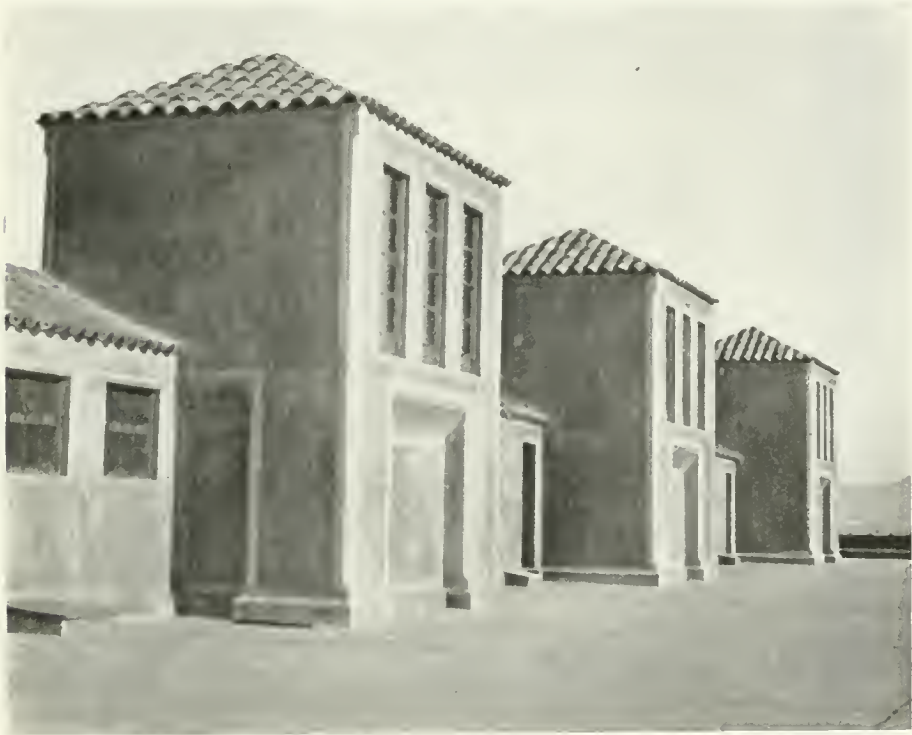
ROOF HOUSES, BUILDING FOR THEO. H. DAVIES & CO., LTD., HONOLULU, T. H. Louis Christian Mullgardt, Architect
