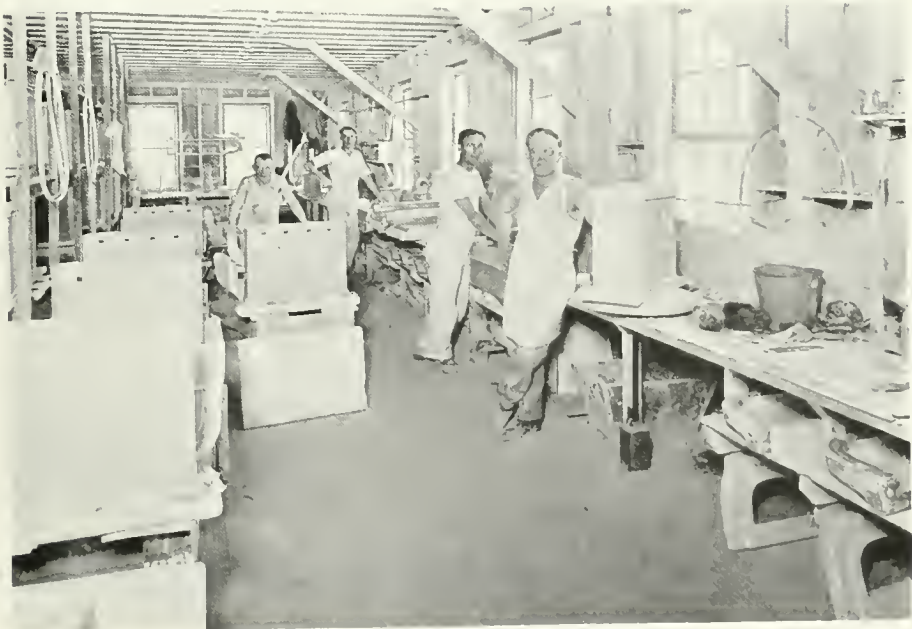
Pressing shops. Toilet tanks assembled.
