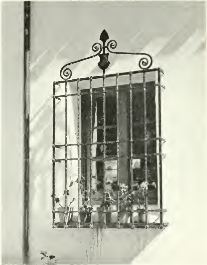
WROUGHT IRON GRILLE, HOUSE OF MR. GEORGE WASHINGTON SMITH, SANTA BARBARA, CALIF. George Washington Smith, Architect
