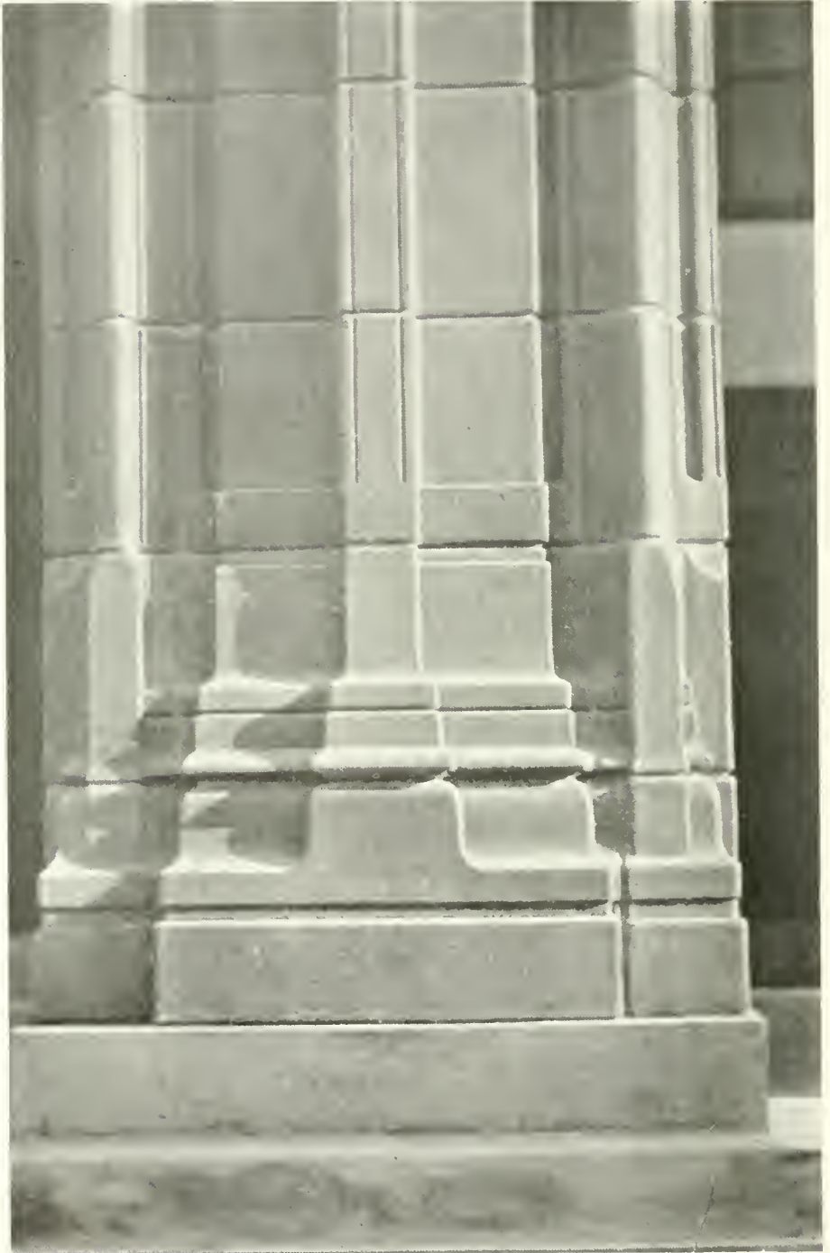
BASE OF ARCADE PIER, BUILDING FOR THEO H. DAVIES & CO., LTD., HONOLULU, T. H. LOUIS CHRISTIAN MULLGARDT, ARCHITECT Terra Cotta manufactured and erected by Gladding, McBean & Co., San Francisco.
