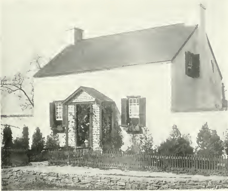
SMOOTH TEXTURE APPROPRIATE FOR A SMALL HOUSE Milton Dana Morrill, Architect
