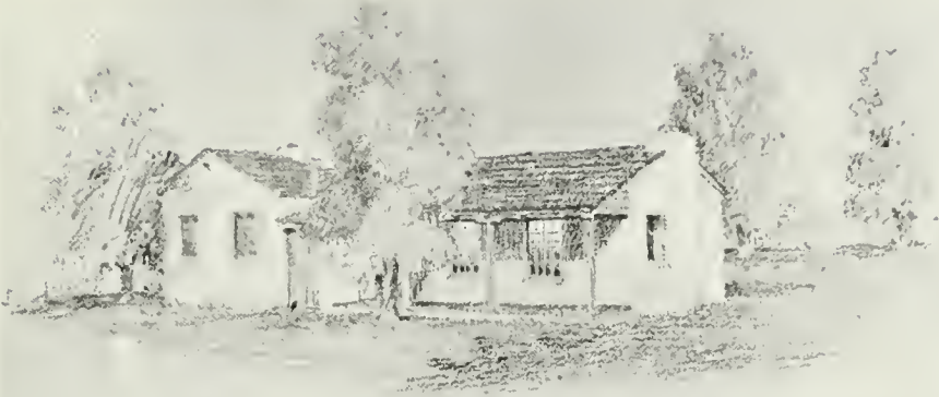
HOUSE FROM SOUTH, SHOWING ENTRY
