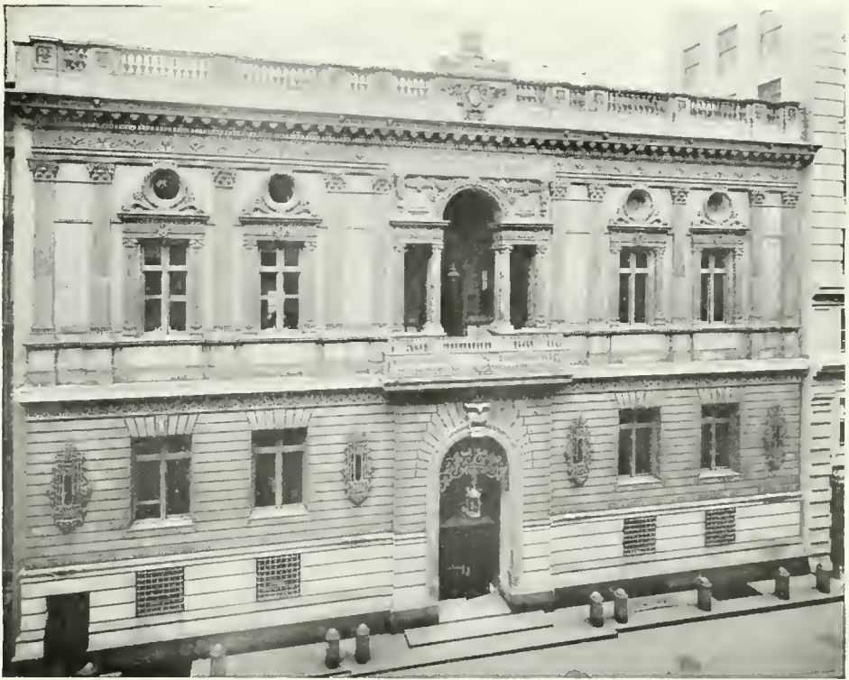
The Century Club, New York City, McKim, Mead & White, Architects. Terra Cotta used for wall finish of lower story above base and ornamental treatment up to and including parapet balustrade.
