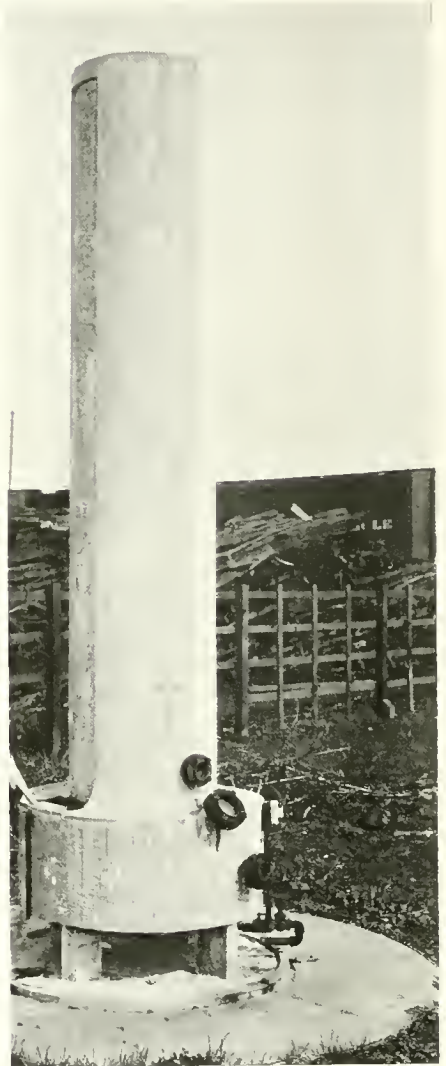
NOVEL TESTING TOWER
