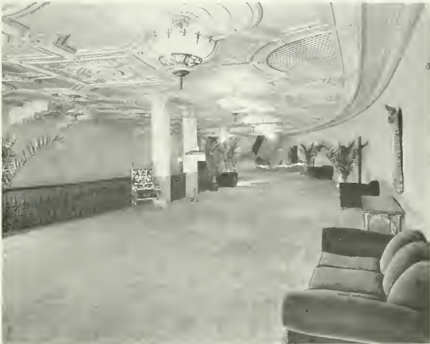
MEZZANINE FLOOR, HILL STREET THEATER, LOS ANGELES G. Albert Lansburgh, Architect
