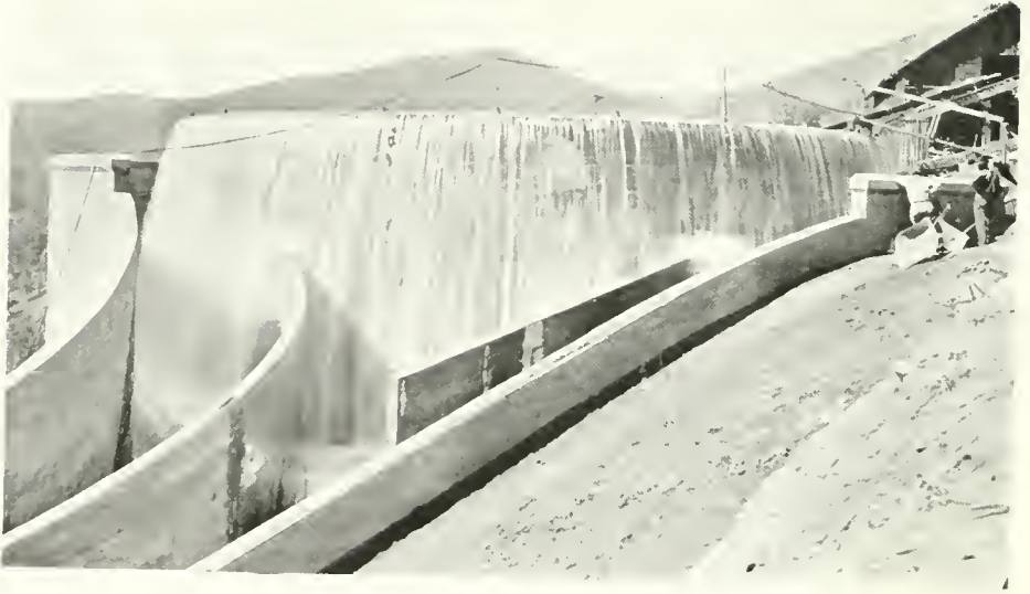
SURGE CHAMBER "SPILLING"
