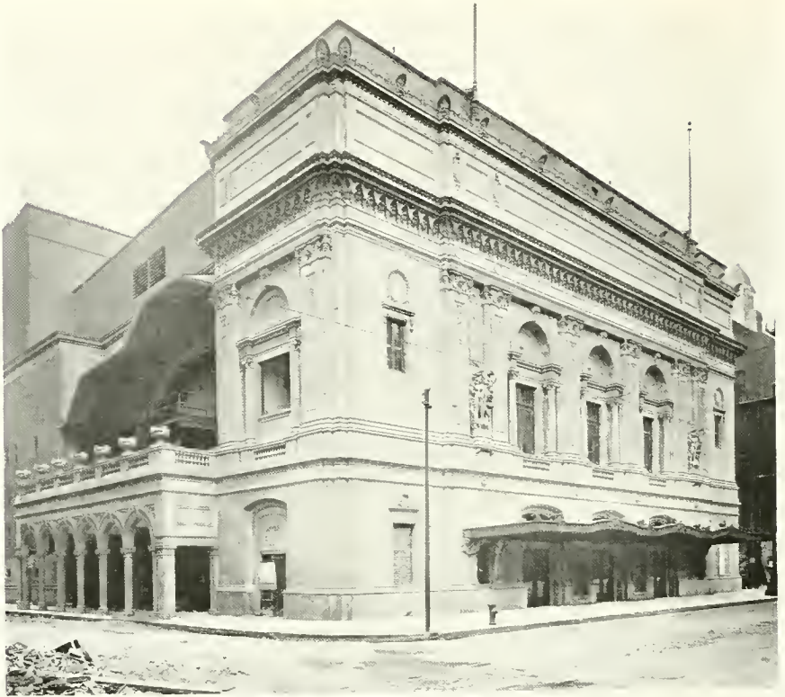
ORPHEUM THEATER, ST. LOUIS, MO. G. Albert Lansburgh, Architect
