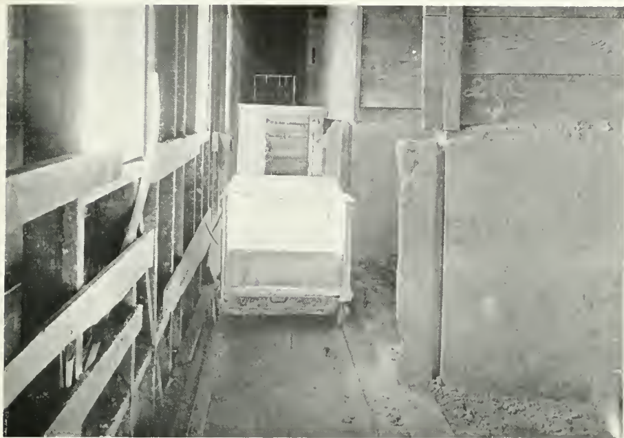
The material bins. The ground materials are stored in these bins and loaded in the necessary quantities on a passing car.
