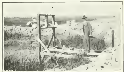
Wooden Lever and Stand for Raising Automatic Gate Valve When Not in Use
