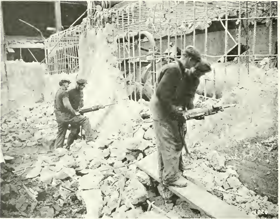
PAVING BREAKERS REMOVING CONCRETE FROM VENTURI VAULT, CLEVELAND, OHIO
