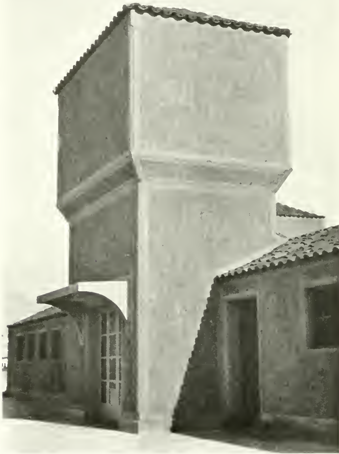
ELEVATOR HOUSE ON ROOF. BUILDING FOR THEO. H. DAVIES & CO. Louis Christian Mullgardt, Architect
