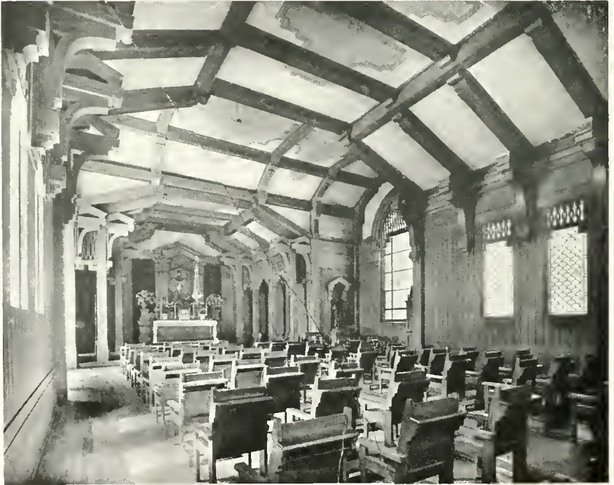
INTERIOR, SCHOOL AT BELMONT John MacQuarrie, Designer
