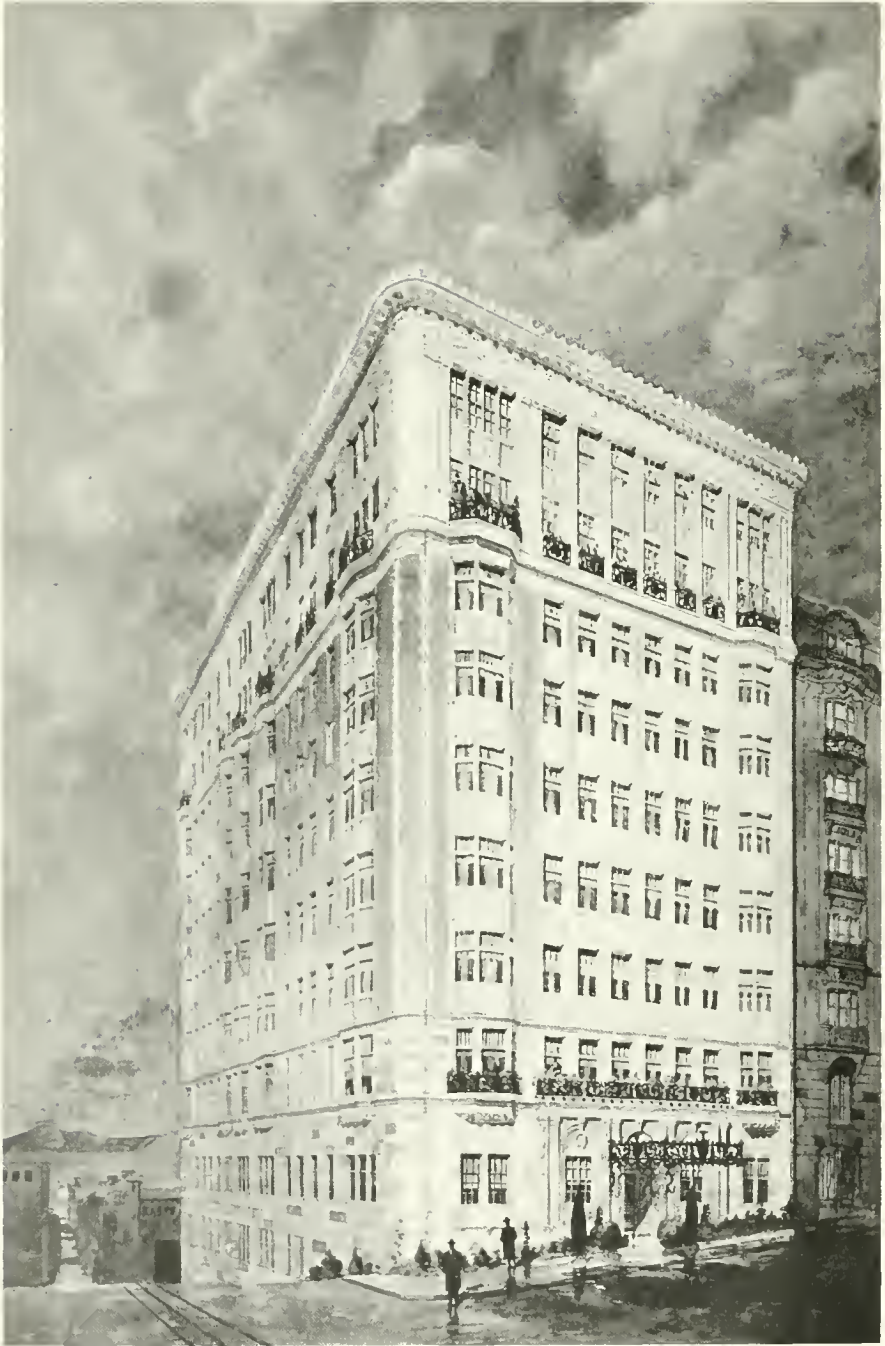
FRANCESCA APARTMENTS, SAN FRANCISCO KENNETH MAC DONALD ARCHITECT MAURICE C. COUCHOT ENGINEER
