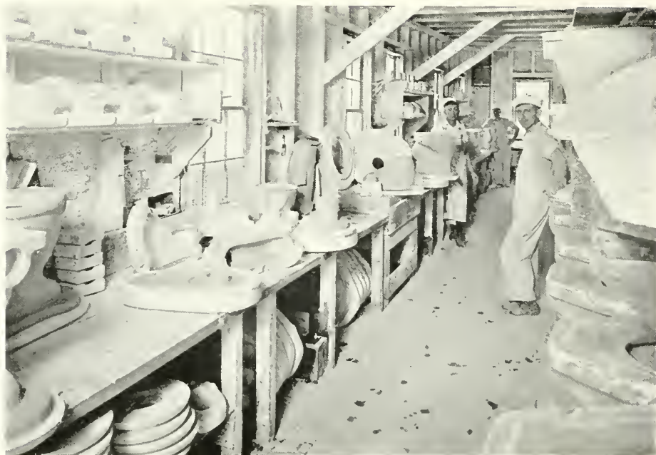
Pressing shops. Toilet bowls in parts and assembled.
