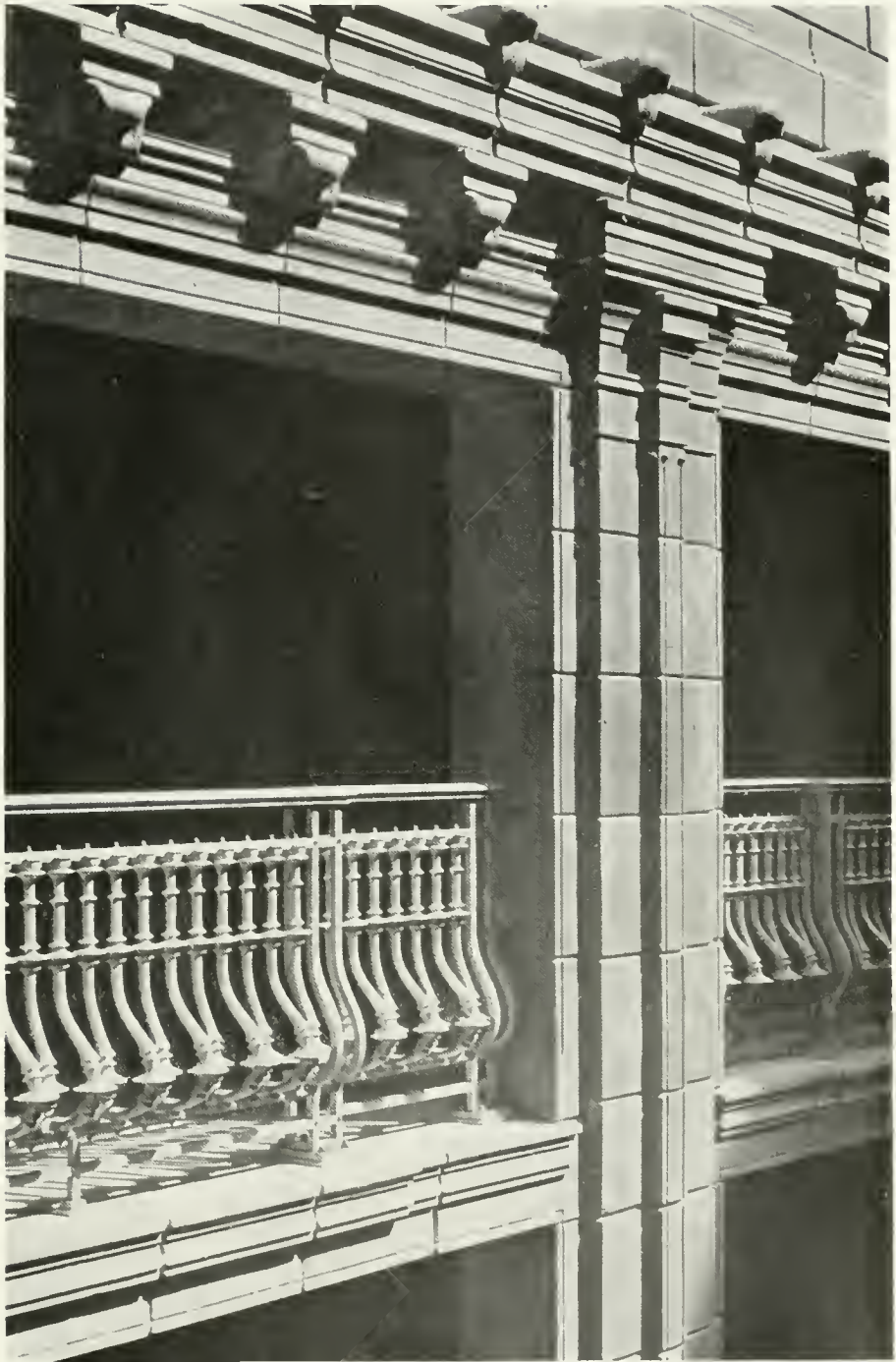
DETAIL OF COURT, BUILDING FOR THEO. H. DAVIES & CO., LTD., HONOLULU, T. H. LOUIS CHRISTIAN MULLGARDT, ARCHITECT
