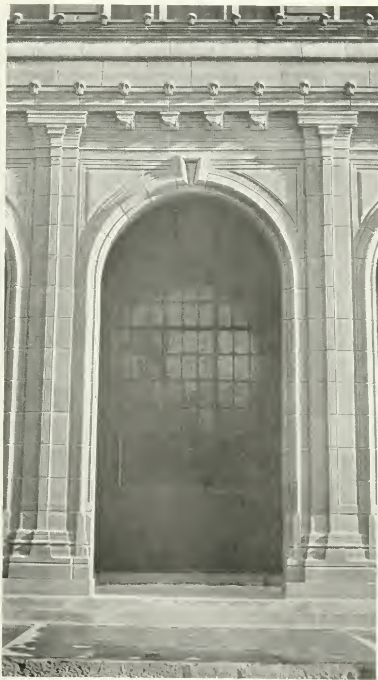
ELEVATION OF ARCH, BUILDING FOR THEO. H. DAVIES & CO., LTD., HONOLULU, T. H. LOUIS CHRISTIAN MULLGARDT, ARCHITECT Terra Cotta manufactured and erected by Gladding, McBean & Co., San Francisco.
