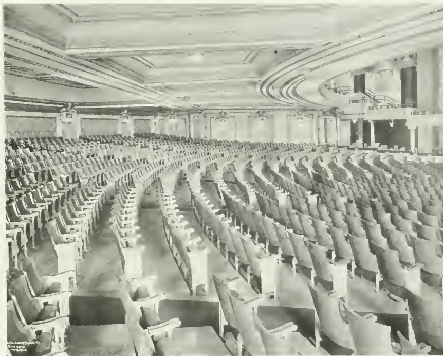
INTERIOR, STATE LAKE THEATER, CHICAGO G. Albert Lansburgh, Architect Kapp and Kapp, Associated Architects
