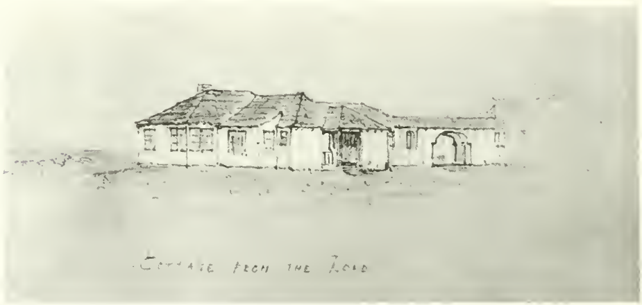
VIEW FROM THE ROAD. COTTAGE FOR MR. AND MRS. HAROLD CHASE. SANDYLAND, NEAR SANTA BARBARA James Osborne Craig, Architect
