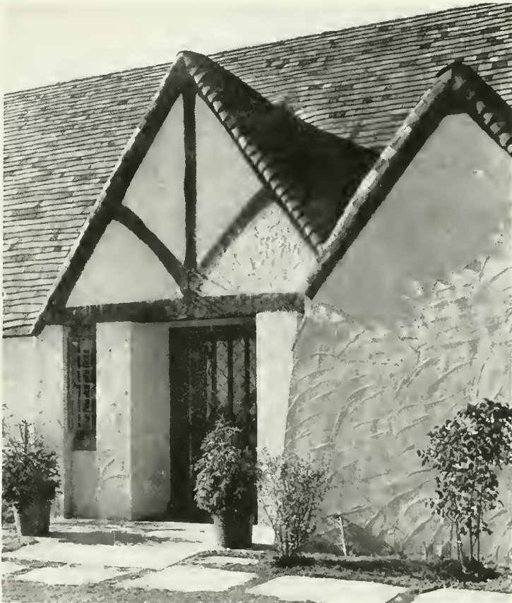
AN INTERESTING TEXTURE THAT SHOWS THE MARKS OF THE TROWEL Bloodgood Tuttle, Architect
