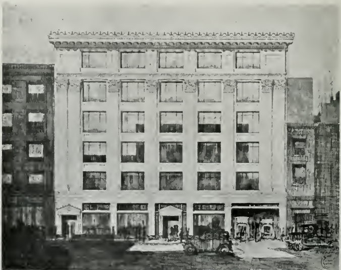
ALTERATIONS, WHOLESALE BUILDING, SAN FRANCISCO S. Heiman, Architect
