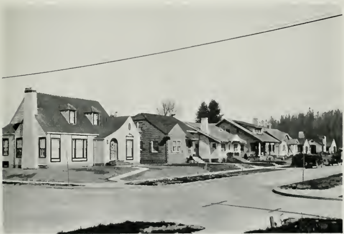
TYPICAL RESIDENCE STREET, LONGVIEW, WASHINGTON
