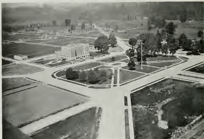
AIR PLANE VIEW, SHOWING HOTEL MONTICELLO AND JEFFERSON SQUARE LONGVIEW, WASHINGTON
