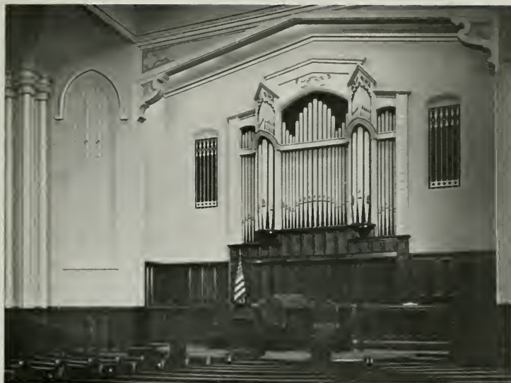
INTERIOR GLENDALE PRESBYTERIAN CHURCH Robert H. Orr, Architect
