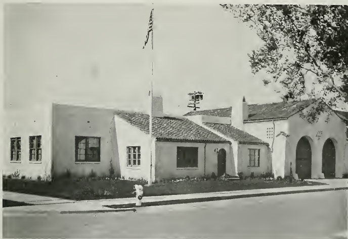
ENGINE HOUSE NO. 8, SACRAMENTO FIRE DEPARTMENT Dean & Dean, Architects
