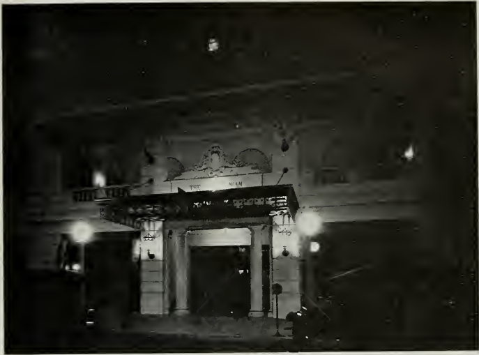
NIGHT ILLUMINATION, ENTRANCE, THE CALIFORNIAN HOTEL, FRESNO H. Rafael Lake and R. F. Felchin and Co., Architects
