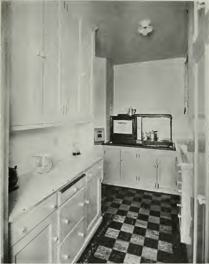
KITCHENETTE, SHOWING ELECTRIC RANGE, HUNTINGTON HOTEL APARTMENTS
