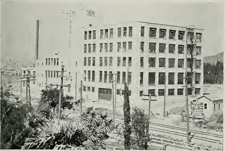
BUILDING FOR THEME HOSIERY COMPANY, LOS ANGELES Lockwood Greene & Co., Engineers
