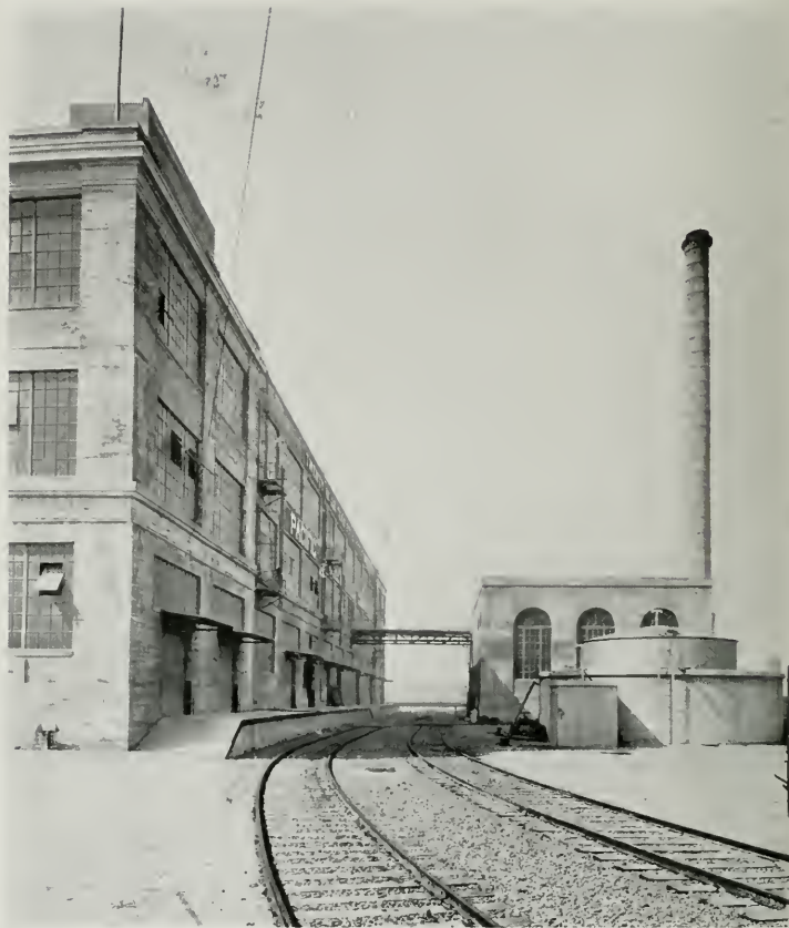
FACTORY FOR PACIFIC COAST BORAX COMPANY, WILMINGTON Albert C. Martin, Architect
