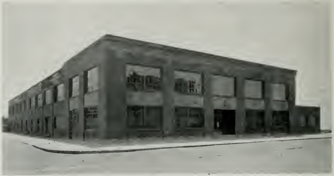
BUILDING FOR GRINNELL COMPANY, SAN FRANCISCO The Austin Company, Builders
