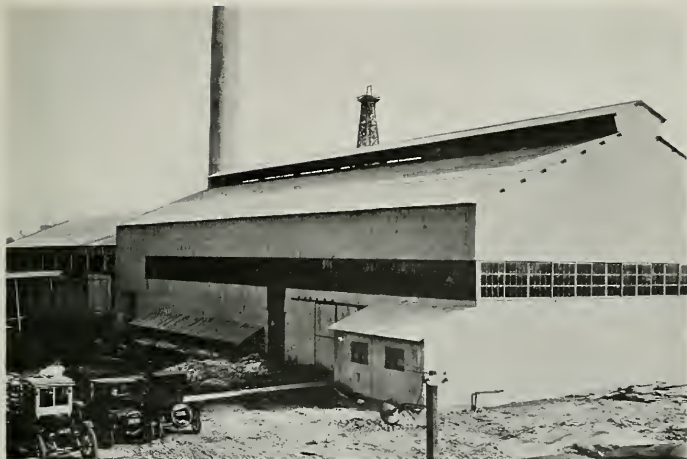
PLANT OF WESTERN SHEET GLASS COMPANY, TORRANCE, CALIFORNIA Roofed and sided with galvanized sheet metal
