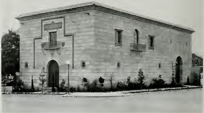
SUB-STATION C., SAN DIEGO CONSOLIDATED GAS AND ELECTRIC CO. Requa and Jackson, Architects
