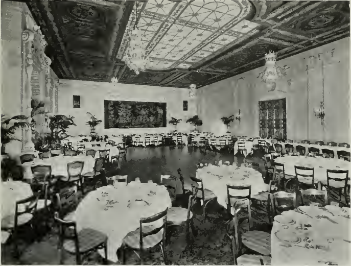
MUSIC ROOM, LOS ANGELES BILTMORE Schultze and Weaver, Architects
