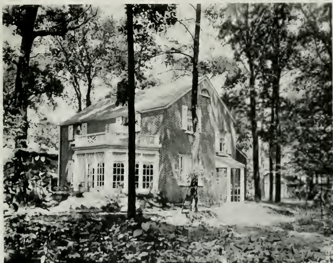
A BRICK COLONIAL HOUSE IN ILLINOIS Bernard C. Greengard, Architect
