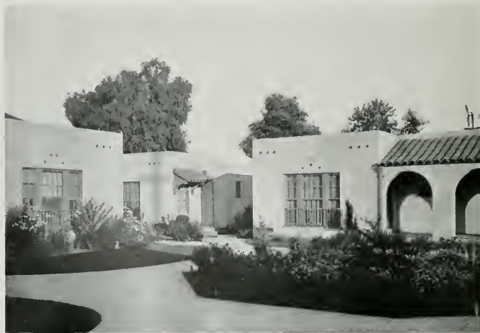
BUNGALOW COURT, PALO ALTO Birge M. Clark, Architect
