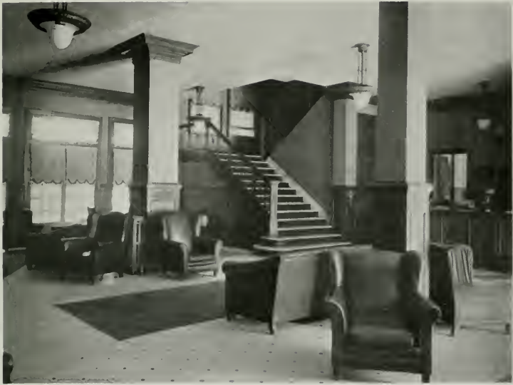
LOBBY, Y. M. C. A. BUILDING, POMONA Robert H. Orr, Architect
