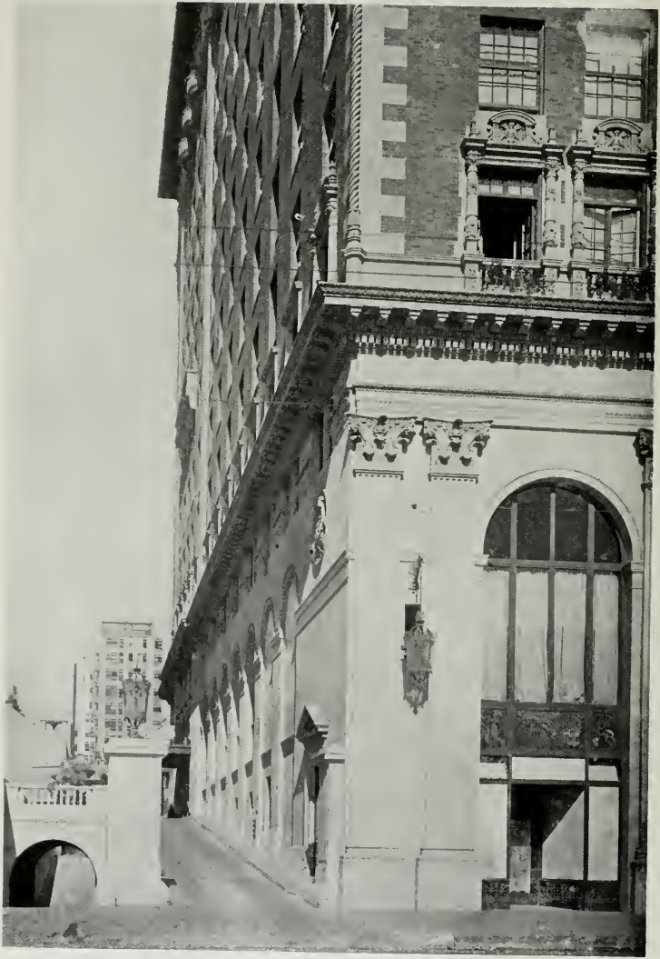
AUTOMOBILE RAMPS, LOS ANGELES BILTMORE SCHULTZE AND WEAVER, ARCHITECTS
