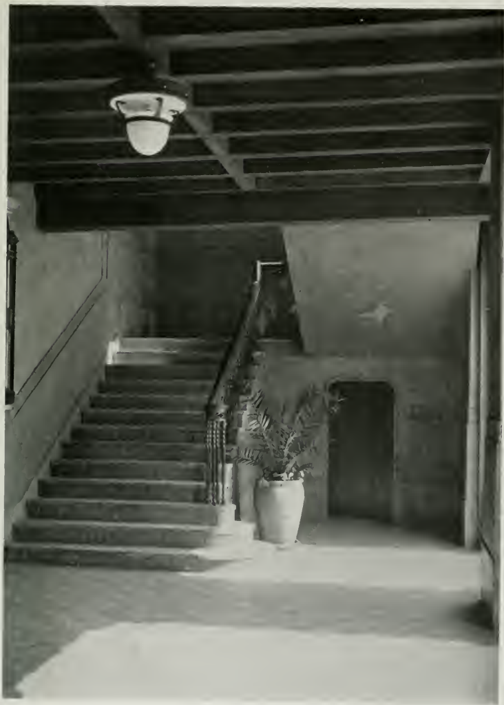
ENTRANCE STAIRWAY HOLLYWOOD HOSPITAL. ROBERT H. ORR, ARCHITECT
