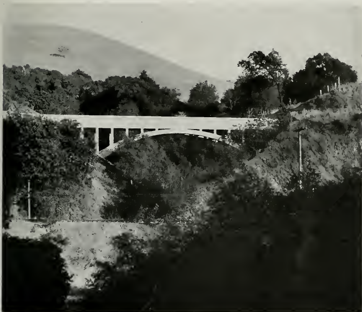
SPRING VALLEY'S SUNOL AQUEDUCT, WITH A CAPACITY OF SEVENTY MILLION GALLONS DAILY, WILL CARRY CALAVERAS WATER DOWN NILES CANYON
