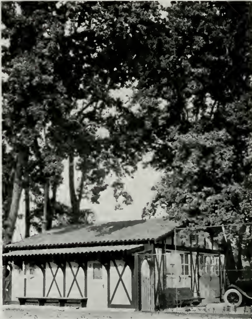
GARAGE FOR MR. H. V. KEELING, LAKEPORT, CALIFORNIA Morrow & Garren, Architects
