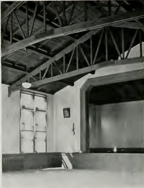
AUDITORIUM, LAKEPORT UNION SCHOOL, LAKEPORT, CALIFORNIA Morrow & Garren, Architects
