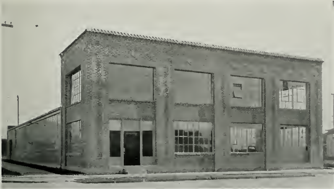
BUILDING FOR STANDARD DIE & SPECIALTY CO., BERKELEY The Austin Company, Builders
