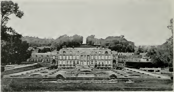
CHATEAU DE DAMPIERRE South Exposure and Gardens
