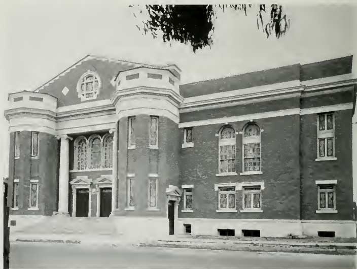
FIRST CHRISTIAN CHURCH, SANTA MONICA Robert H. Orr, Architect
