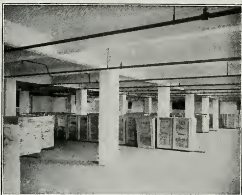
INTERIOR OF A STOREHOUSE AFTER FIRE. NOTE CONDITION OF THE CONTENTS AND THE SPRINKLER HEAD THAT WAS NOT FUSED INDICATING LOW TEMPERATURE AT ALL TIMES.
