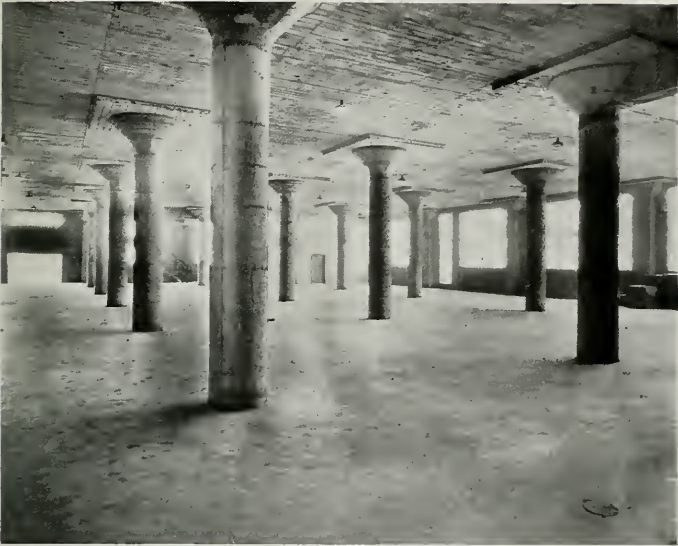
TYPICAL FLOOR, FACTORY FOR PACIFIC COAST BORAX COMPANY, WILMINGTON Albert C. Martin, Architect
