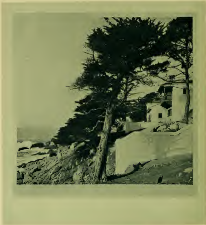
HOUSE OF MR. AND MRS ARTHUR ROSE VINCENT PEBBLE BEACH, CALIFORNIA GEORGE WASHINGTON SMITH, ARCHITECT
