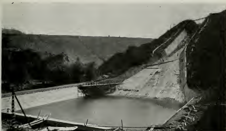
SPILLWAY OF CALAVERAS DAM, SEPTEMBER, 1924. THE TOP OF THE DAM IS SEEN ON THE SKYLINE
