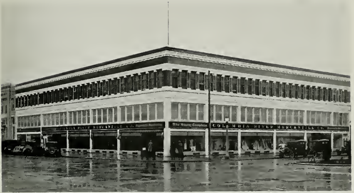
STORE BUILDING FOR COLUMBIA RIVER MERCANTILE COMPANY, LONGVIEW, WASH.
