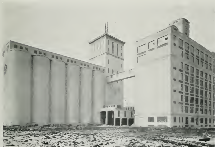
SPERRY FLOUR MILLS, OGDEN, UTAH Maurice C. Couchot and Jesse Rosenwald, Architects
