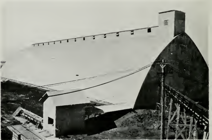
SEED HOUSE FOR THE SAN DIEGO OIL PRODUCTS COMPANY Over 32,475 pounds of 26 gauge Armeo Ingot Iron used for roof and sides
