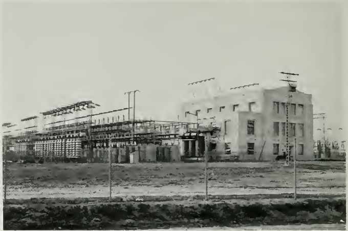
LAGUNA BELL SUBSTATION, SOUTHERN CALIFORNIA EDISON COMPANY, LOS ANGELES
