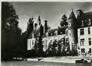
WEST FACADE, CHATEAU ST. MESME OLD AND NEW PORTION
