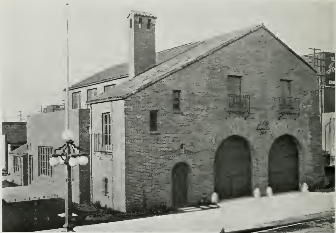
ENGINE HOUSE NO. 1, SACRAMENTO FIRE DEPARTMENT Dean & Dean, Architects
