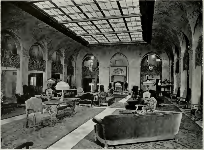
LOBBY, HOTEL SENATOR, SACRAMENTO MacDonald and Couchot, Architect and Engineer
