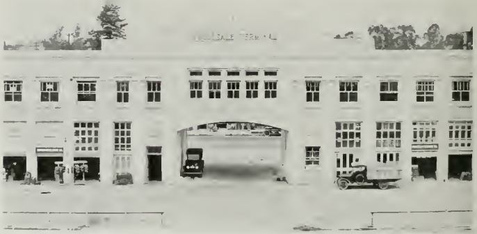
ENTRANCE TO MARKET YARD, WHOLESALE TERMINAL, LOS ANGELES John Parkinson and Donald B. Parkinson, Architects
