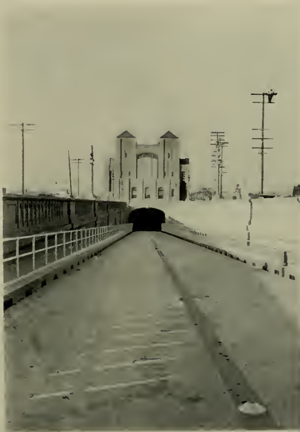
ALAMEDA APPROACH TO TUBE AND VENTILATION EQUIPMENT BUILDING AT PORTAL
