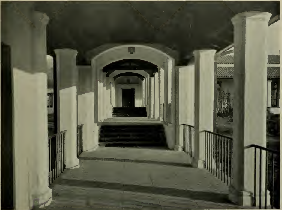
ARCADE, ST. MARY'S COLLEGE, CALIFORNIA John J. Donovan, Architect
