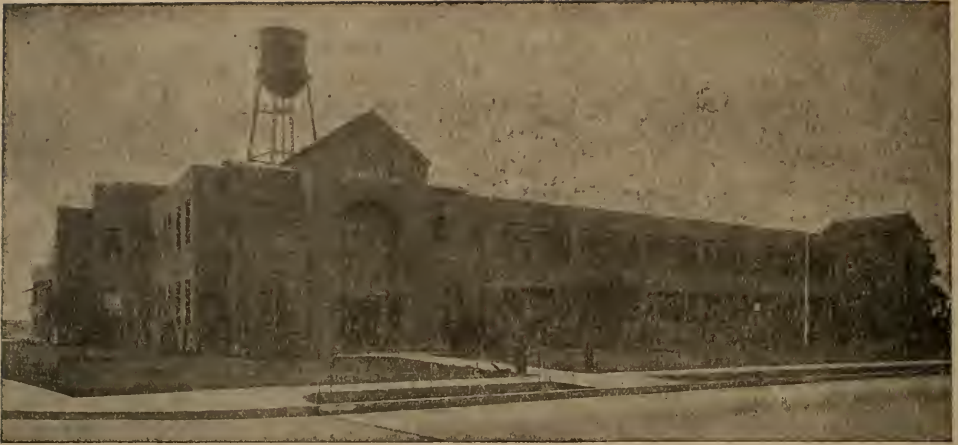
Kitinger Furniture Factory, Industrial & Pacific Streets, Los Angeles, California. Builders, Wm. P. Neil Company.
