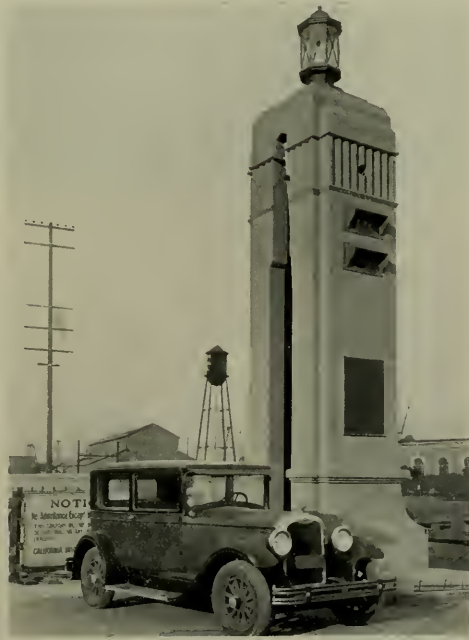
CONCRETE APPROACH WALL PYLON SHOWING TRAFFIC GATE, SIREN AND SIGNALS
