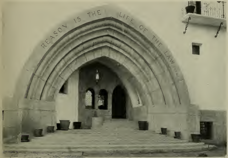
FIGUEROA STREET ENTRANCE, COURT HOUSE, SANTA BARBARA William Mooser Co., Architects
