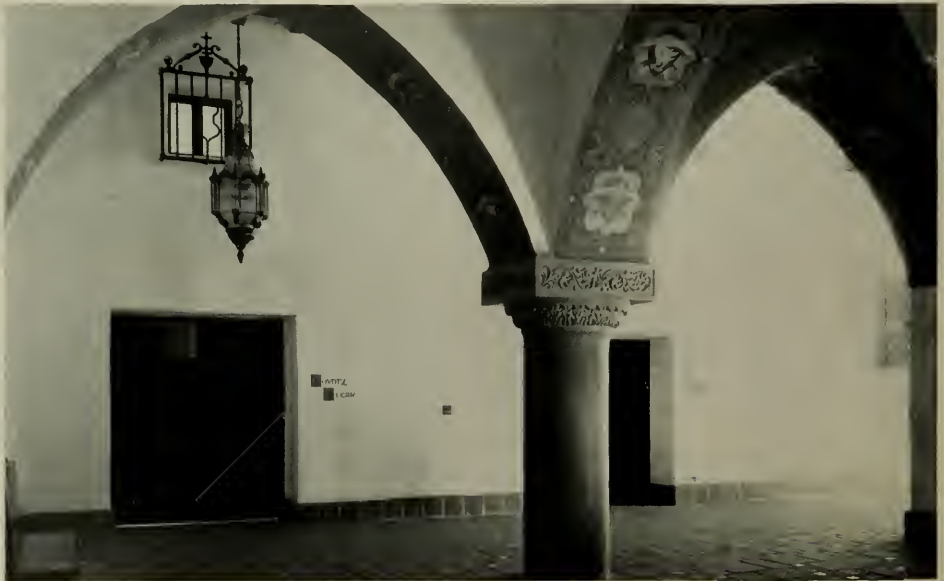
ASSEMBLY GALLERY, COURT HOUSE, SANTA BARBARA William Mosser Co., Architects
