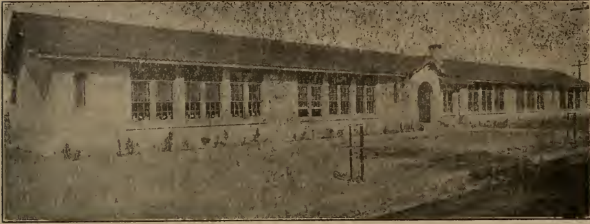
Wasco Grammar School. Architect for first unit, Ernest J. Kump. En- trance and additions de- signed by Symmes and Cullimore, Bakersfield. G. A. Graham, General Contractor. Lowell Strong, Plasterer.
