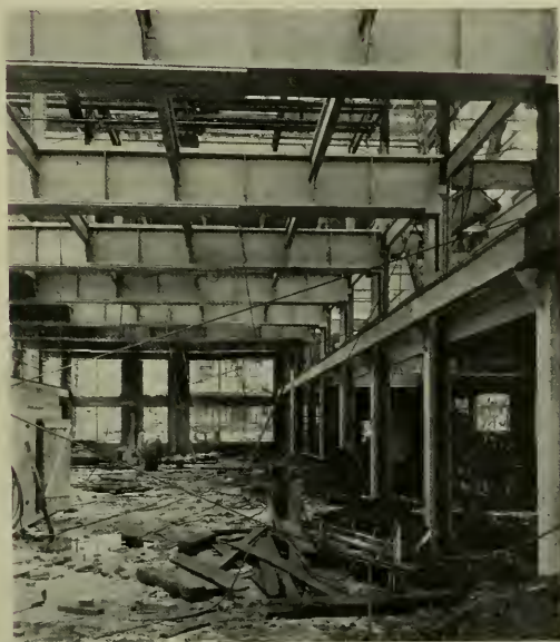
WELDED PLATE GIRDERS IN SHARON BUILDING, SHARON, PENNSYLVANIA
