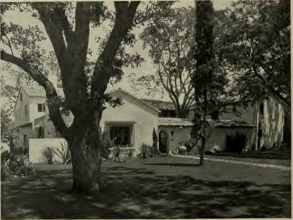
HOUSE OF CHAS. AND KATHLEEN NORRIS, PALO ALTO Birge N. Clark, Architect
