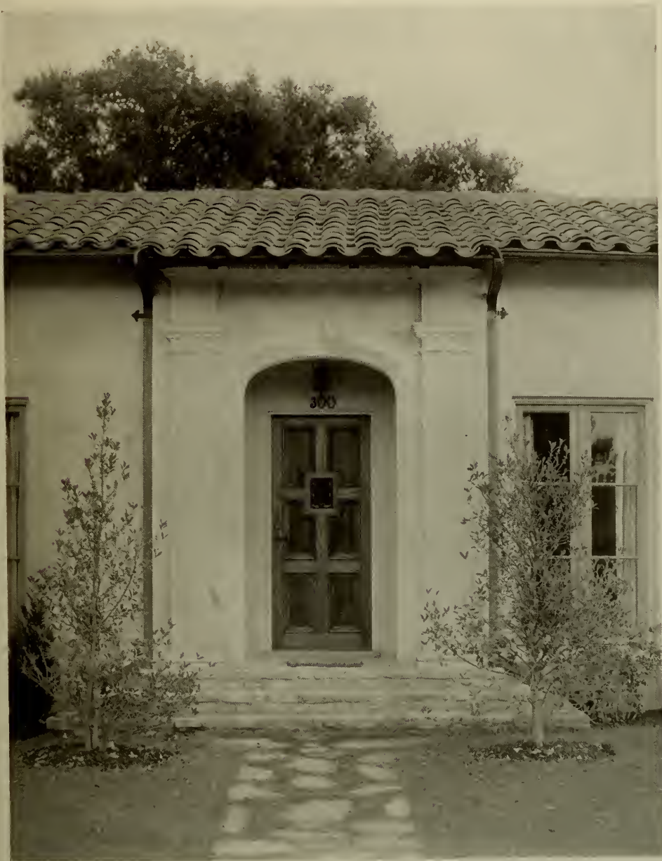
DETAIL, HOUSE OF MRS. F. W. HUNT, PALO ALTO, CALIFORNIA JOHN K. BRANNER, ARCHITECT
