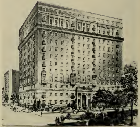
TOWNHOUSE APARTMENTS, LOS ANGELES
