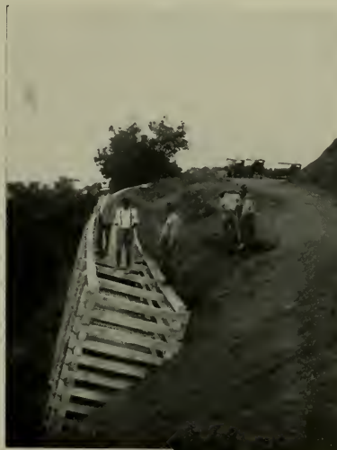
PICTURE SHOWS GENERAL CONSTRUCTION VIEW BEING BACK-FILLED
