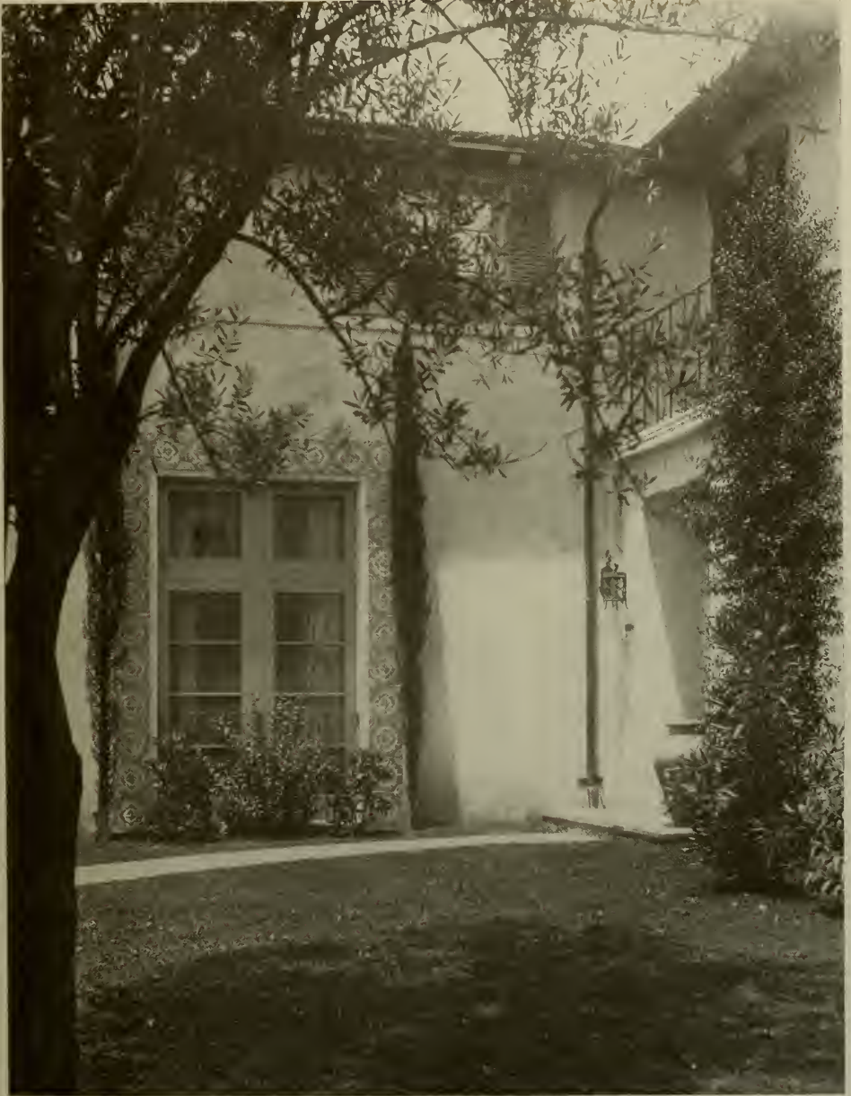
DETAIL, COMPETITION HOUSE BUILT FOR MR. VAN JOHNSTONE, SAN MARINO HENRY C. NEWTON AND ROBERT D. MURRAY, ARCHITECTS
