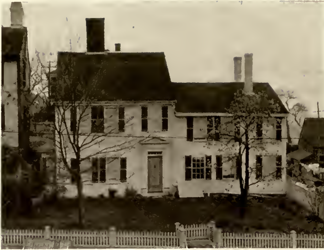
Mr. Low's house on North Street (overlooking the bay).
