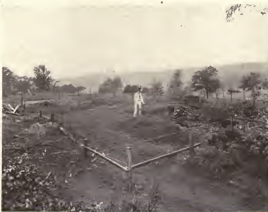
Laying out the work on the ground.
