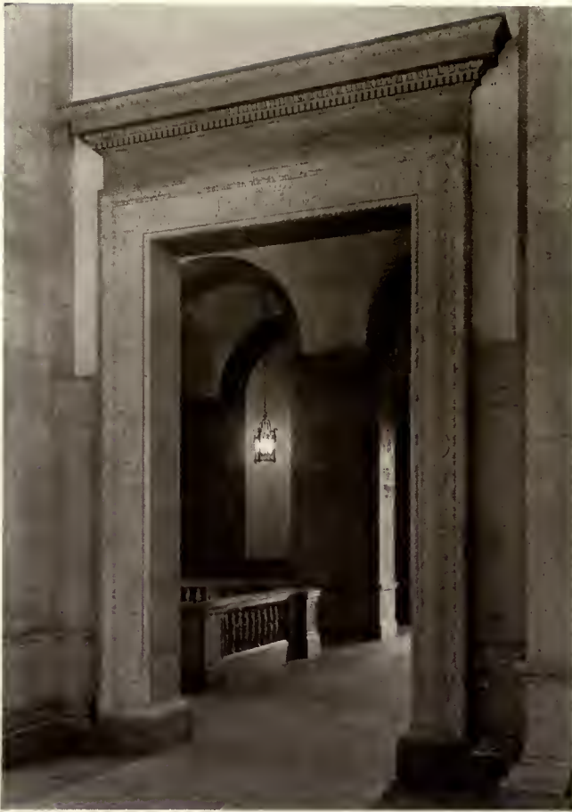
DOORWAY, FIRST FLOOR.
