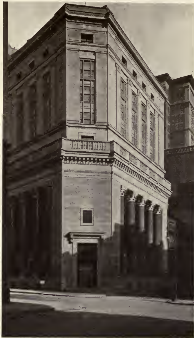
SEABOARD NATIONAL BANK BUILDING, NEW YORK ALFRED C. BOSSOM, Architect Equipped with Sturtevant Apparatus
