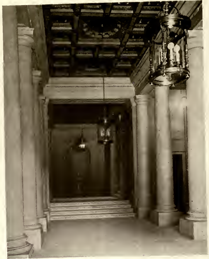
ENTRANCE-HALL AND MAIN STAIR.
