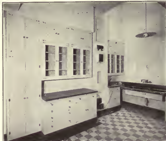
A view of one of the Pantries where our Standard Size Units were laid out to comply with dimensions and requirements.
