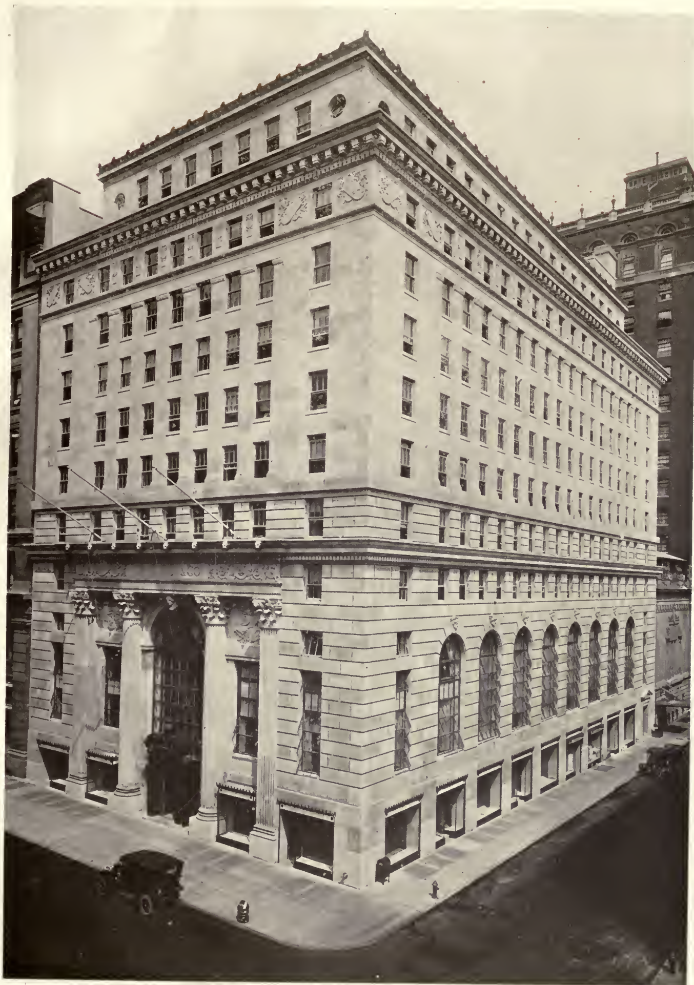
BANKING-HOUSE, S. W. STRAUS & CO., FIFTH AVENUE AND 46TH STREET, NEW YORK.
