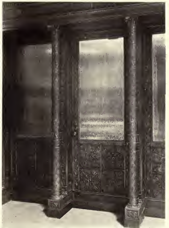
DOORS TO DELIVERY-ROOM.
