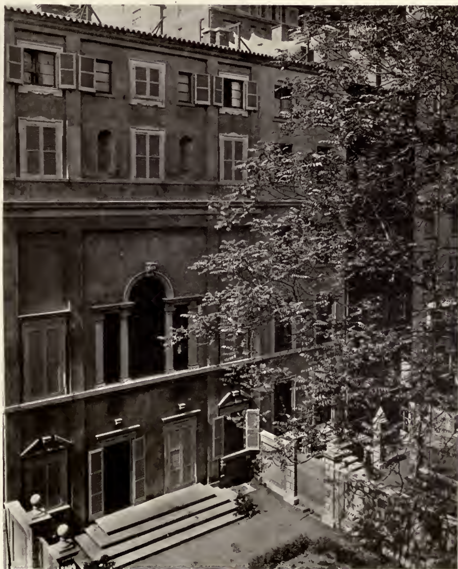
REAR OF HOUSE AND GARDEN.
