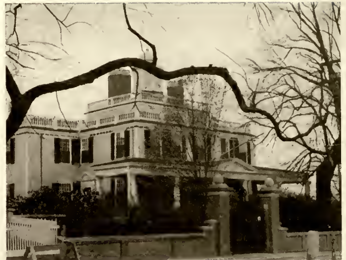
Edward Winslow house, North Street, Plymouth, built 1754 (after alterations).
