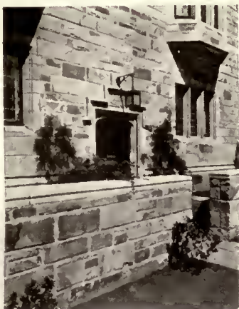
King Entry, Branford Court.
