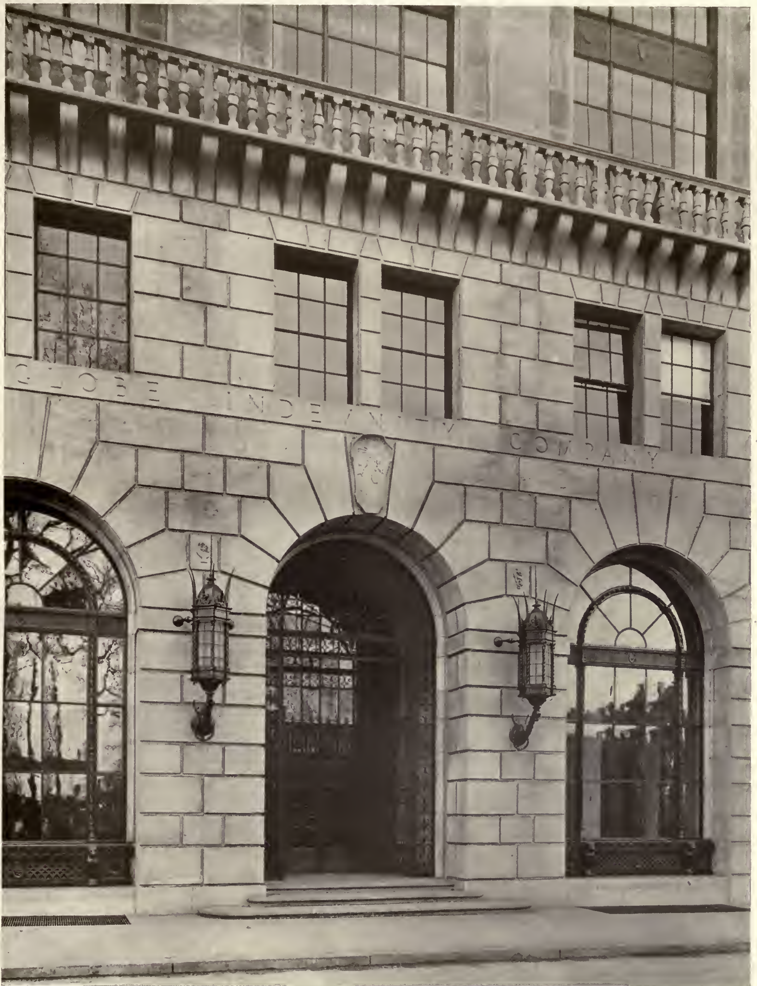
MAIN ENTRANCE, ADMINISTRATION BUILDING, GLOBE INDEMNITY CO., NEWARK, N. J.
