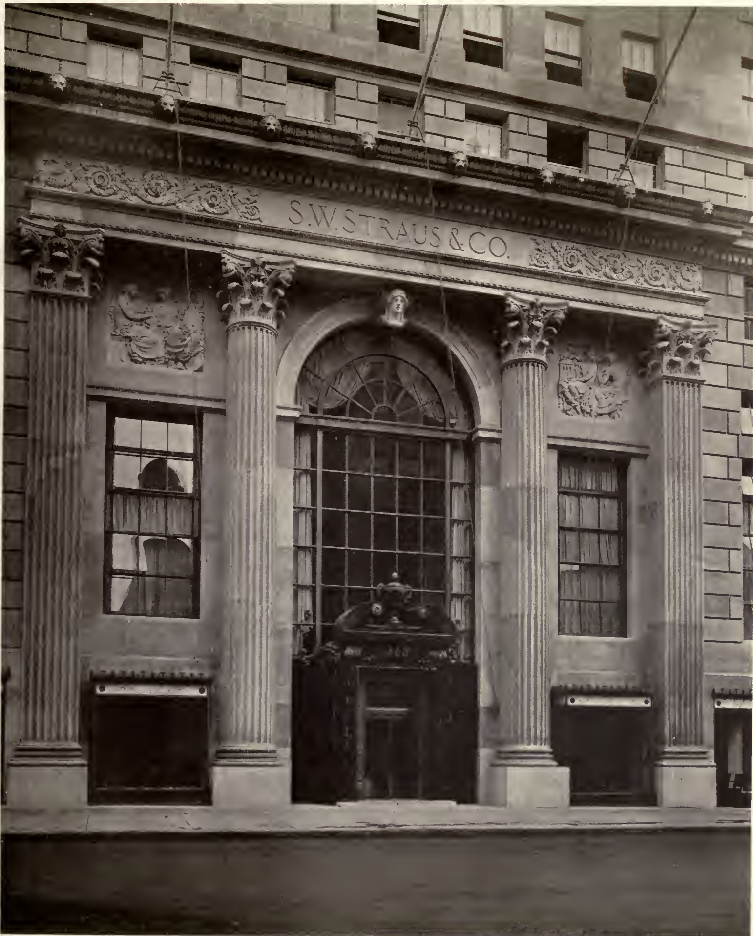
ENTRANCE DETAIL, BANKING-HOUSE, S. W. STRAUS & CO., FIFTH AVENUE AND 46TH STREET, NEW YORK.
