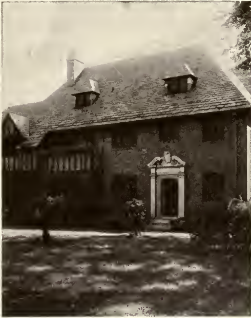
RAPHAEL HUME, ARCHITECT
