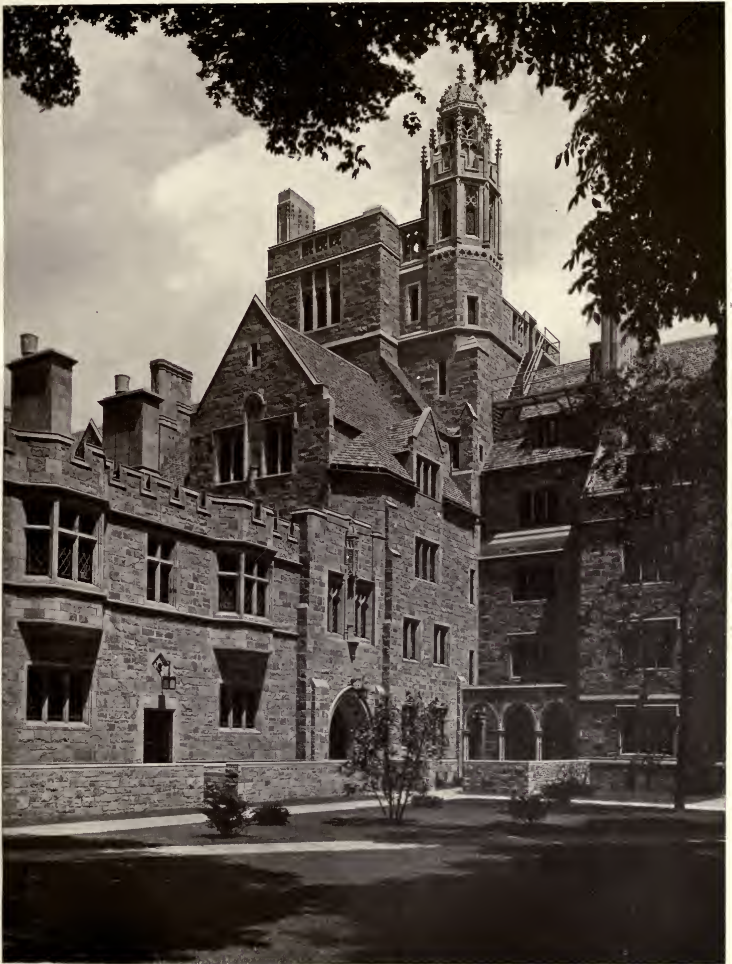
TOURELLE AT NORTHEAST ANGLE OF BRANFORD COURT.
