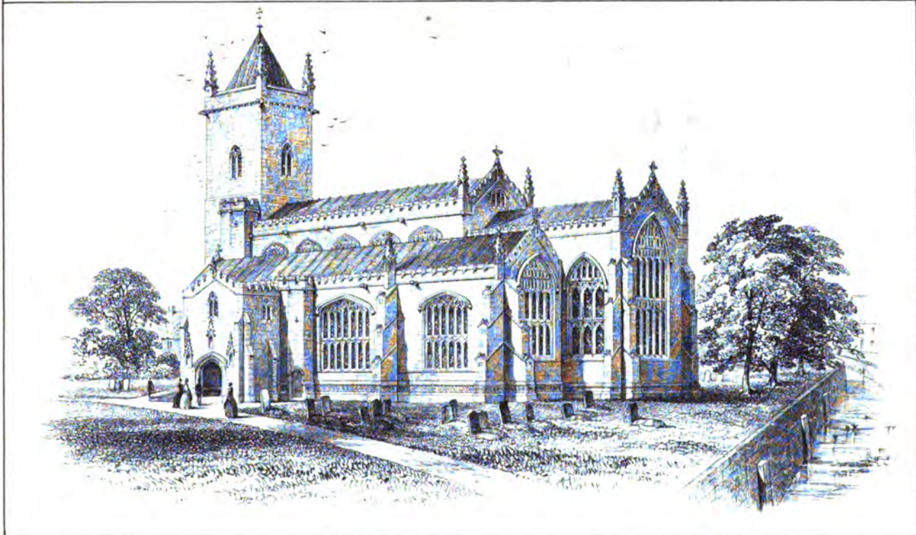
S. E. VIEW OF OUTWELL CHURCH. NORFOLK (Restored)
