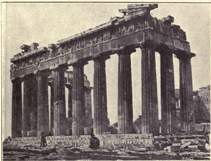
FIG. 335. — Doric order of the Parthenon.
