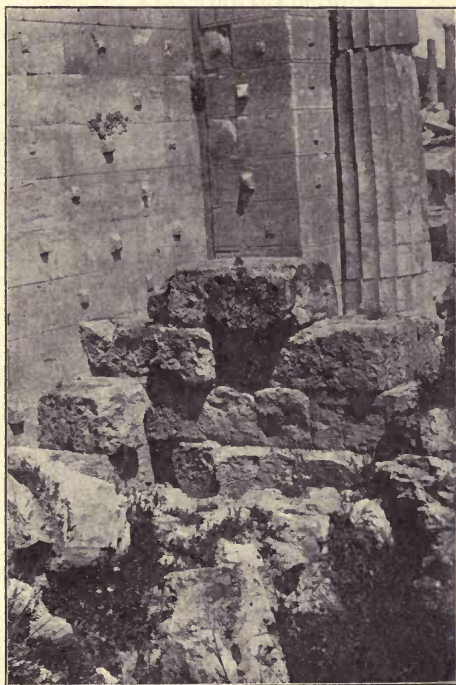
FIG. 20.—Anathyrosis from wall of Propylaea, Athens.
