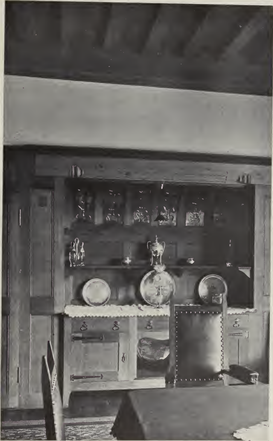
THE DINING-ROOM SIDBOARD AT BRAHAN, PERTH. THIS FITTING IS MADE OF AUSTRIAN OAK, AND IS LEFT CLEAN FROM THE TOOL THE REPOUSSÉE COPPER PANELS ARE BY MR. EDGAR SIMPSON AND THE HANDLES AND HINGES BY MR. R. LL. RATHBONE
