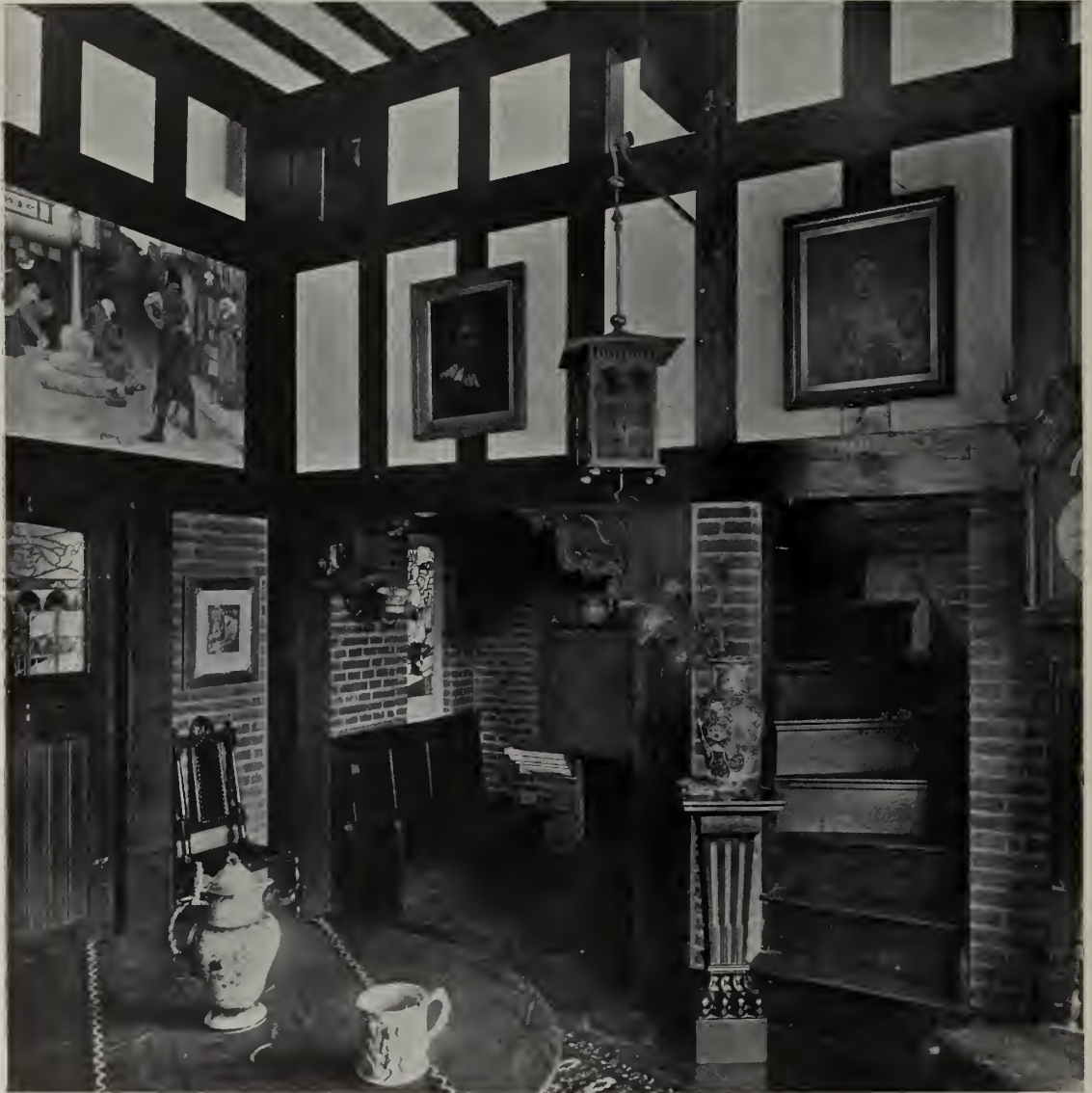
VIEW TOWARDS THE INGLE-NOOK IN THE HALL OF MR. CROUCH'S HOUSE AT SUTTON COLDFIELD, WARWICKSHIRE. THE SOLID CONSTRUCTIONAL BEAMS AND POSTS AND BRACKETS GIVE SIMPLICITY AS WELL AS STRENGTH. THE FRIEZE, MEASURING 14 FT. BY 3 FT. 6 IN., IS BY FRED DAVIS, R.I., AND FORMS PART OF A SCHEME ILLUSTRATING MORRIS'S "DREAM OF JOHN BALL." THE UPPER PORTION OF THE HALL IS IN OAK AND PLASTER, WHILE THE LOWER PART IS BUILT OF RED SAND-FACED BRICKS FROM LEICESTERSHIRE, VERY RICH AND VARIED IN COLOUR. THE GLASS WINDOWS ON EACH SIDE OF THE INGLE, BY MARY NEWILL, REPRESENT JOHN BALL AND WAT TYLER
