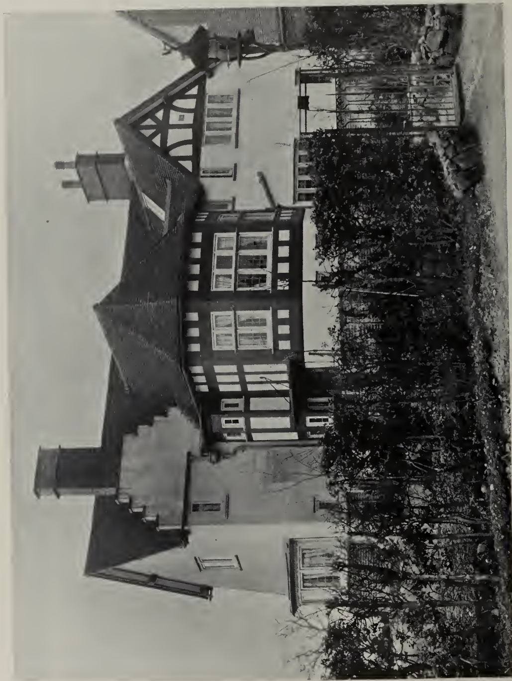
MR. BUTLER'S HOUSE AT SUTTON COLDFIELD, WARWICKSHIRE. MATERIALS: HALF-TIMBER AND PLASTER, 2 IN. LEICESTERSHIRE BRICKS, AND HANDMADE TILES
