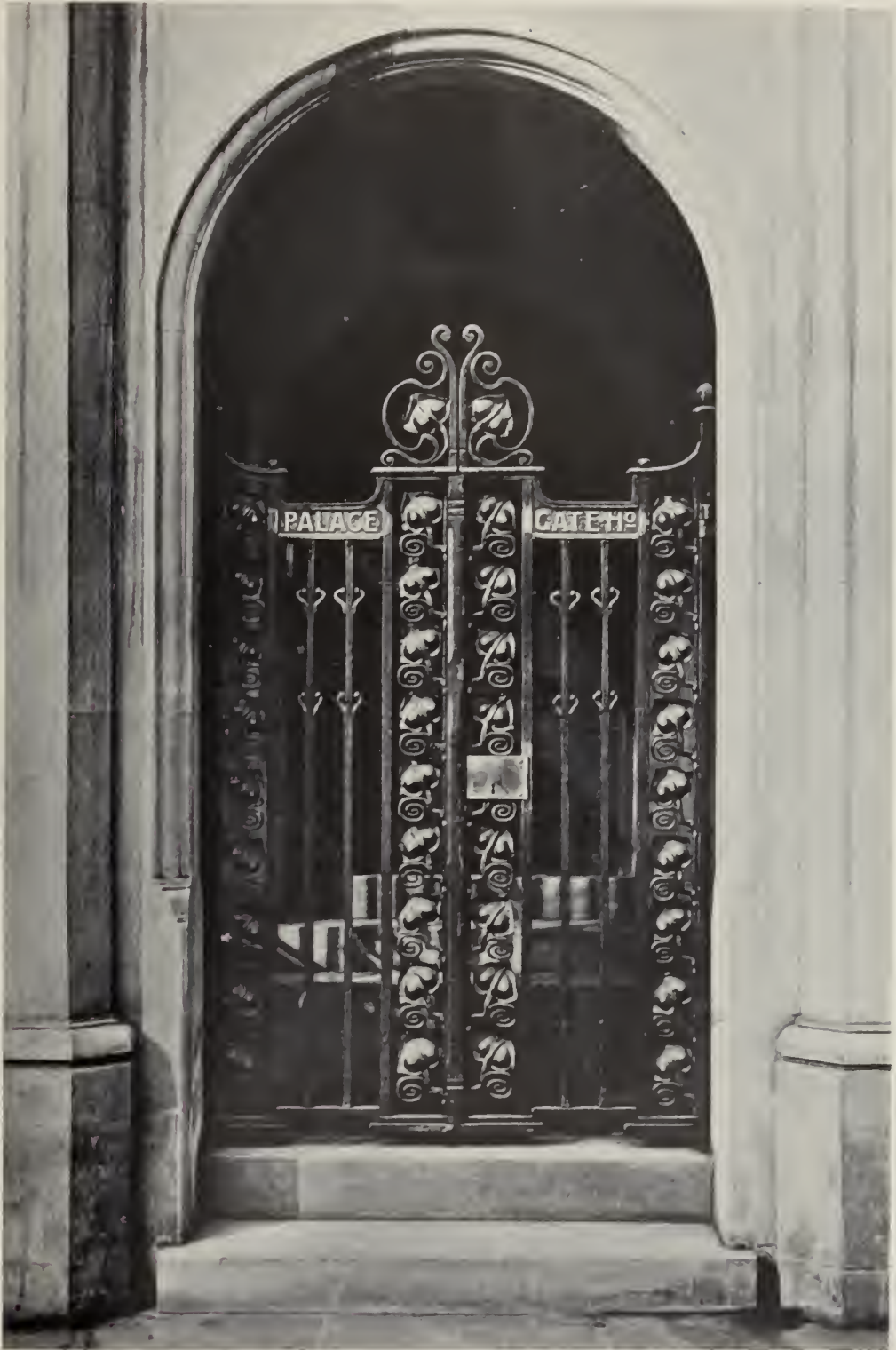
FORGED IRON GATE TO PALACE GATE HOUSE, KENSINGTON. THIS GATE WAS NOT MADE IN THE USUAL MODERN MANNER BY SCREWING OR FITTING TOGETHER A NUMBER OF SMALL PIECES; IT WAS FORGED THROUGHOUT IN THE THIRTEENTH CENTURY MANNER
