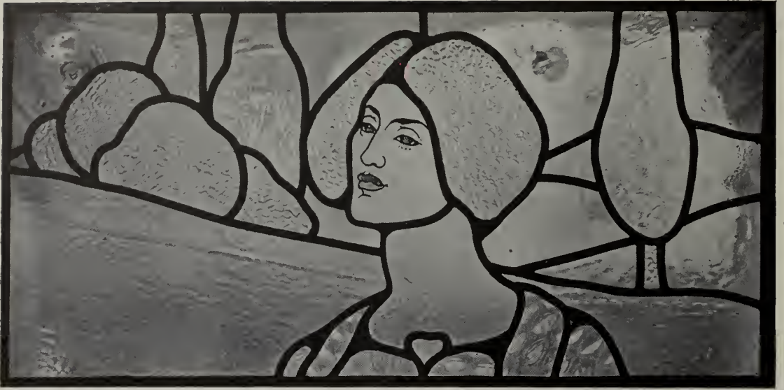
FANLIGHT OVER A DOOR, CARRIED OUT ENTIRELY IN WHITE GLASSES OF VARIOUS TEXTURES. THE SKY IS OF CROWN GLASS, WITH THE "BULLIONS" LEFT IN; THE ROUNDED CORNERS ARE FORMED, NOT BY PAINTING, BUT BY CARRYING THE LEAD ROUND
