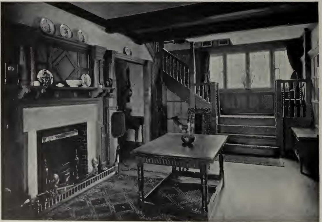
THE HALL, TOYS HILL, KENT. THE PANELLING AND FLOOR ARE OF WAINSCOT OAK, AND THE STAIRS WERE BUILT UP WITH OLD BALUSTERS. THE MATERIALS USED IN THE BUILDING OF THE HOUSE WERE LYMPFIELD COURSED RAG-STONE AND HOWLEY PARK STONE, THE FIRST HAVING A RICH YELLOW TONE, THE OTHER A STRONG GREY
