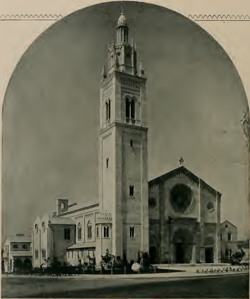
Wiltshire Boulevard Church, Los Angeles, California, one of many fine examples of monolithic exposed concrete Allison and Allison, Architects, Los Angeles.
