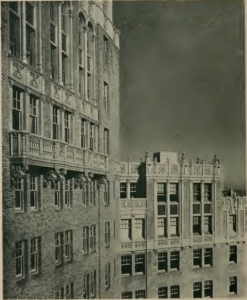
DETAIL, 15TH FLOOR, HOTEL MARK HOPKINS, SAN FRANCISCO, CALIF. WEEKS & DAY, ARCHITECTS
