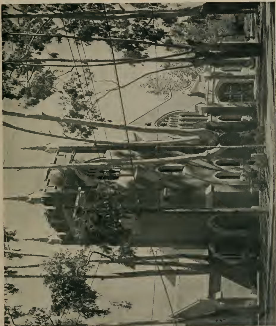
St. Paul's Episcopal Church, Burlingame, Calif. Wm. C. F. Gillam, Architect ARCHITECTURAL EXHIBITION, NORTHERN CALIFORNIA CHAPTER, A. I. A., SAN FRANCISCO, CALIFORNIA
