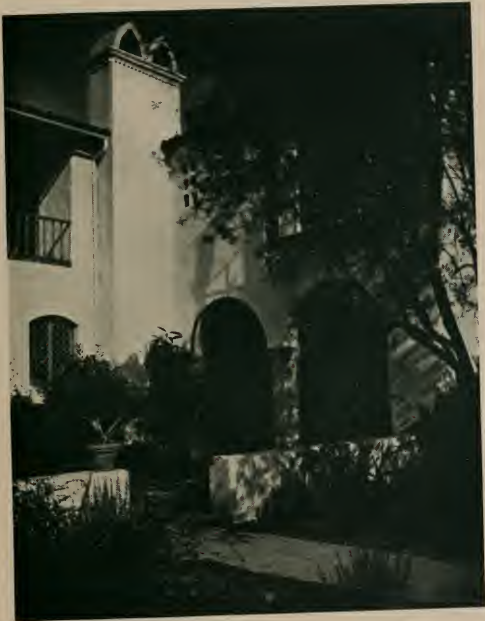
LOGGIA—RESIDENCE FOR MR. MILTON BARUCH, LOS ANGELES, CALIFORNIA GORDON B. KAUFMANN, ARCHITECT
