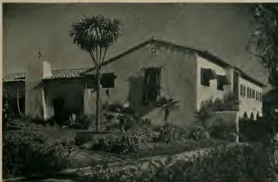
RESIDENCE FOR MR. ROBERT OVERELL, LOS ANGELES, CALIFORNIA DESIGNED BY DAVID MALCOLM MASON
