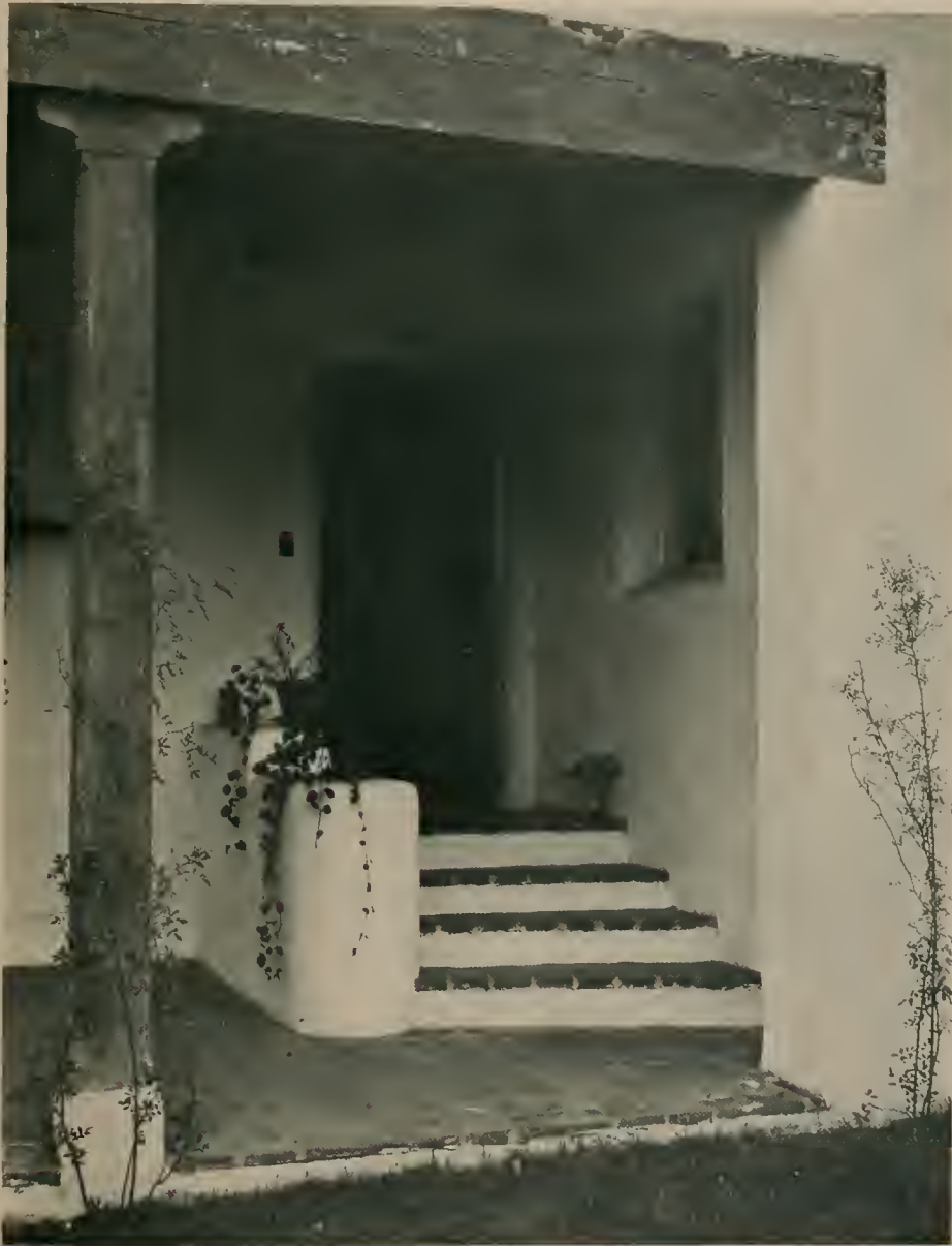
LOGGIA DETAIL—A HOUSE IN PASADENA, CALIF. ROLAND E. COATE, ARCHITECT
