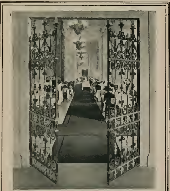
Ornamental Gridded Gates to Dining Room, Enlarged Clift Hotel, San Francisco. Schultze & Weaver, Architects.
