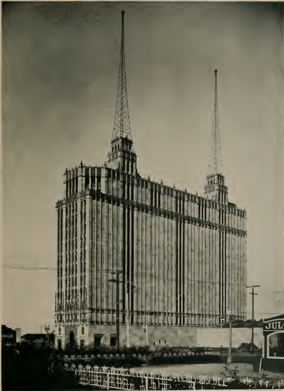
HOLLYWOOD STORAGE WAREHOUSE, LOS ANGELES, CALIF. MORGAN, WALLS AND CLEMENTS, ARCHITECTS
