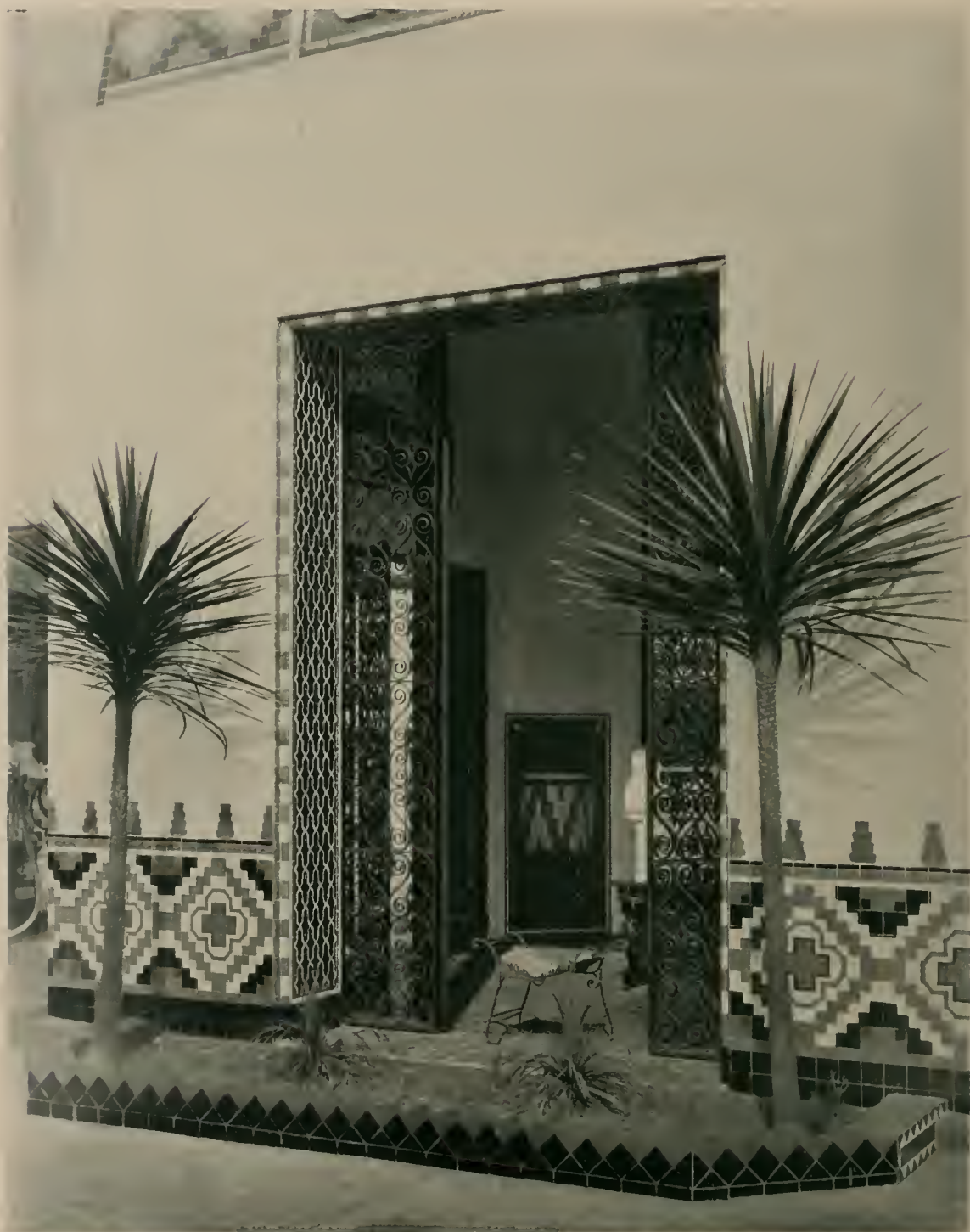
Decorative Tile in black, red, and white carries out the Carpet color scheme in this distinctive filling station at Los Angeles. Roland E. Coate, Architect. The style is Tunisian, and under the warm, white Southern sunlight it is most attractive.
