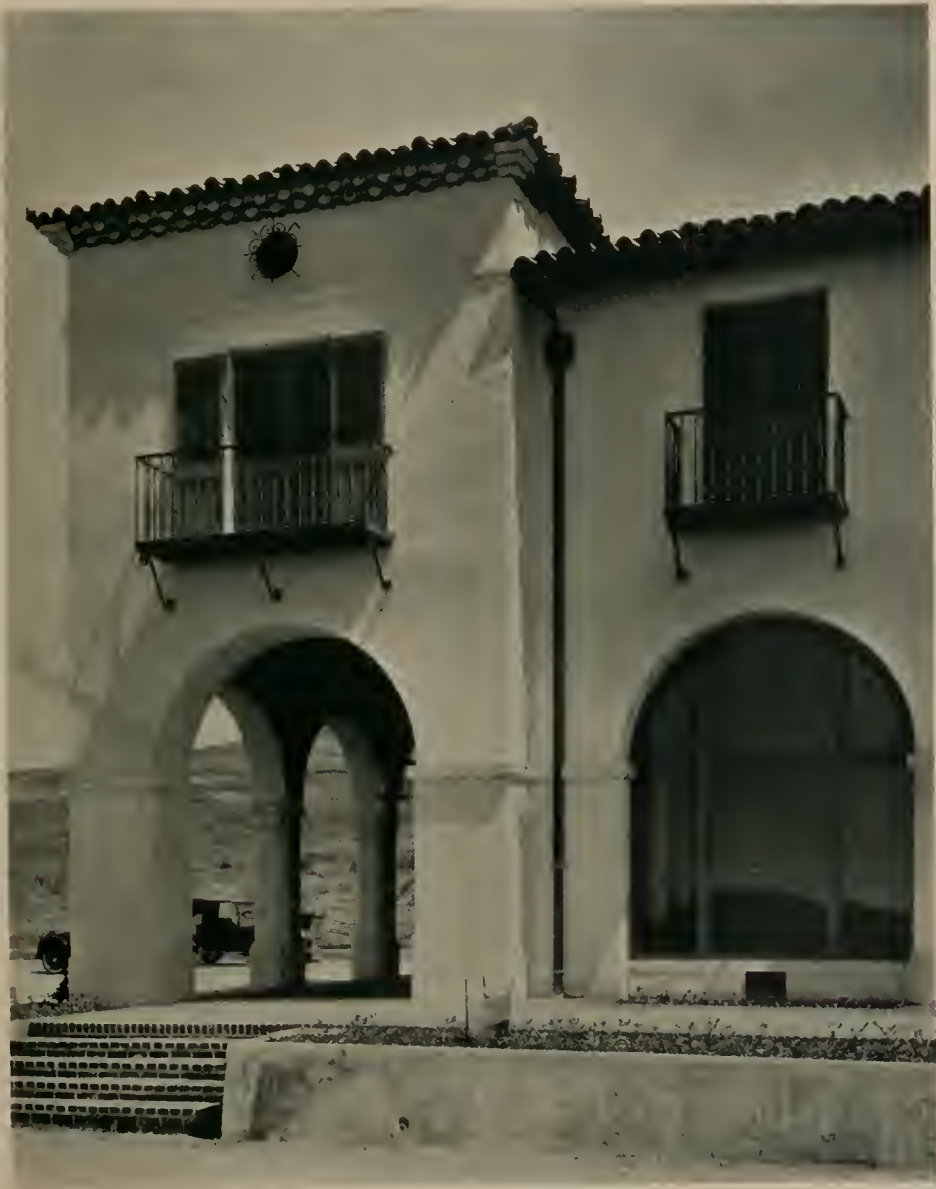
END PAVILION, MALAGA PLAZA STORES—PALOS VERDES, CALIFORNIA WEBBER, STAUNTON & SPAULDING, ARCHITECTS
