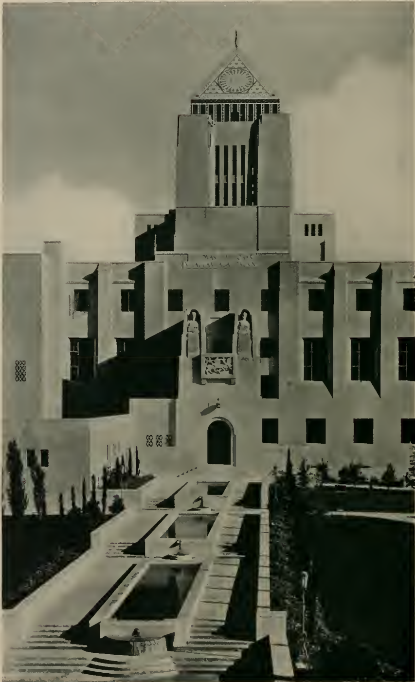
LOS ANGELES PUBLIC LIBRARY, LOS ANGELES, CALIFORNIA
