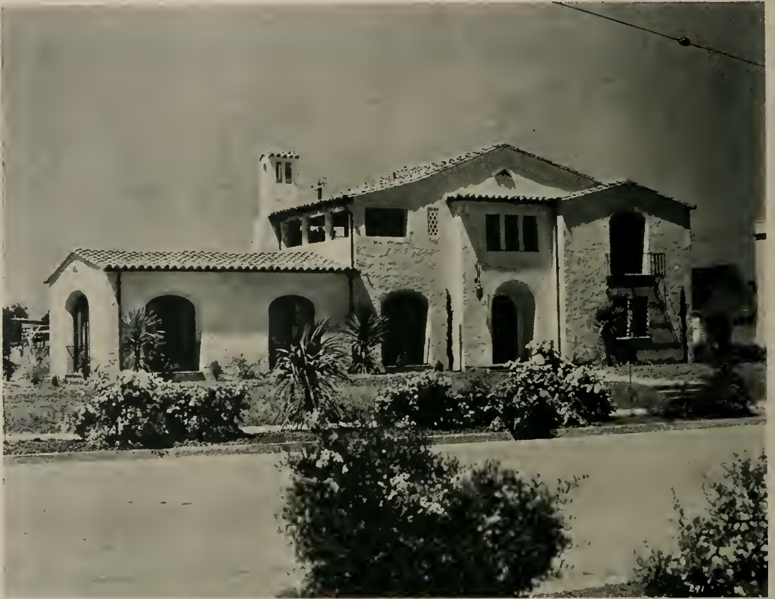
Burt L. Davis House, Crescent Park, Palo Alto, Calif.
