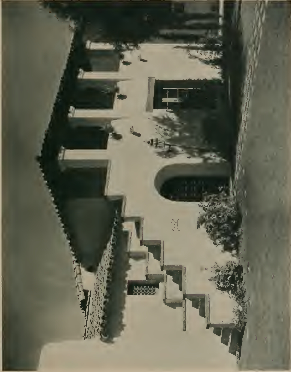
ENTRANCE DETAIL. RESIDENCE IN BEVERLY HILLS, CALIFORNIA. DESIGNED BY DAVID MALCOLM MASON
