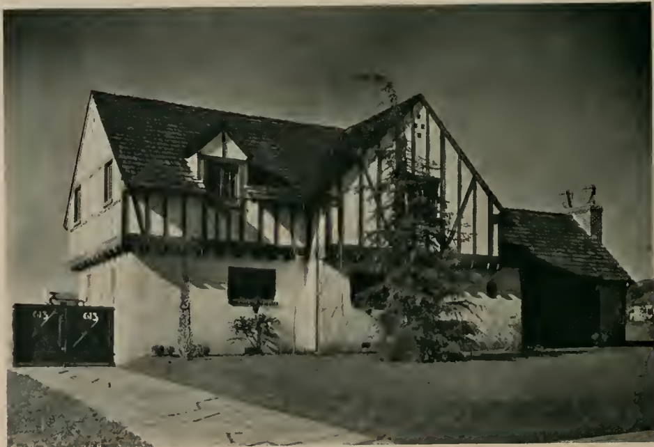
RESIDENCE FOR MR. CHARLES CARPENTER, LOS ANGELES, CALIFORNIA DESIGNED BY DAVID MALCOLM MASON
