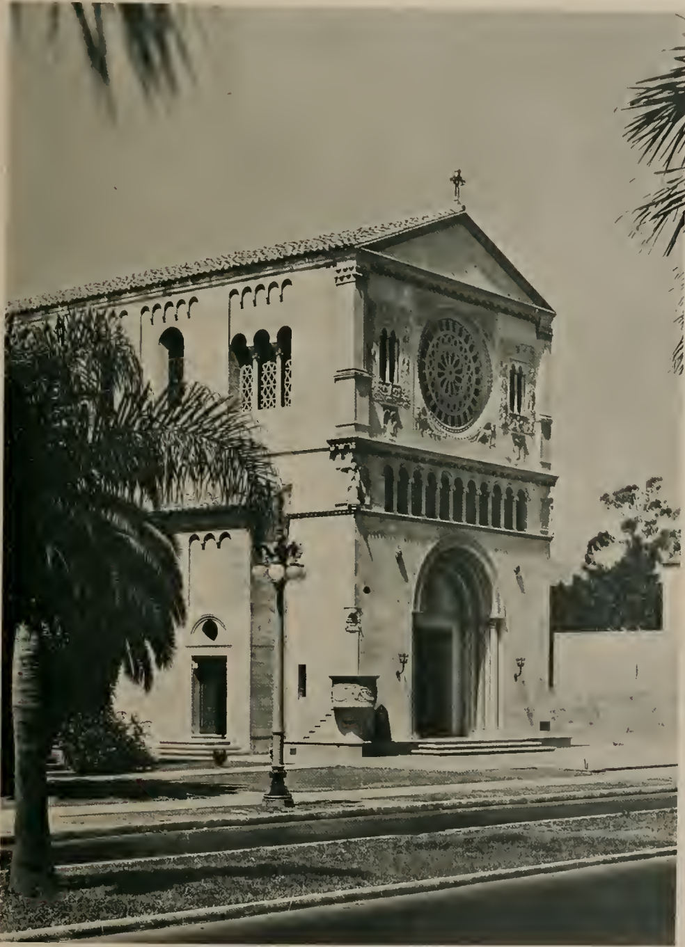
ST. JOHN'S CHURCH, LOS ANGELES PIERPONT AND WALTER S. DAVIS, ARCHITECTS
