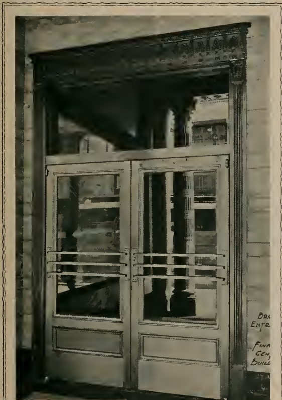
Bronze Entrance, Financial Center Building, Los Angeles, Calif. Norton & Wallis, Architects. Edwards, Wildley & Dixon, Contractors
