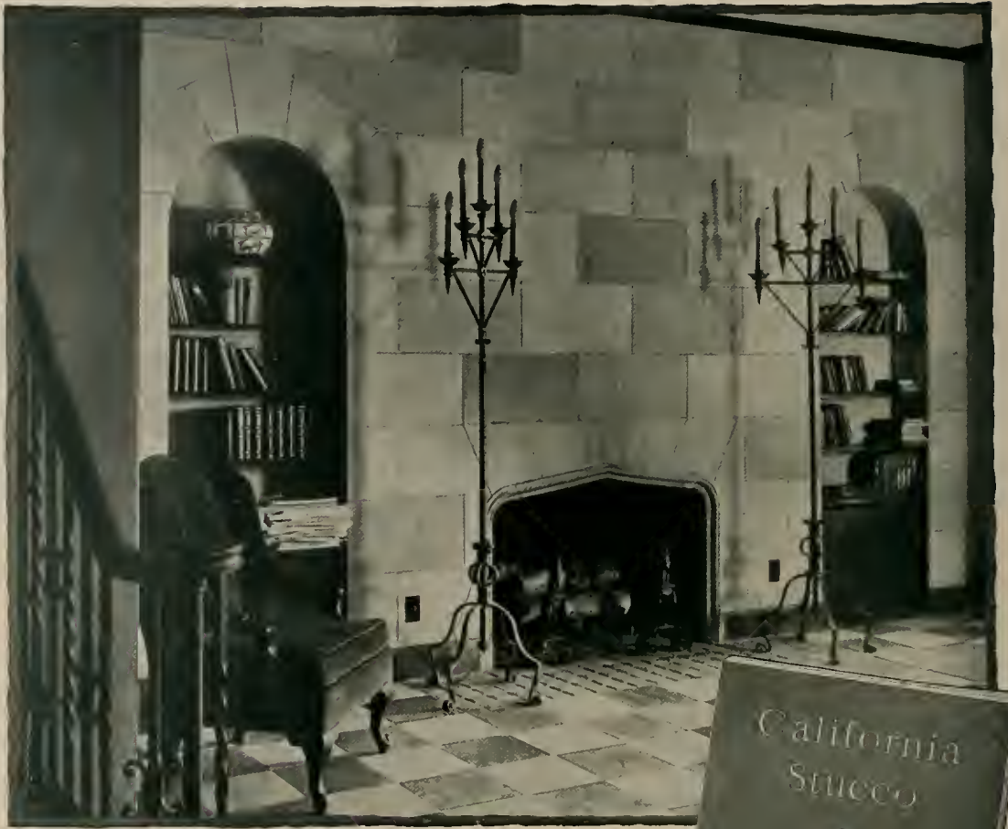
California Stucco in French Caen Stone Texture was used in the Lobby of Bladell Arms, Los Angeles
