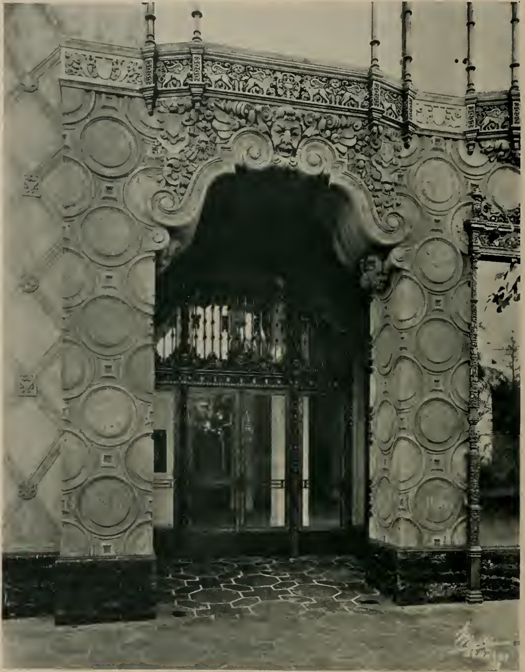
DETAIL OF OFFICE ENTRANCE, EL CAPITAN THEATRE, HOLLYWOOD, CALIFORNIA MORGAN, WALLS AND CLEMENTS, ARCHITECTS
