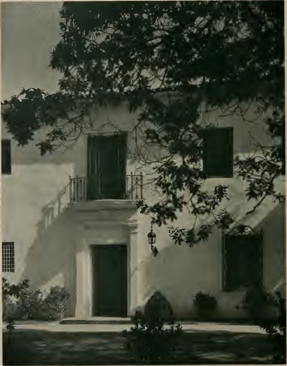
ENTRANCE DETAIL, RESIDENCE OF MR. JACQUES VINMONT, LOS ANGELES, CALIF. ROLAND E. COATE, ARCHITECT
