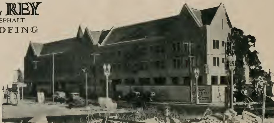
Melrose Hotel, recently completed at Los Angeles. S. Charles Lee was the Architect and Troyer Brothers, the builders. El Rey Slate Shingles were used on the slanting sections of the roof and El Rey Rolled Roofing on the flat surfaces.
