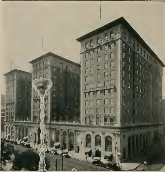
(The Biltmore, Los Angeles, illuminates its guest rooms with Duplex-a-lites...Schultze & Weaver, Architects)
