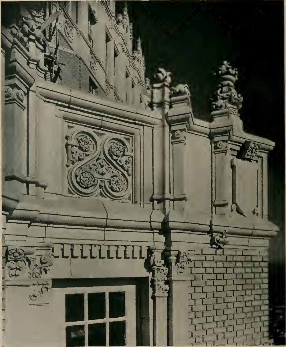
DETAIL OF PARAPET, 15TH FLOOR, HOTEL MARK HOPKINS, SAN FRANCISCO, CALIF. WEEKS & DAY, ARCHITECTS
