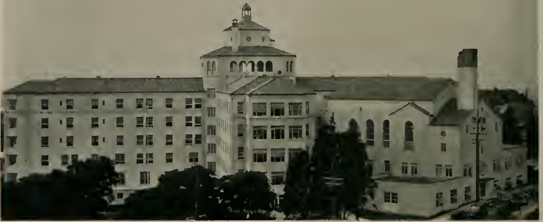
PROVIDENCE HOSPITAL, OAKLAND, CALIFORNIA
