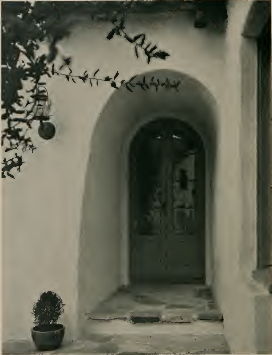
ENTRANCE DETAIL, RESIDENCE IN PASADENA, CALIFORNIA. DESIGNED BY HAROLD J. BISSNER Photo by Hiller
