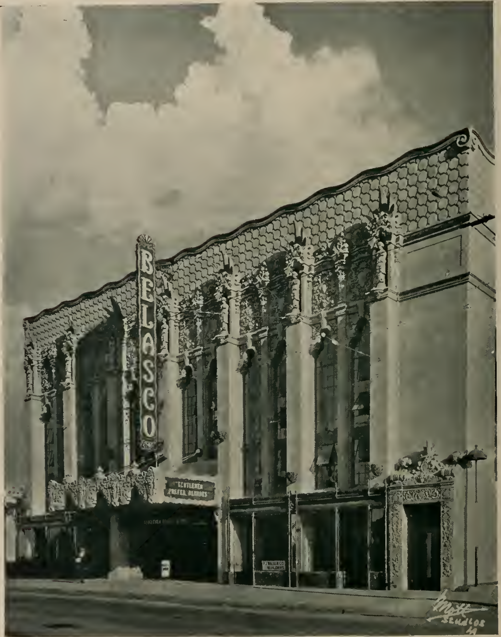
BELASCO THEATRE, LOS ANGELES, CALIFORNIA MORGAN, WALLS AND CLEMENTS, ARCHITECTS
