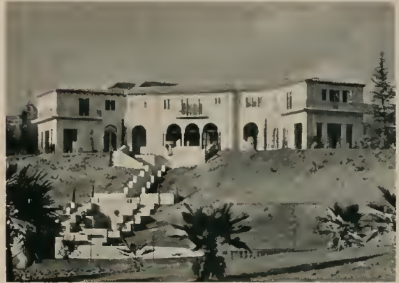
Buster Keaton Residence, Beverly Hills, California Gene Verge, Los Angeles, Architect
