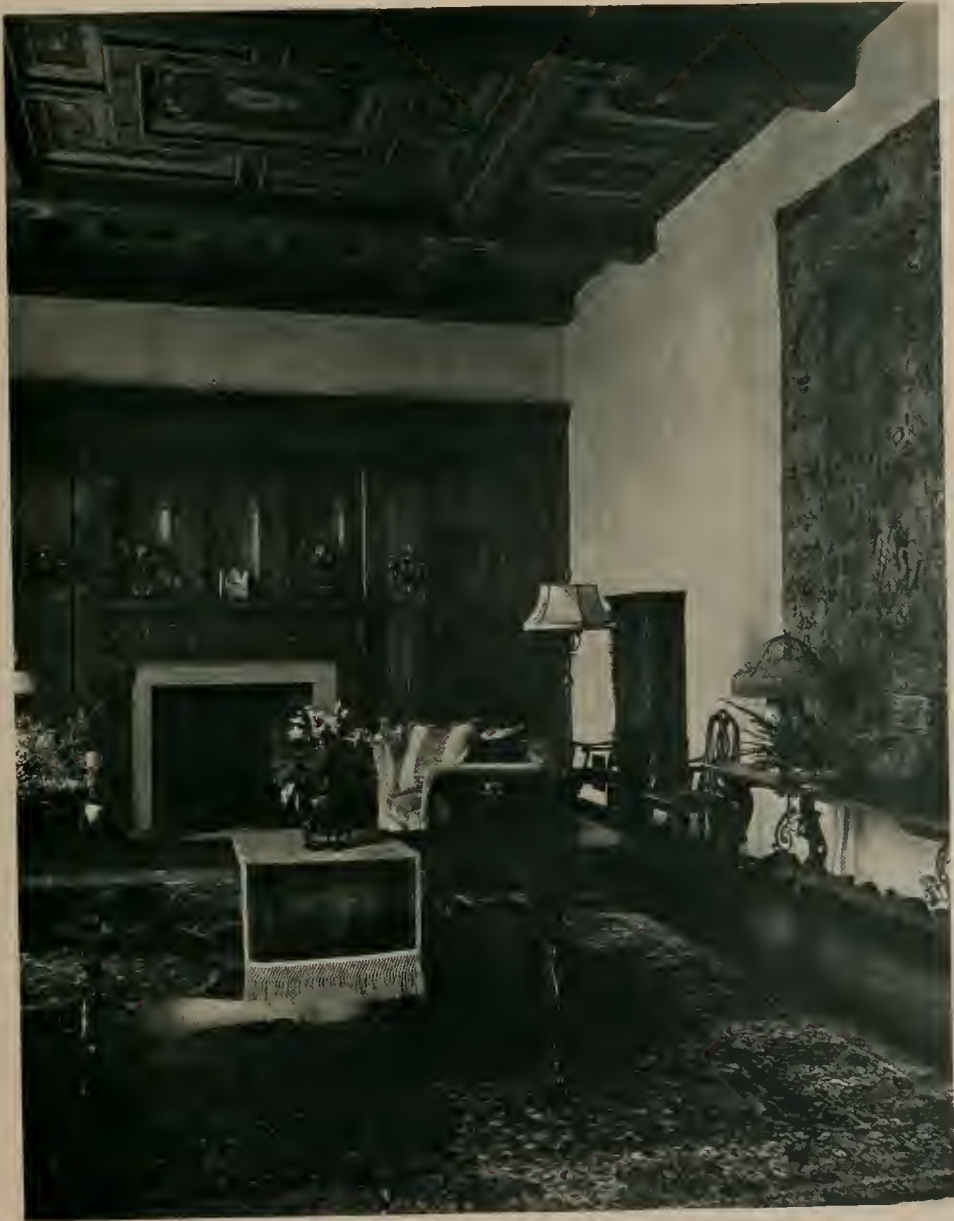
LIVING ROOM—RESIDENCE FOR MR. BENJ. R. MEYER, BEVERLY HILLS, CALIFORNIA GORDON B. KAUFMANN, ARCHITECT
