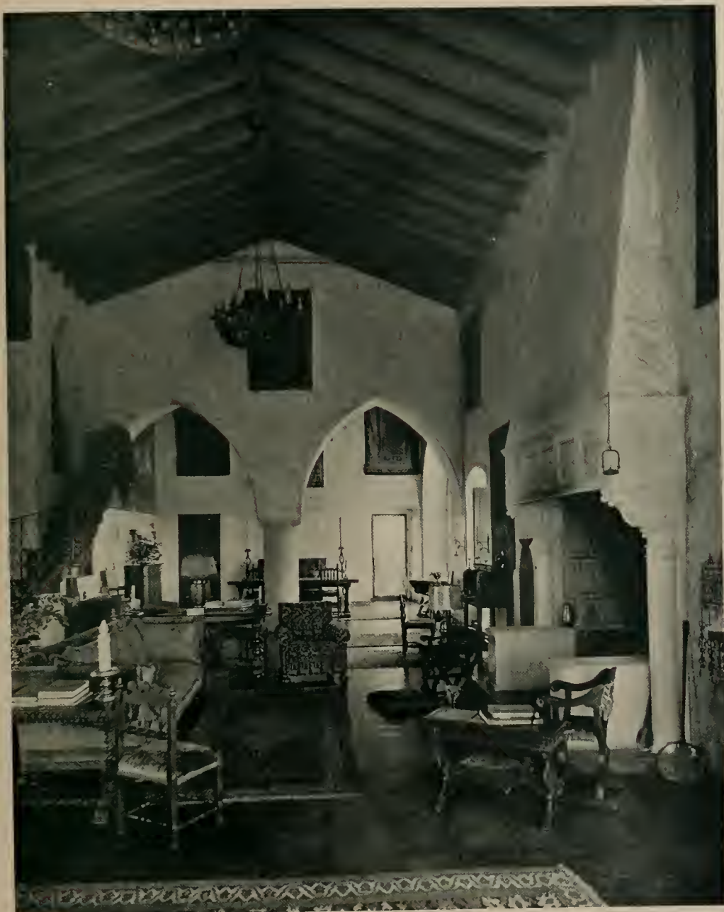
LIVING-ROOM—TOWARD DINING-ROOM, RESIDENCE OF MR. GARFIELD D. MERNER, HILLSBOROUGH, CALIF. WILLIS POLK & CO., ARCHITECTS
