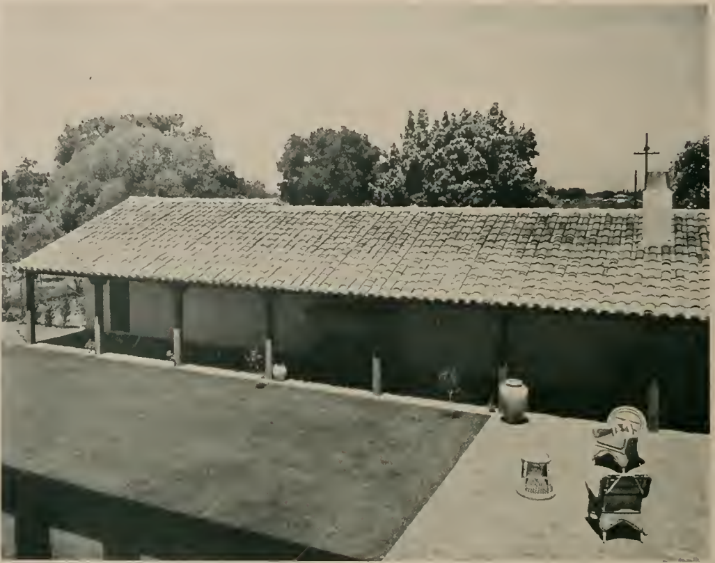
John A. Dunker Home, Palo Alto, Calif. Wells P. Goodenough, General Contractor. Birge M. Clark, Architect
