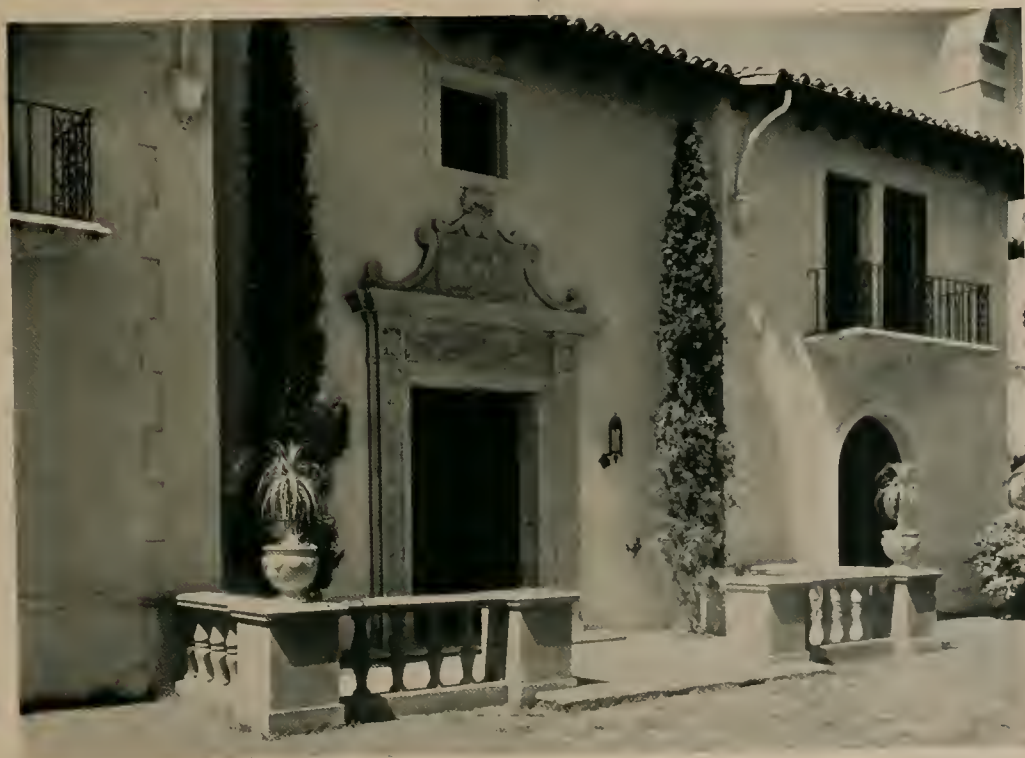
RESIDENCE OF MRS. CHARLOTTE PICKFORD, BEVERLY HILLS, CALIFORNIA WALLACE NEFF, ARCHITECT
