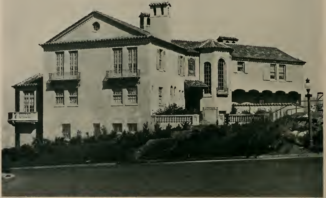
Howard Brickell Residence, Seacliff, San Francisco.
