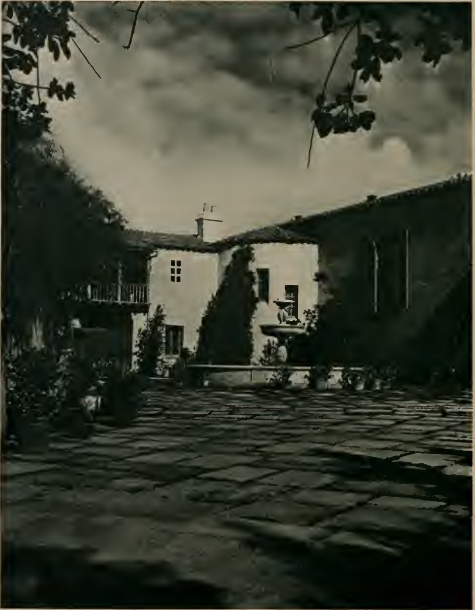
COURT—RESIDENCE FOR MR. BENJ. R. MEYER, BEVERLY HILLS, CALIFORNIA GORDON B. KAUFMANN, ARCHITECT
