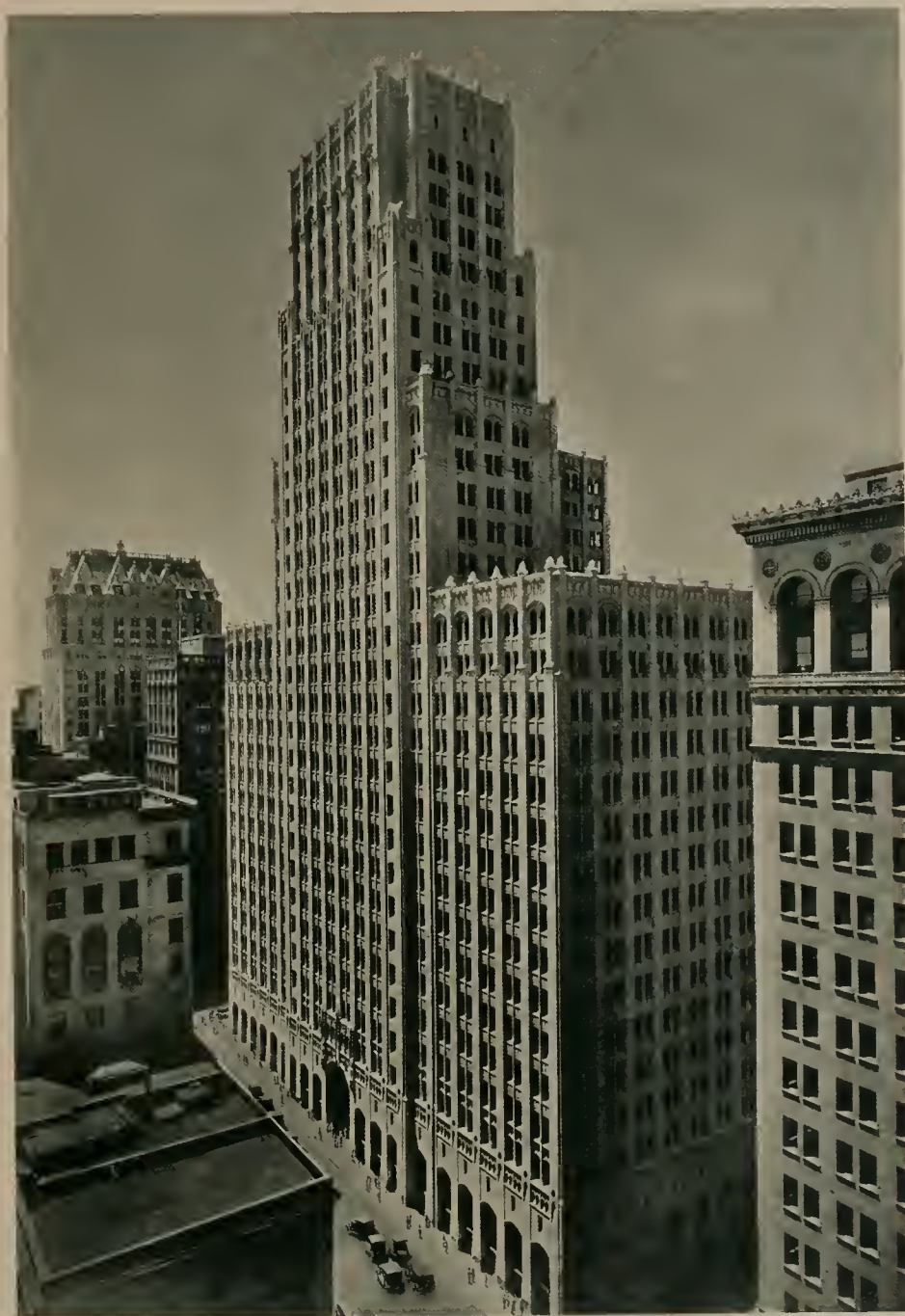
RUSS BUILDING, SAN FRANCISCO, CALIFORNIA. GEORGE W. KELHAM, ARCHITECT
