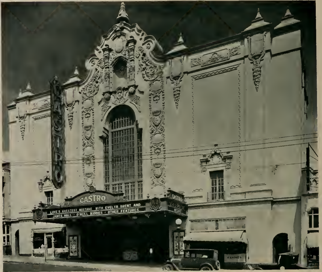
CASTRO THEATRE, SAN FRANCISCO, CALIFORNIA MILLER AND PELUEGER, ARCHITECTS
