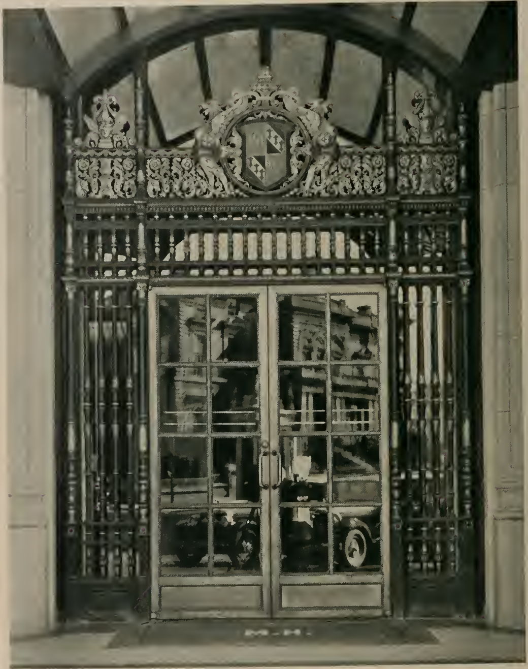
ENTRANCE, HOTEL MARK HOPKINS, SAN FRANCISCO, CALIFORNIA. WEEKS AND DAY, ARCHITECTS Executed by Michel & Pfeffer
