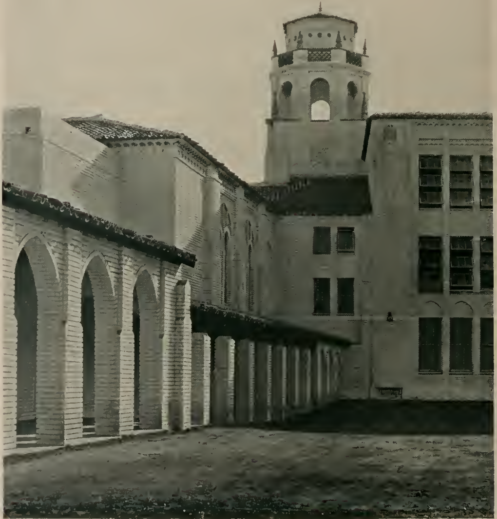
AUDITORIUM WING FROM PLAYGROUND, W. P. FRICK SCHOOL, OAKLAND, CALIFORNIA WYTHE, BLAINE AND OLSEN, ARCHITECTS
