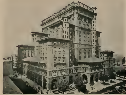
HOTEL VANCOUVER, Vancouver, B. C. R. T. Garrow, Architect J. S. Christy, General Contractor
