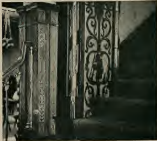
Pilaster of sand-etched Douglas Fir on stairway of Hotel Emerson. This design has the early pioneer hunter of the Pacific Northwest for a motif.
