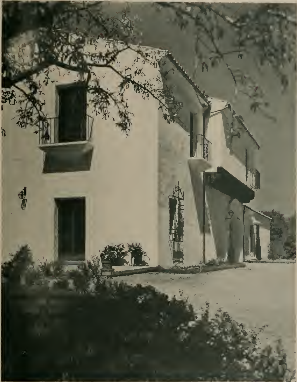
RESIDENCE OF COL. D. C. JACKLING, WOODSIDE, CALIF. GEORGE WASHINGTON SMITH, ARCHITECT
