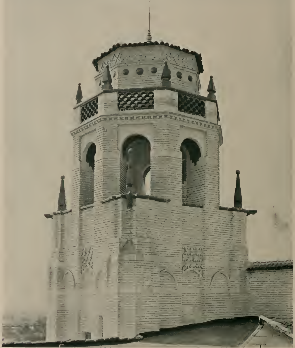
TOWER DETAIL, W. P. FRICK SCHOOL, OAKLAND, CALIFORNIA WYTHE, BLAINE AND OLSEN, ARCHITECTS
