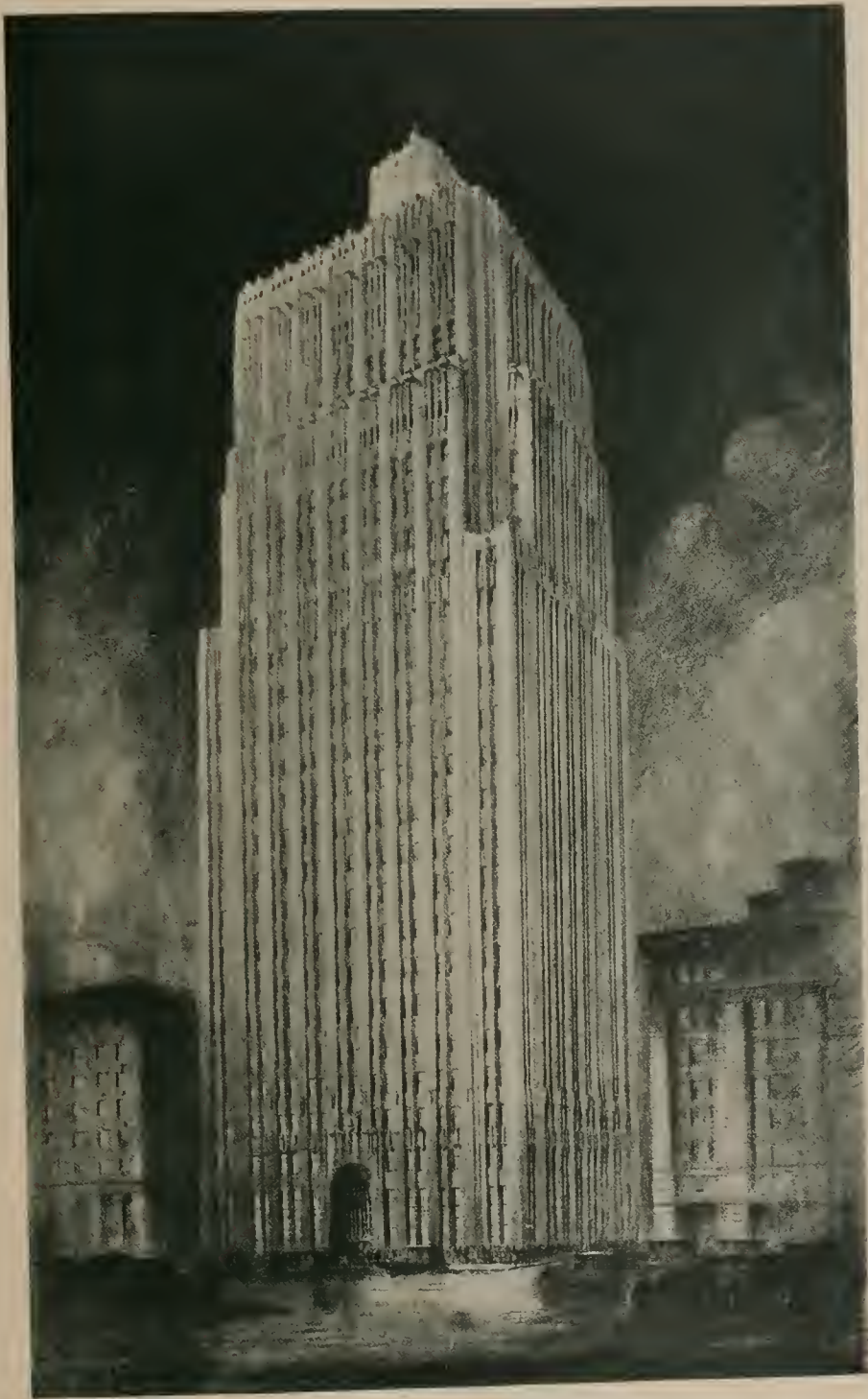
COAST DIVISION BUILDING, PACIFIC TELEPHONE & TELEGRAPH CO., SAN FRANCISCO MILLER AND PFLUEGER, ARCHITECTS; A. A. CANTIN, ASSOCIATE
