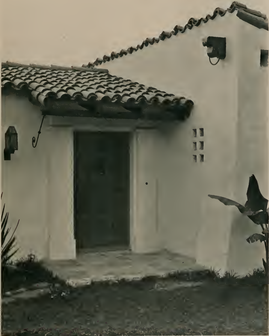
ENTRANCE DETAIL, RESIDENCE IN PASADENA, CALIFORNIA. DESIGNED BY HAROLD J. BISSNER
