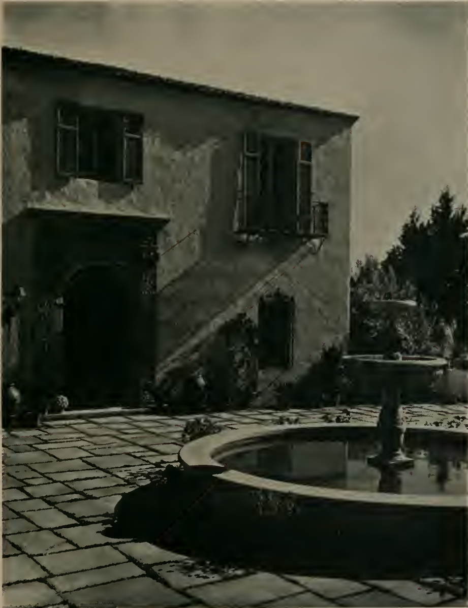
ENTRANCE DETAIL—RESIDENCE FOR MR. BENJ. R. MEYER, BEVERLY HILLS, CALIFORNIA GORDON B. KAUFMANN, ARCHITECT
