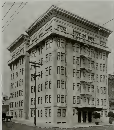
MCKENZIE BUILDING, SAN FRANCISCO R. W. Moller, Architect—Glidden's Liquid Cement on Exterior, Applied 1913.
