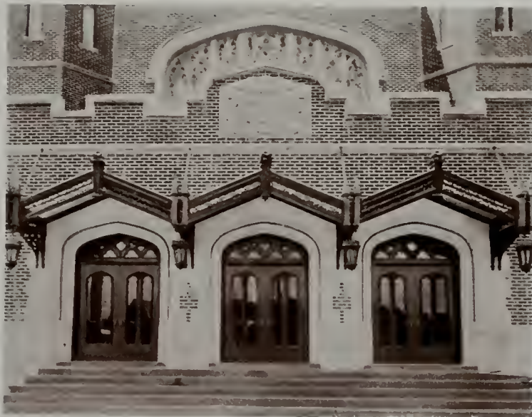
MAIN ENTRANCE DETAIL LINCOLN PARK HIGH SCHOOL, TACOMA, HEATH & GOVE, ARCHITECTS
