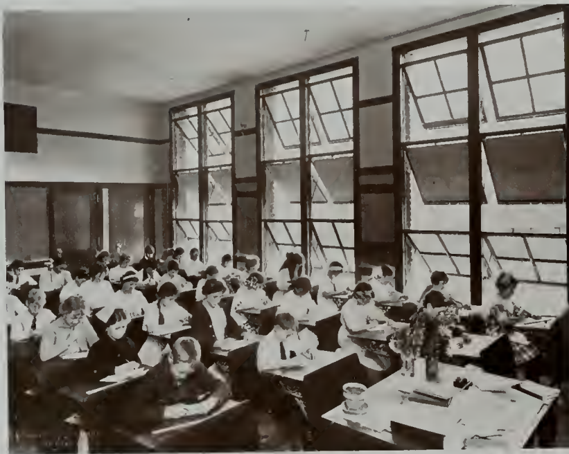
TYPICAL INTERIOR VIEW OF CLASS ROOMS, OAKLAND SCHOOLS
