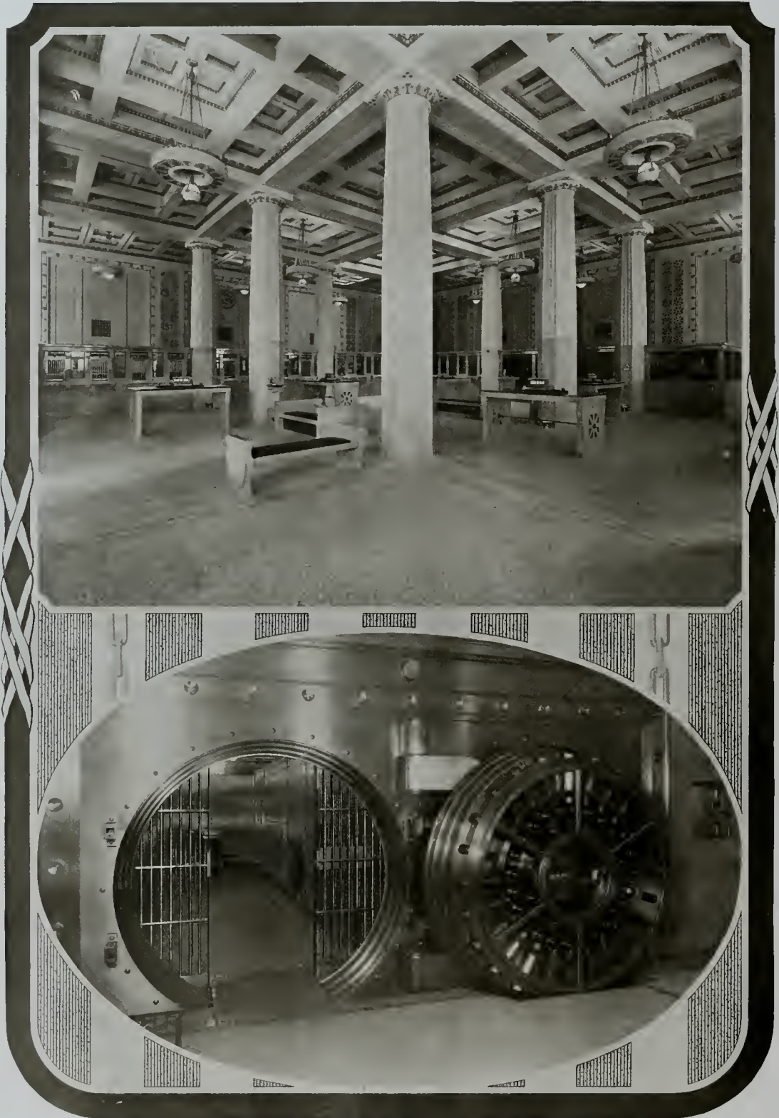
GENERAL VIEW INTERIOR BANKING ROOM AND SAFE DEPOSIT VAULT DOOR CITIZENS NATIONAL BANK BUILDING, LOS ANGELES JOHN PARKINSON AND EDWIN BERGSTROM, ARCHITECTS
