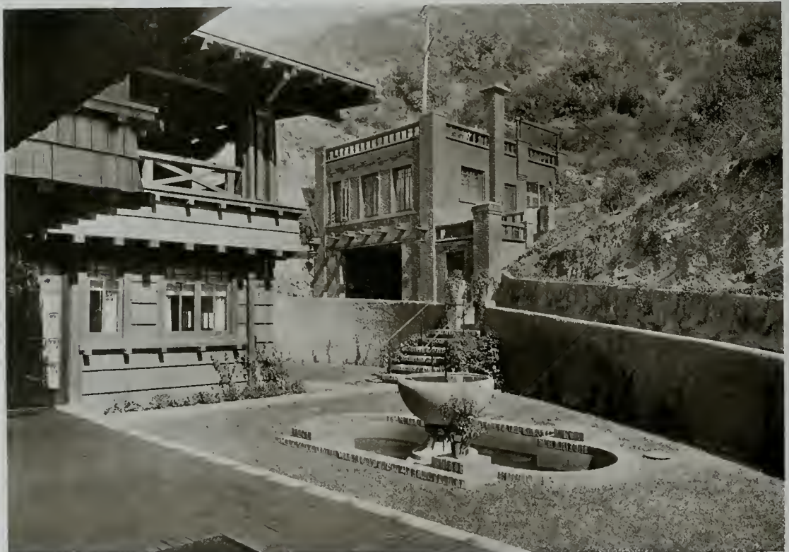
PATIO AND GARAGE F. E. ENGSTRUM RESIDENCE, ARTEMISIA, CANYON ROAD, HOLLYWOOD F. A. BROWN, ARCHITECT
