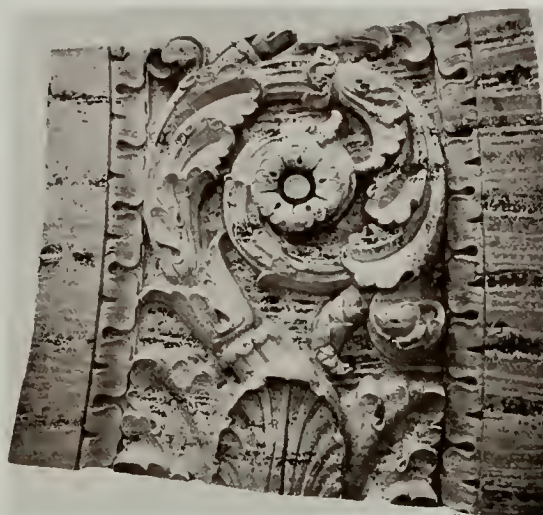
Cast Travertine, with Ornamentation.
