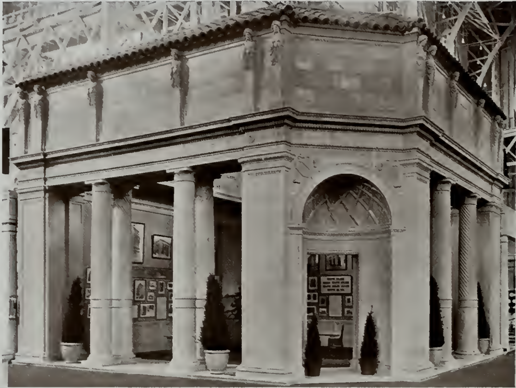
National Terra Cotta Society Building in Varied Industries Building
