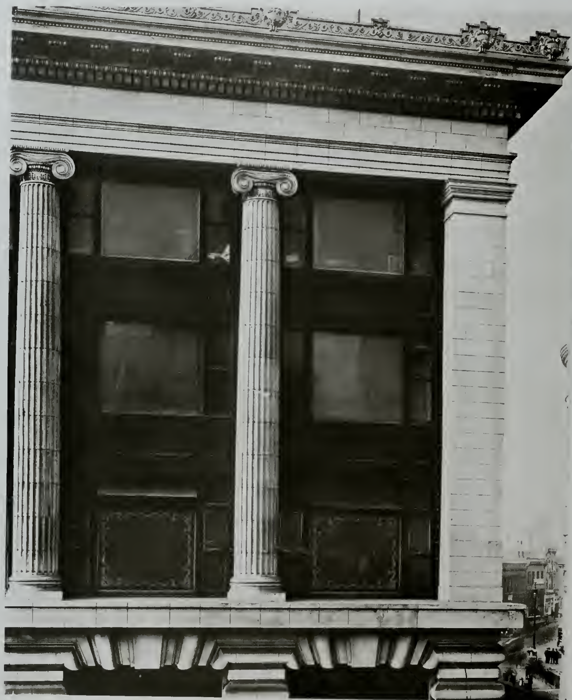
DETAIL OF UPPER STORIES HALE BROS. BUILDING, SAN FRANCISCO REID BROS., ARCHITECTS
