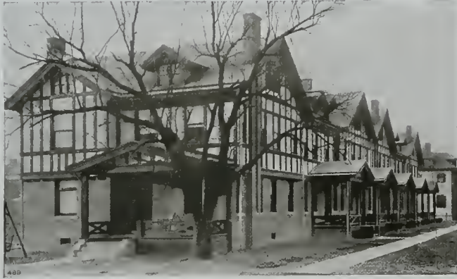
Flat Asbestos Building Lumber Used in Half Timber Effect on Residences Roofing of Asbestos Shingles
