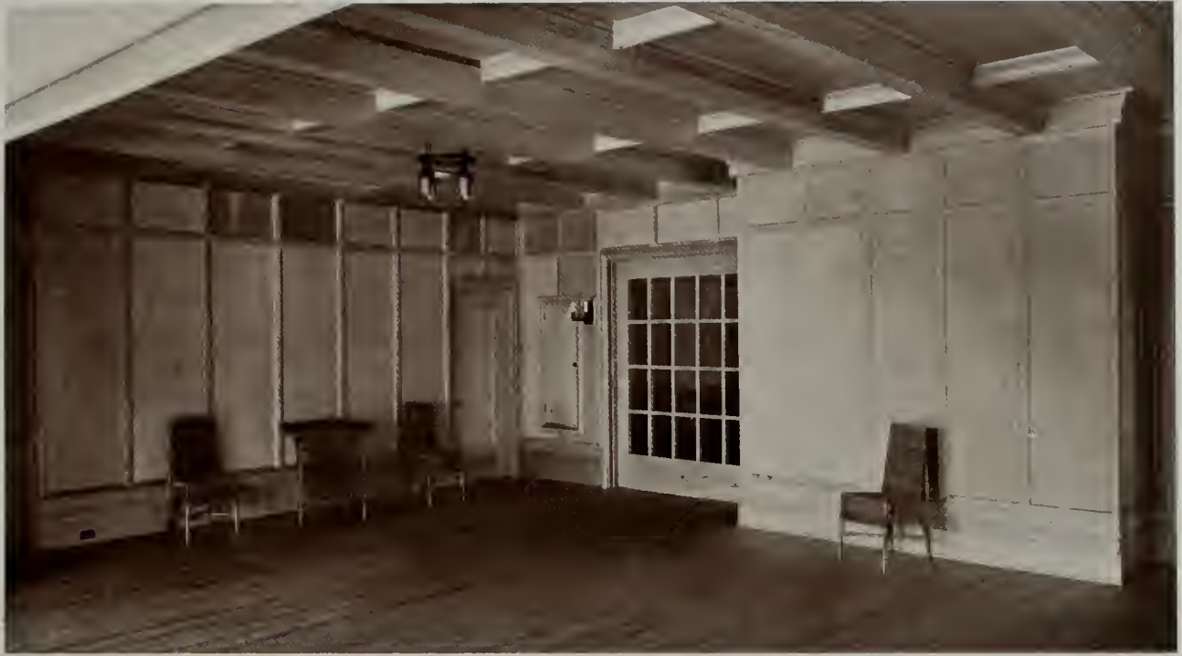
Interior View California White and Sugar Pine Industries Building, showing Wall Panels
