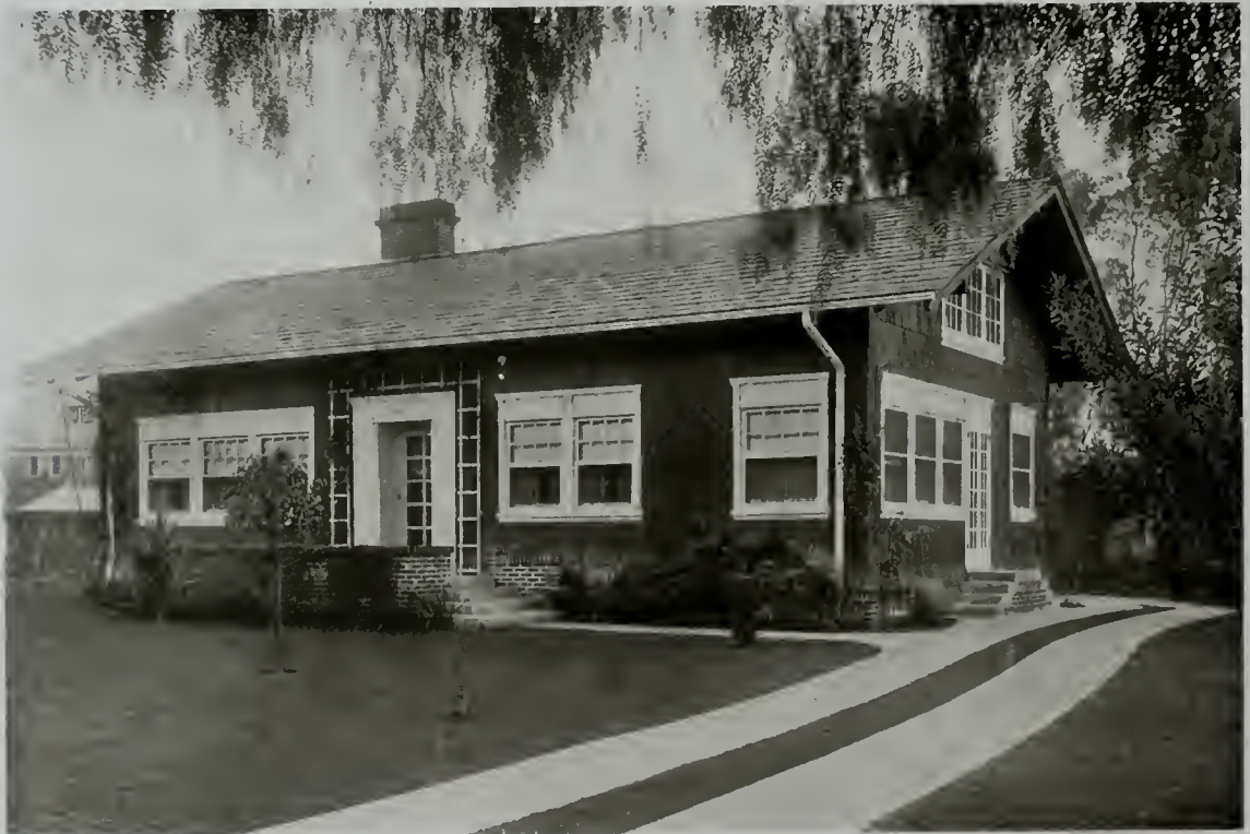
Plate No. 8 There is a reticence expressed in the design of this bungalow that would lead one to think that the owner or architect was not fully in sympathy with the bungalow movement. To escape the approbrium of the class, a delicate colonial door and window treatment could not be foregone though somewhat at variance with rough shakes. The effect of shakes cut to the size of shingles is a compromise. Notwithstanding all this, it is a successful design.
