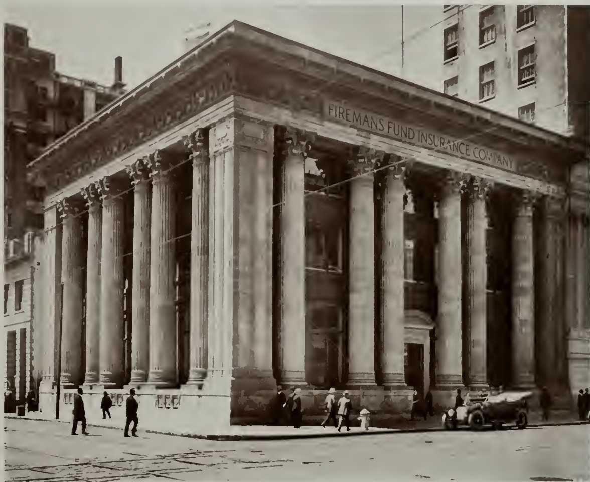
FIREMAN'S FUND INSURANCE COMPANY BUILDING San Francisco
