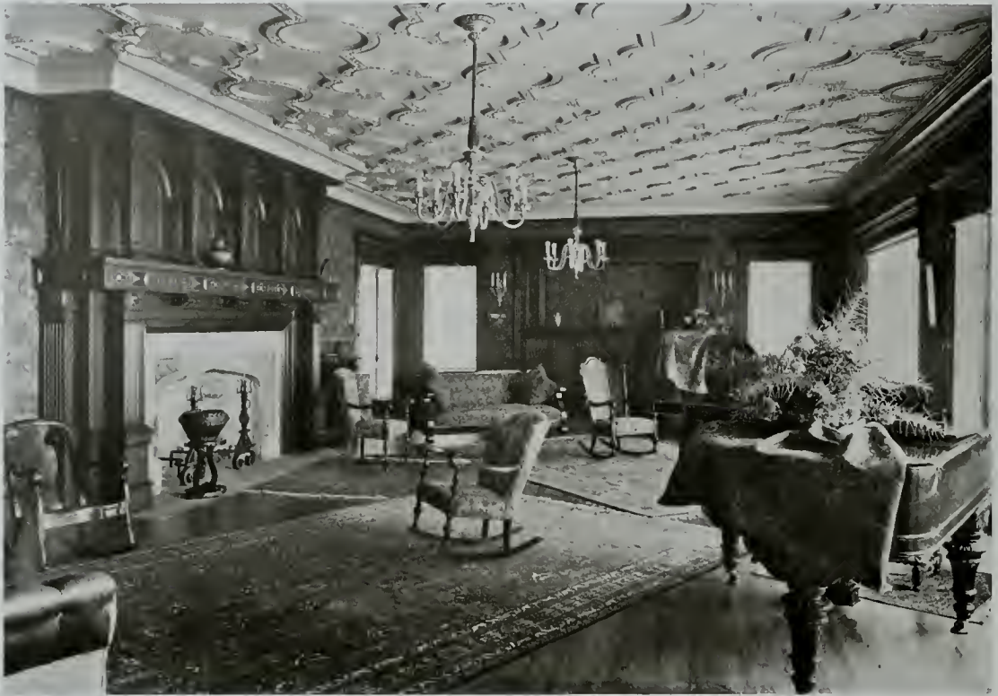
LIVING ROOM SHOWING VIEW OF MANTLE
