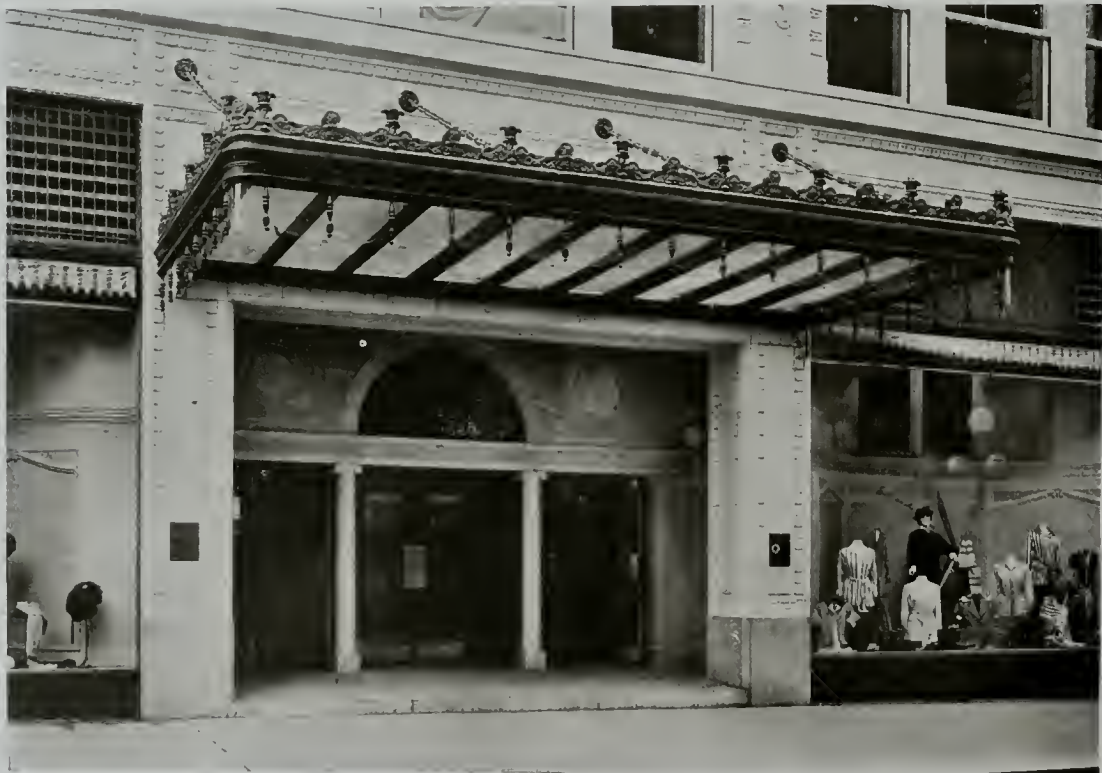
FIFTH STREET ENTRANCE MEIER & FRANK COMPANY DEPARTMENT STORE, PORTLAND DOYLE & PATTERSON, ARCHITECTS
