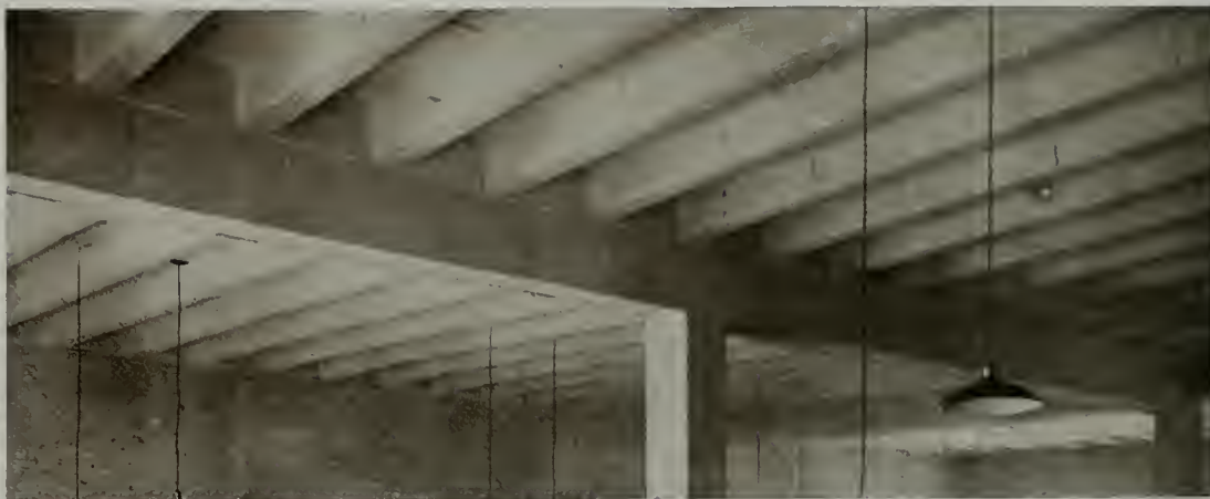
Open Ceiling Construction Resulting from use of Meyer System Metal Forms.
