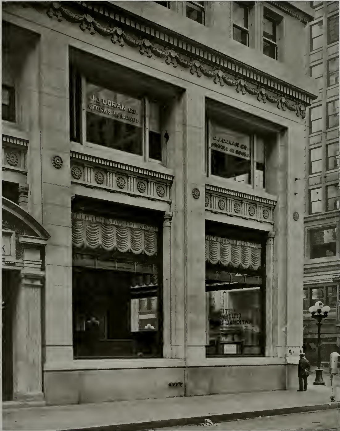
DETAIL OF FIRST AND SECOND STORIES CITIZENS NATIONAL BANK BUILDING, LOS ANGELES JOHN PARKINSON AND EDWIN BERGSTROM, ARCHITECTS
