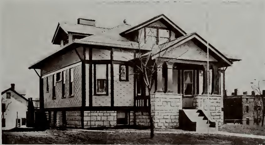
W. E. Crawford Residence, Cincinnati, Ohio. Fasse and Reed Architects. Asbestos "Century" Shingles applied French Method on the Roof and Honeycomb Effect on the Sides.
