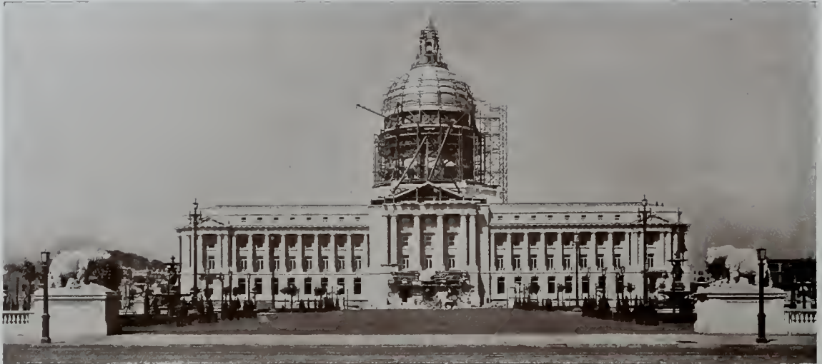
CUT SHOWS PROGRESS ON NEW CITY HALL, SAN FRANCISCO, BAKEWELL & BROWN, ARCHITECTS
