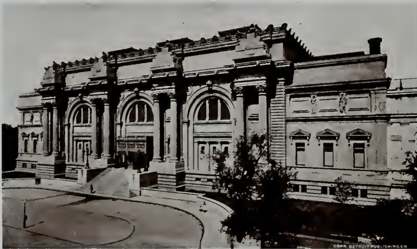
Metropolitan Museum of Art, New York City Covered with "Target and Arrow" Roofing Tin
