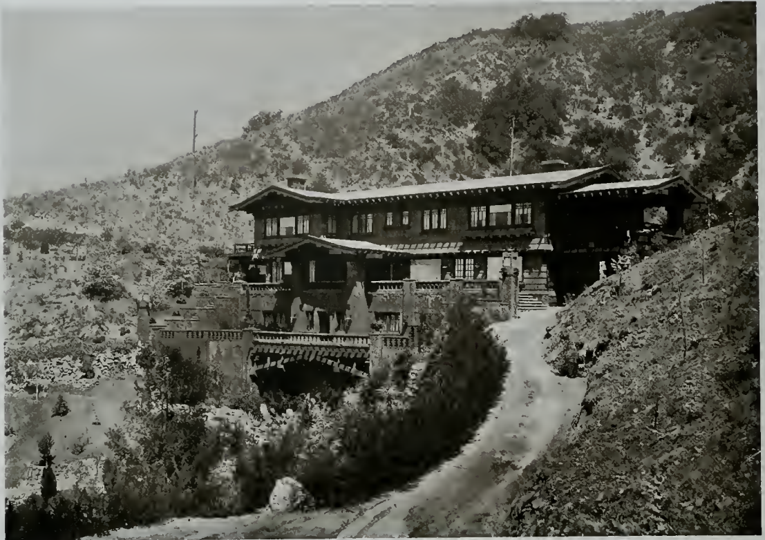
VIEW FROM DRIVEWAY
