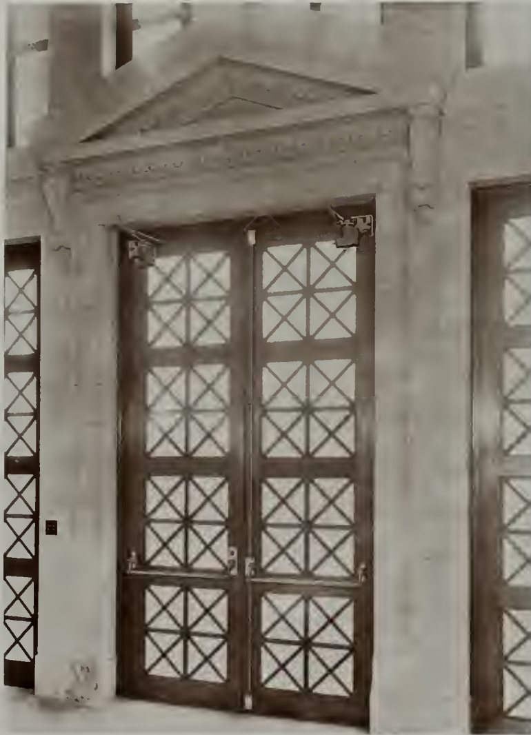
INTERIOR DETAIL OF DOORWAY IN OAKLAND TECHNICAL HIGH SCHOOL SHOWING THE APPLICATION OF RUSSWIN PANIC-EXIT BOLTS, FURNISHED THROUGH THE MAXWELL HARDWARE COMPANY
