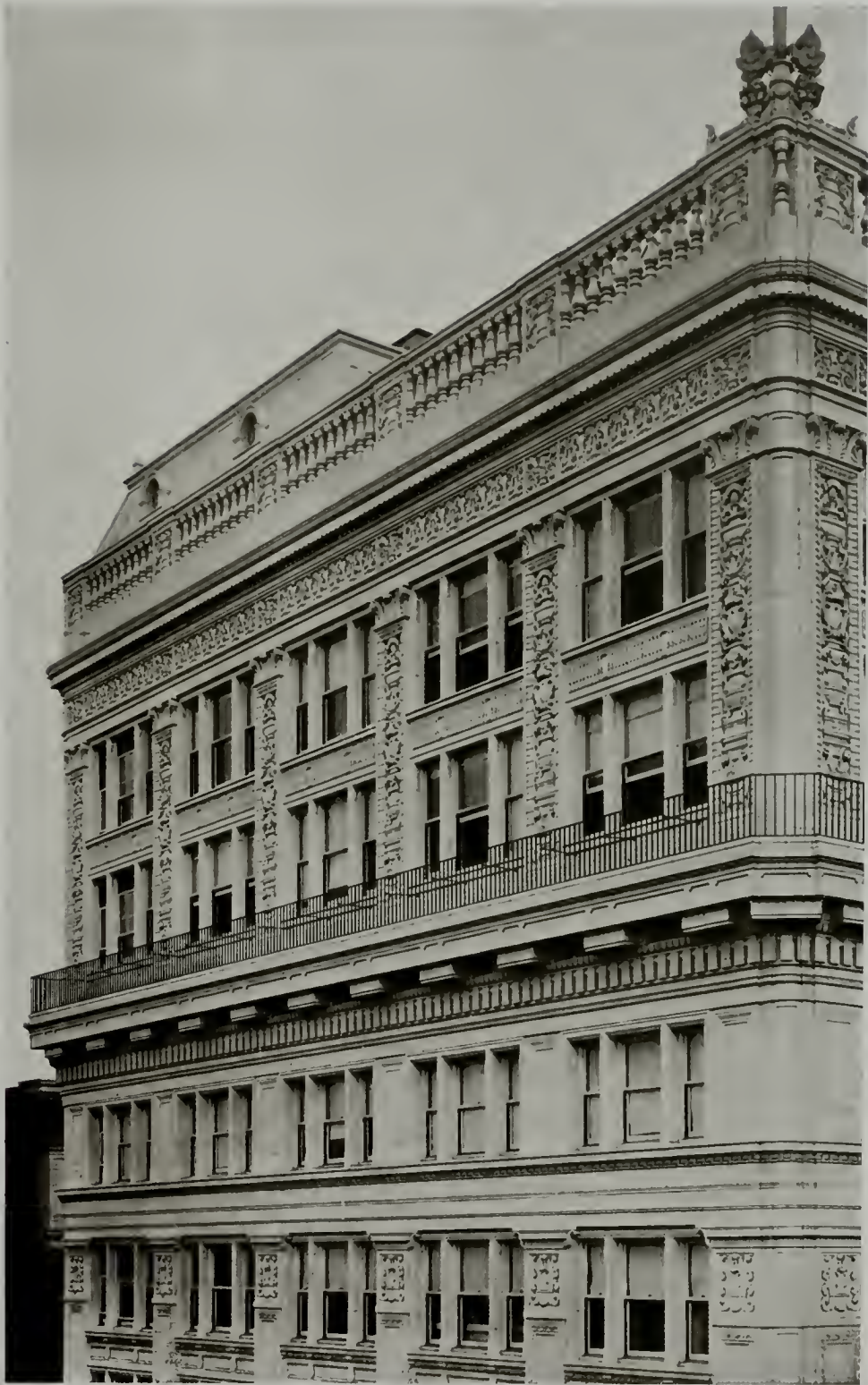
UPPER STORIES MEIER & FRANK COMPANY DEPARTMENT STORE, PORTLAND DOYLE & PATTERSON, ARCHITECTS
