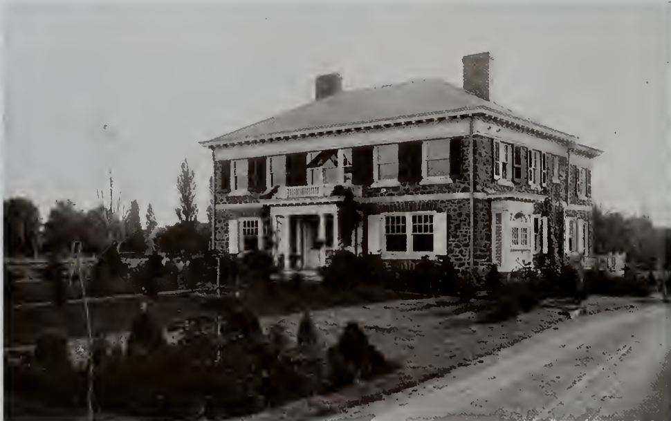
E. W. Twaddle Residence, Devon, Pa. Asbestos "Century" Shingles applied French Method on the Roof
