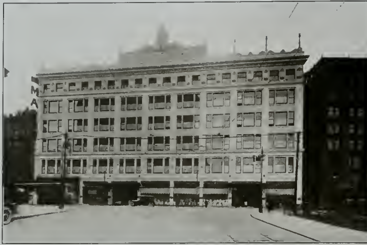
Meyer System Floor Construction MAY CO. DEPARTMENT STORE, CLEVELAND, OHIO Graham, Burnham Co., Architects
