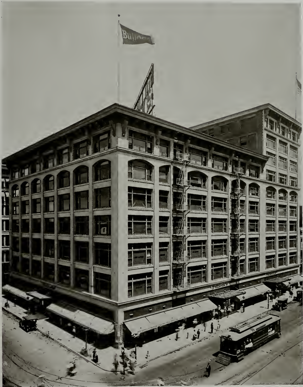
BULLOCK'S STORE, LOS ANGELES JOHN PARKINSON and EDWIN BERGSTROM, ARCHITECTS ROLLAND H. HESS, DESIGNER OF EQUIPMENT
