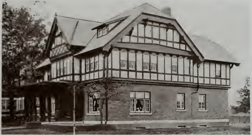
Francis Line Residence, Cleveland, Ohio. J. Milton Dyer and F. G. Bates, Architects. Asbestos "Century" Shingles applied American Method on the Roof and Asbestos Building Lumber on the Sides.
