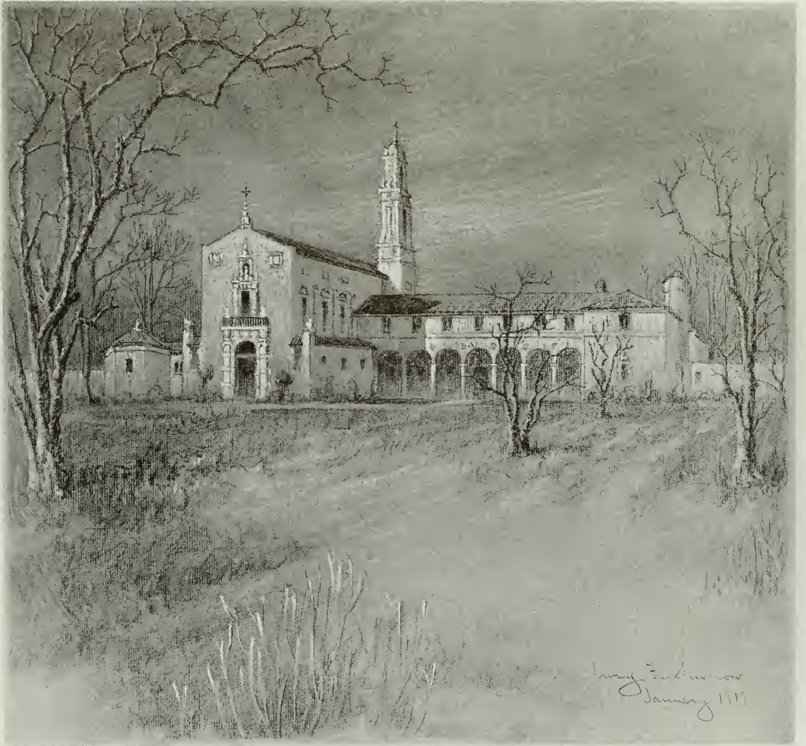
GENERAL VIEW FROM FRONT CARMELITE MONASTERY, SANTA CLARA, CAL. MAGINNIS & WALSH, Architects
