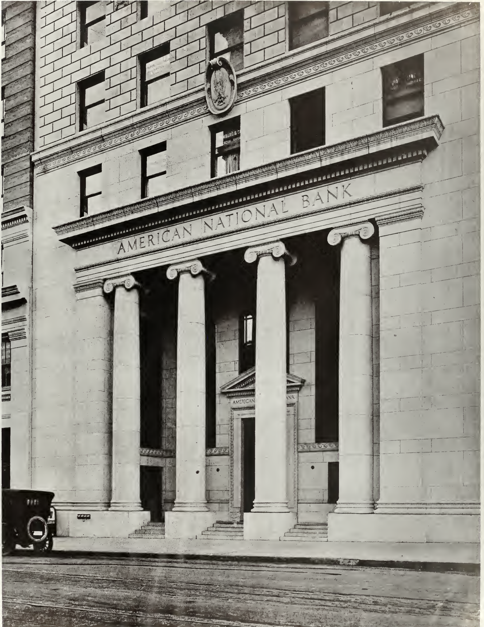
ENTRANCE DETAIL THE AMERICAN NATIONAL BANK BUILDING, SAN FRANCISCO GEORGE W. KELHAM, Architect
