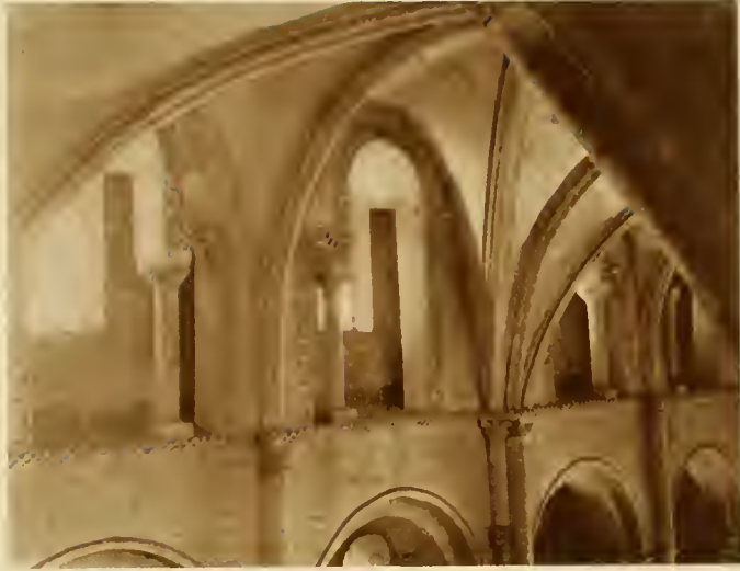
FIG. 61. S.-Etienne, Caen, (Calvados). Nave vaults.
