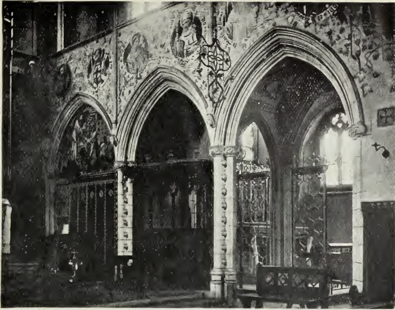
CHURCH OF THE HOLY ROOD, WATFORD: CHANCEL (PAINTED DECORATION).
