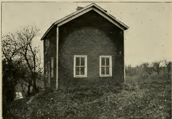
Fig. 71.—Shop (looking South).
