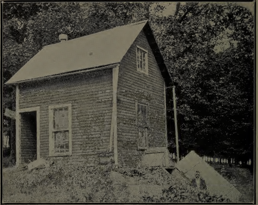
Fig. 56. A France outapiary house with cellar beneath which serves as winter cellar.
