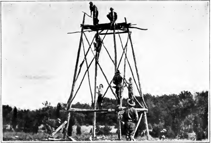
Building the Tower
