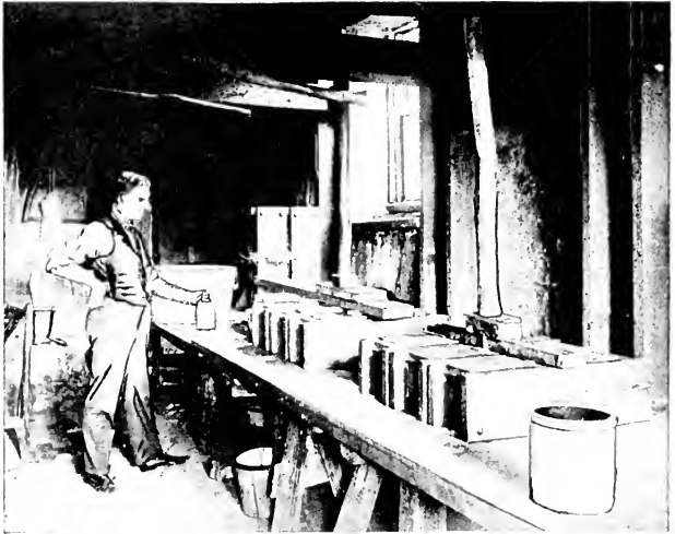
Block Swiss under pressure in individual molds.
