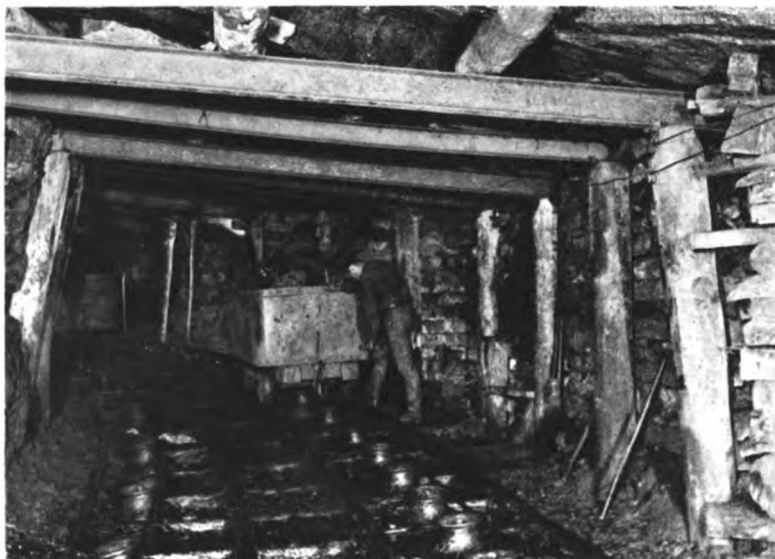
CURVE ON ENDLESS ROPE HAULAGE
