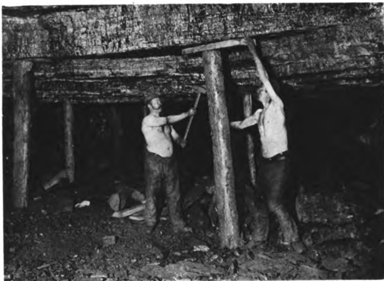
SETTING TIMBER PROPS
