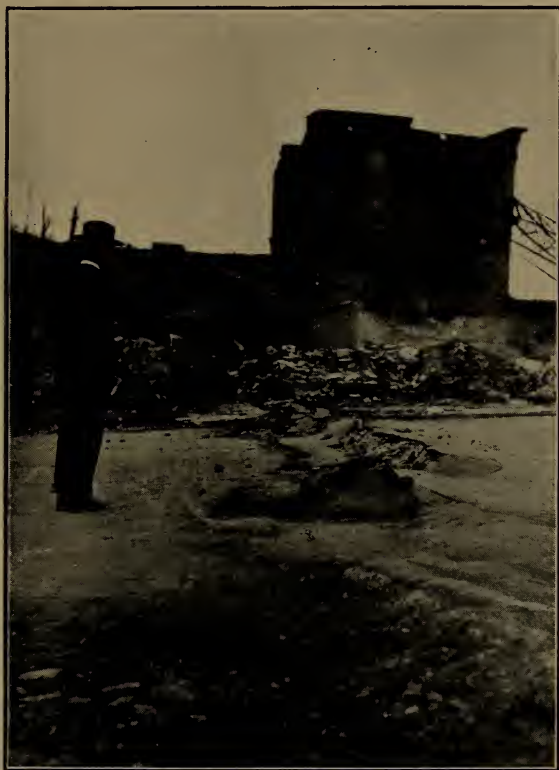
A Crack Across Van Ness Avenue.
