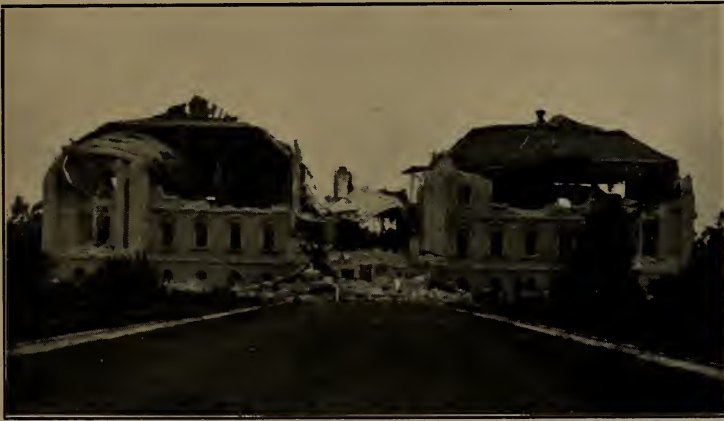
Ruined Buildings at Stanford University.
