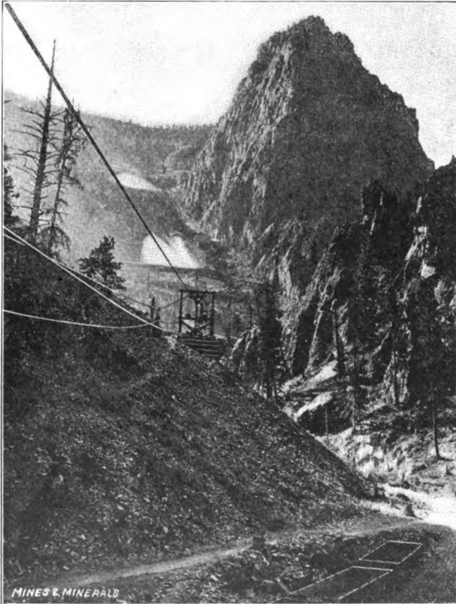
FIG. 157.—WIRE ROPE BUCKET TRAMWAY, CREEDE, COLO.
