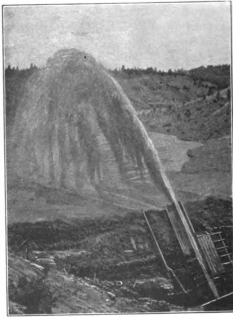
FIG. 114.—HYDRAULIC ELEVATOR, NORTH BLOOMFIELD, CALIFORNIA.
