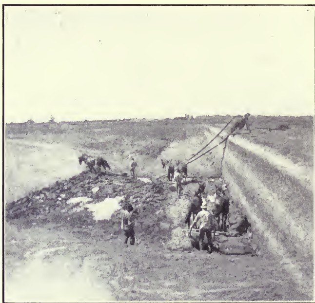
Fig. 56.—Stripping Coal by Scrapers.
