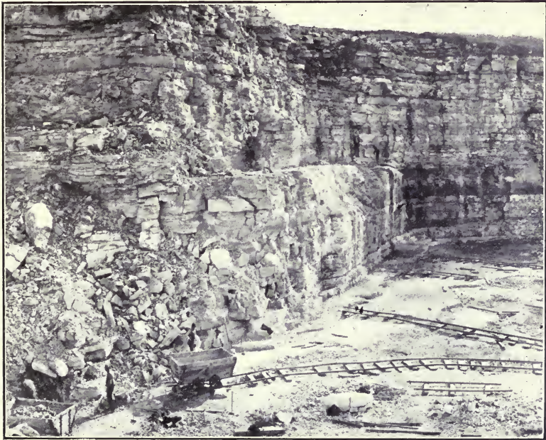
Fig. 54.— Quarry showing Bench before Blast.
