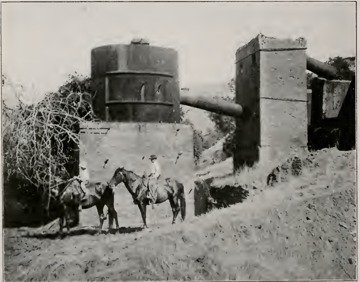
Photo No. 28. Old coarse-ore quicksilver furnace, erected 1873, at Keystone Mine, San Luis Obispo County Photo by E. W. Carson.
