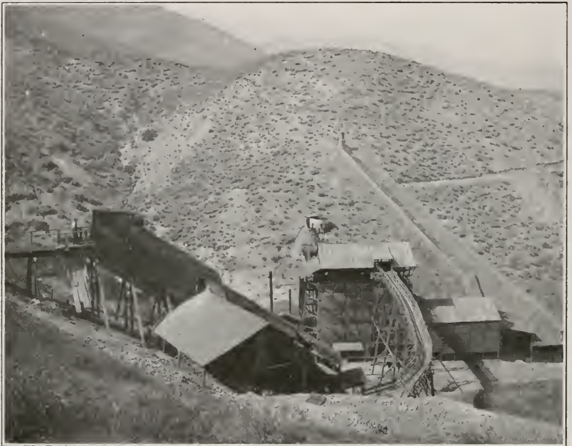
Photo No. 3. Furnace at New Mercy (Pacific) Quicksilver Mine, Fresno County.
