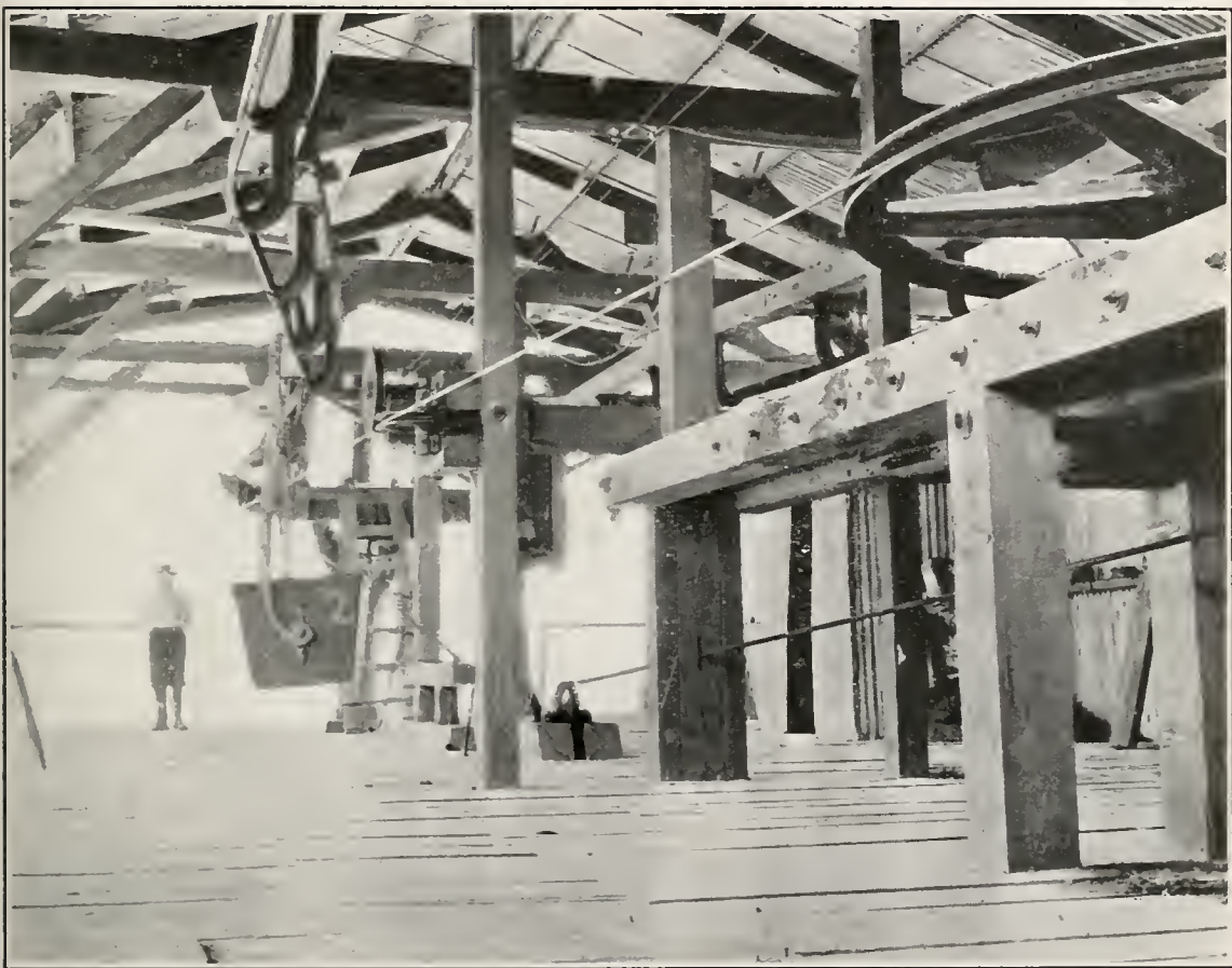
Photo No. 32. Tramway unloading terminal at Oceanic Mine.
