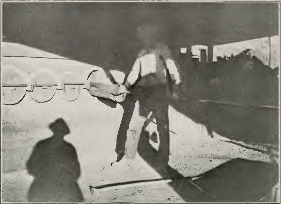
Photo No. 43. Charging a Johnson-McKay retort at the Patriquin Mine, Monterey County.
