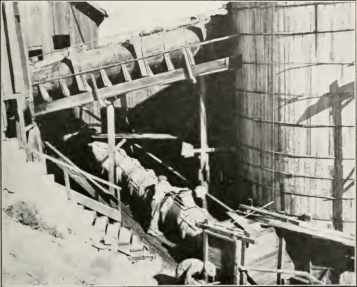
Photo No. 65. Condenser Flues—Vitrified Pipe (lower), and Wood-stave (upper),—at New Idria Mine, San Benito County.
