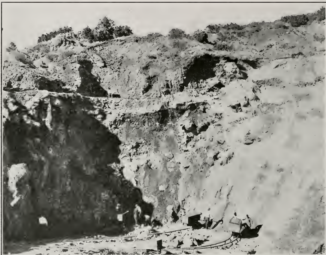
Photo No. 25. San Carlos Mine, open cut above No. 2 level. Recovering dump material and old pillars.
