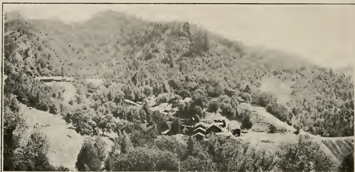
Photo No. 38. Great Eastern Mine, near Guerneville, Sonoma County. Ledge outcrop at left; furnaces in center; furnace dump at right.
