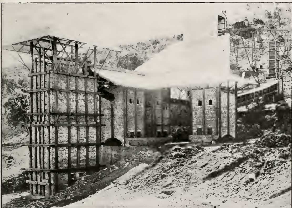
Photo No. 7. Ten-ton Scott fine-ore furnace and condensers, Kings Quicksilver Mining Company, Ltd., Kings County.
