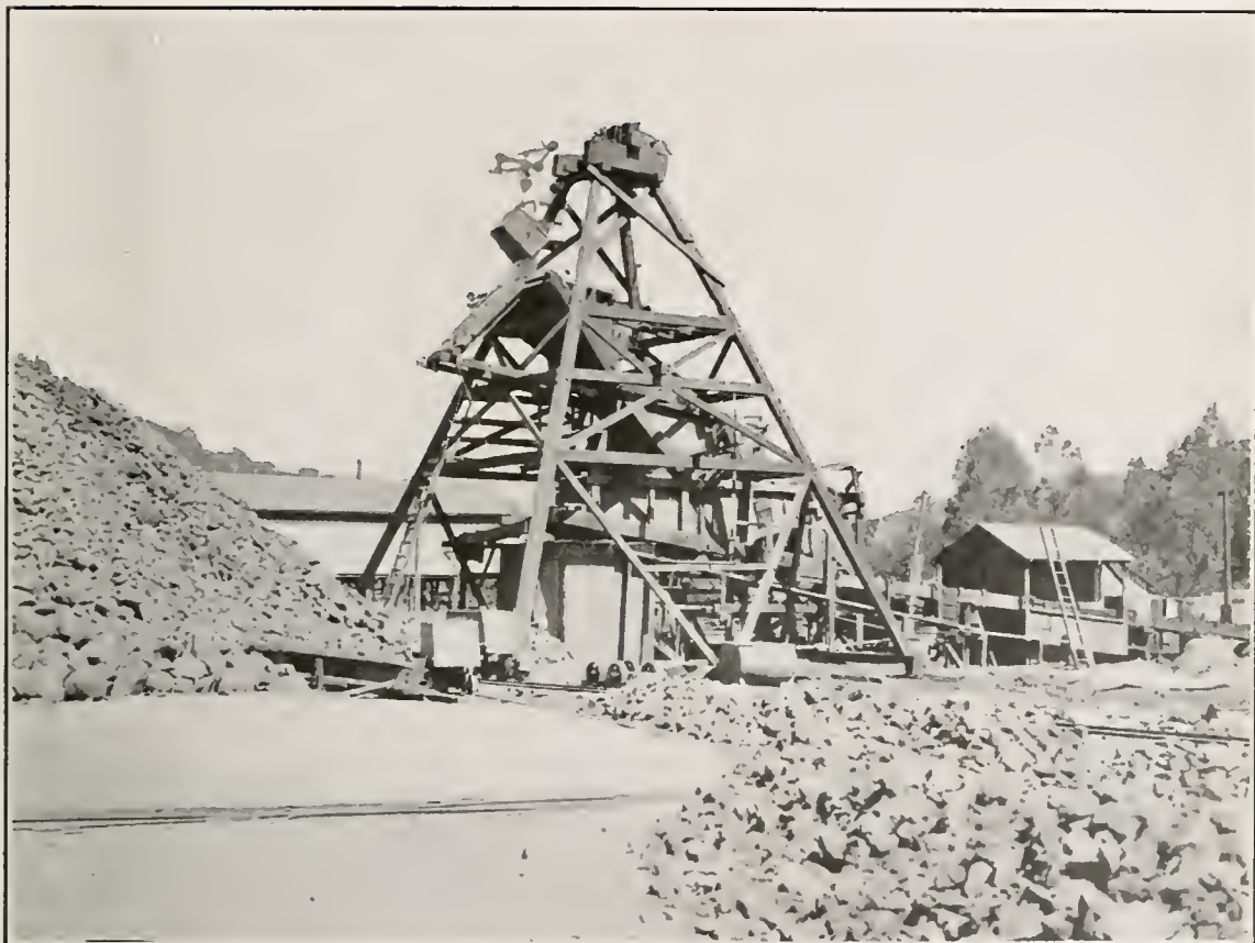
Photo No. 77. Gravel-washing plant for recovering metallic quicksilver from material excavated from old furnace sites, at Hacienda of New Almaden Company, Santa Clara County.
