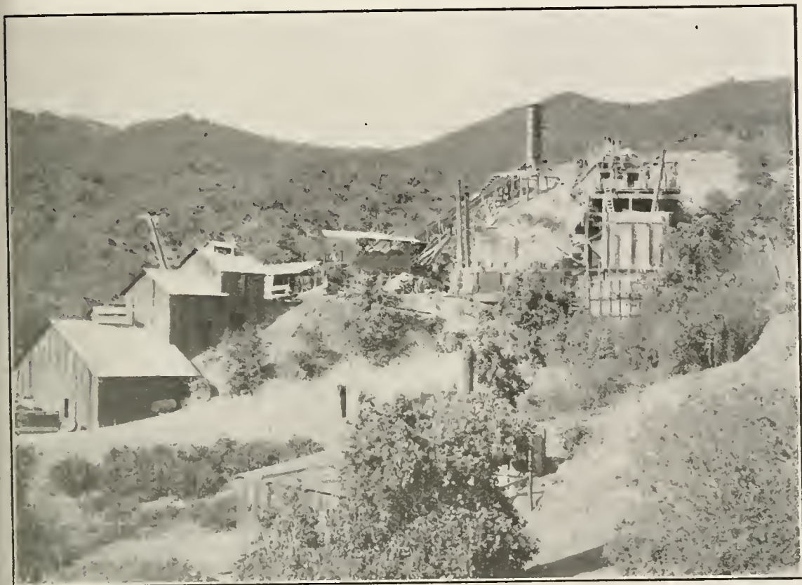
Photo No. 15. Furnaces at La Joya Mine, Napa County. Fitzgerald furnace in buildings at left; Livingston at right; and retorts on bench between.
