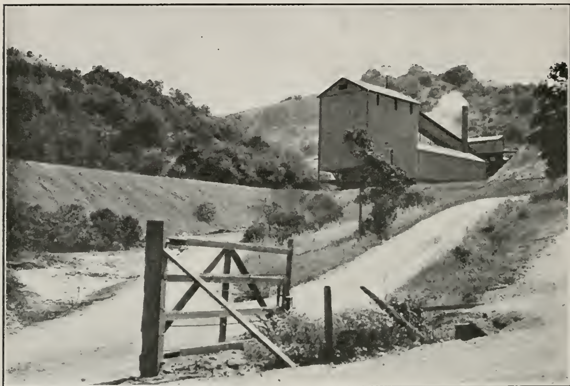
Photo No. 35a. New 90-ton Scott furnace at Senator Mine of New Almaden Company.
