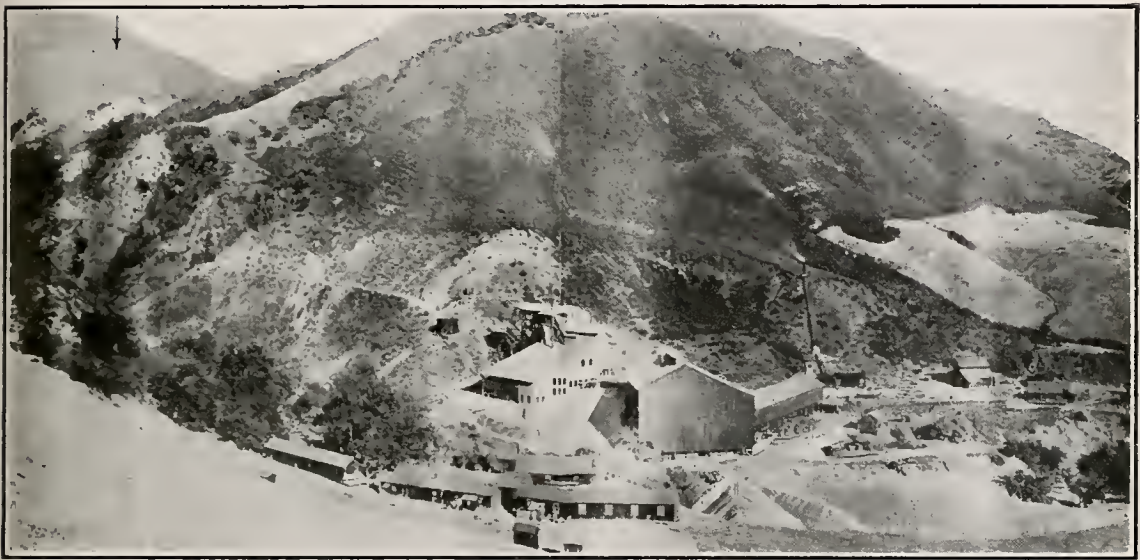
Photo No. 31. Plant of Oceanic Mine, San Luis Obispo County. The light streak below the arrow is the line of the open cuts.
