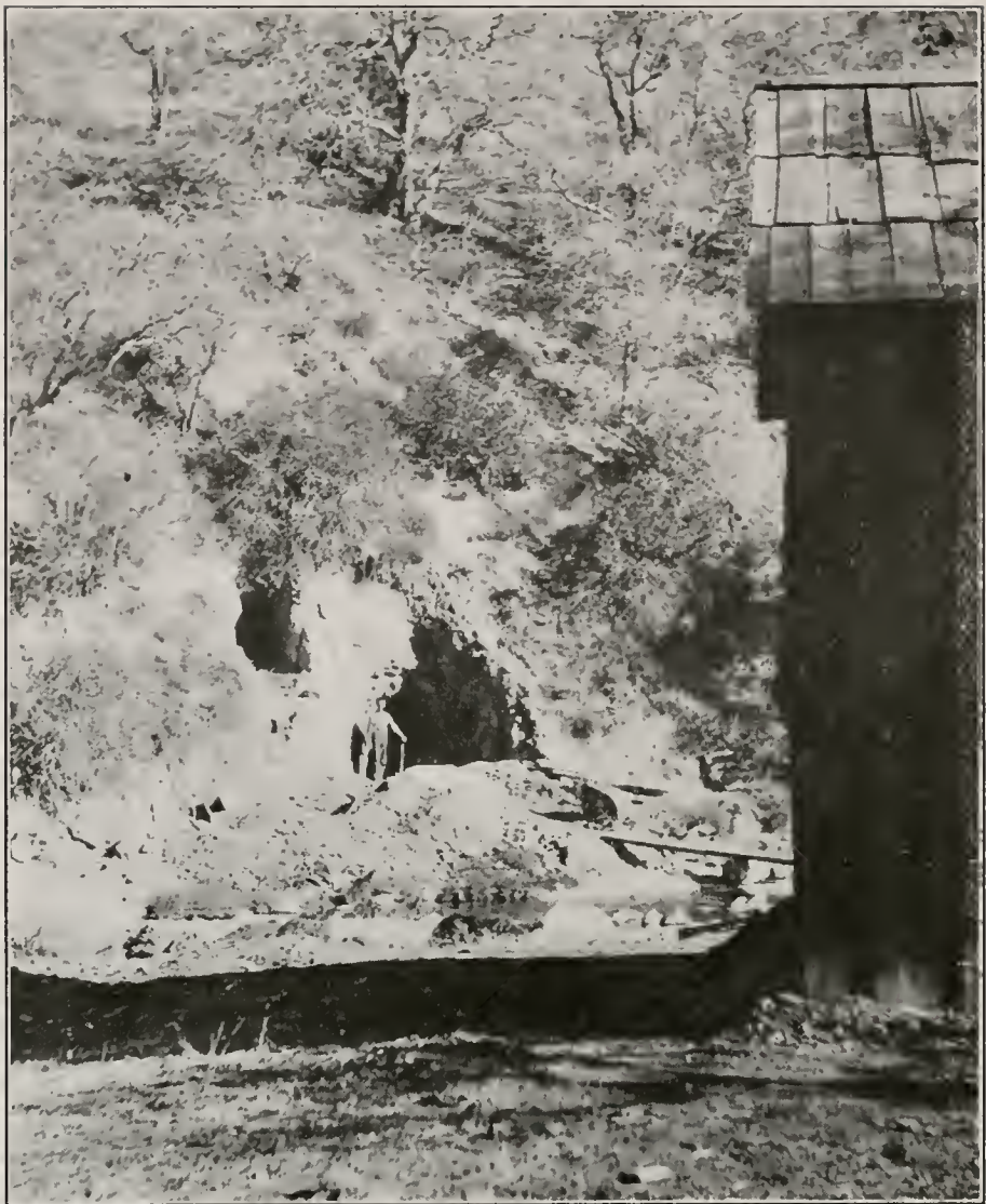
Photo No. 19. Old and new prospect tunnels, Florence Mack Mine. The old (upper) tunnel was a few feet too high and failed to uncover the vein; the lower tunnel showed a fair prospect of cinnabar. Photo by C. A. Logan.
