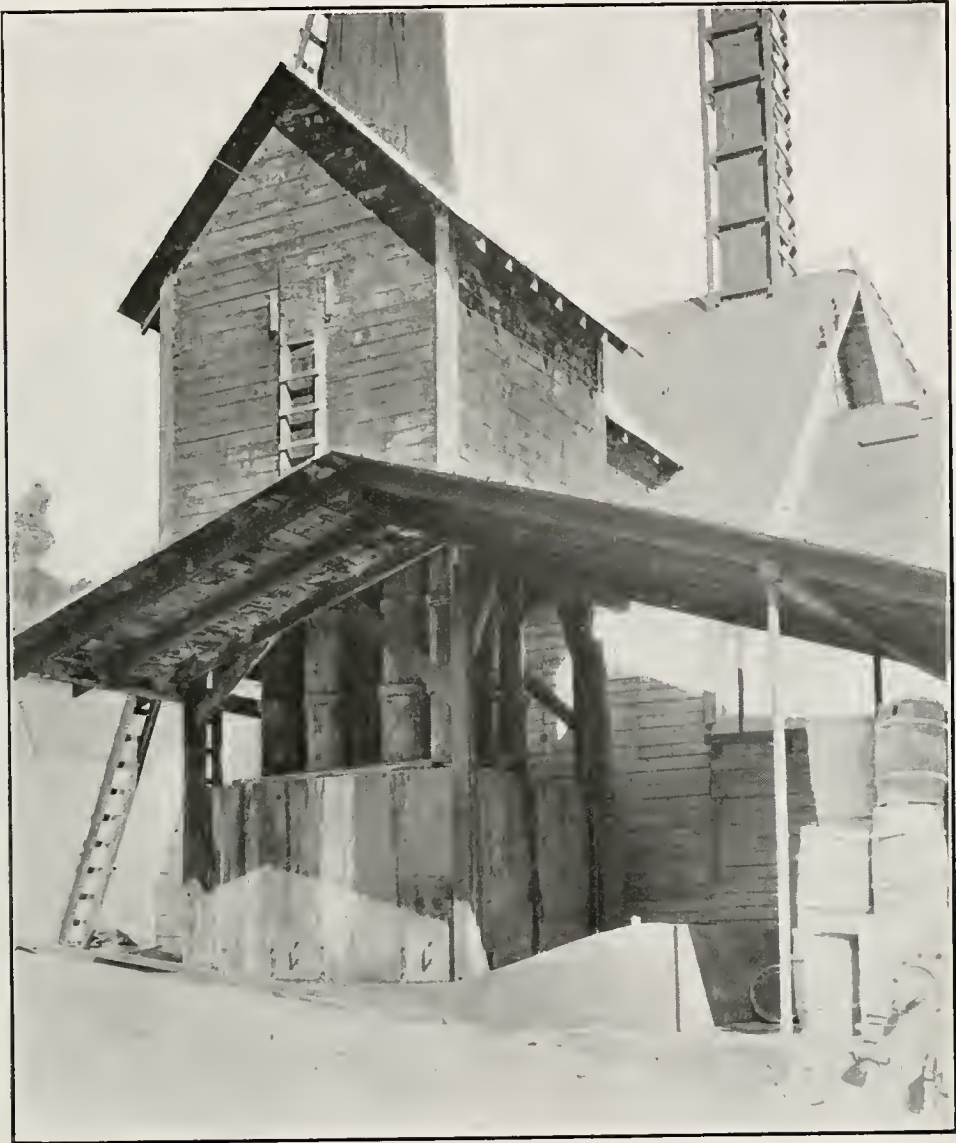
Photo No. 55. Cottrell Precipitator, or 'Cold Treater,' at Senator Mine.
