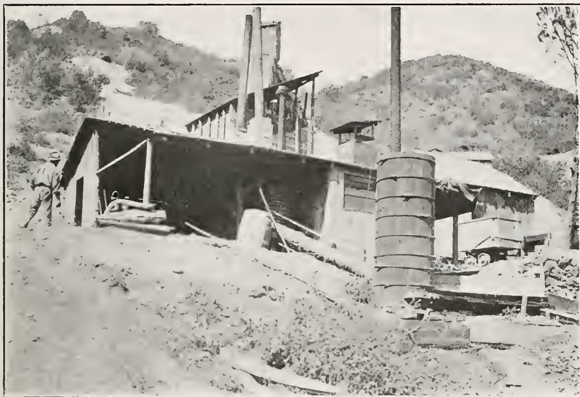
Photo No. 8. Retorts and condensers at the Big Injun Mine, near Middletown, Lake County.
