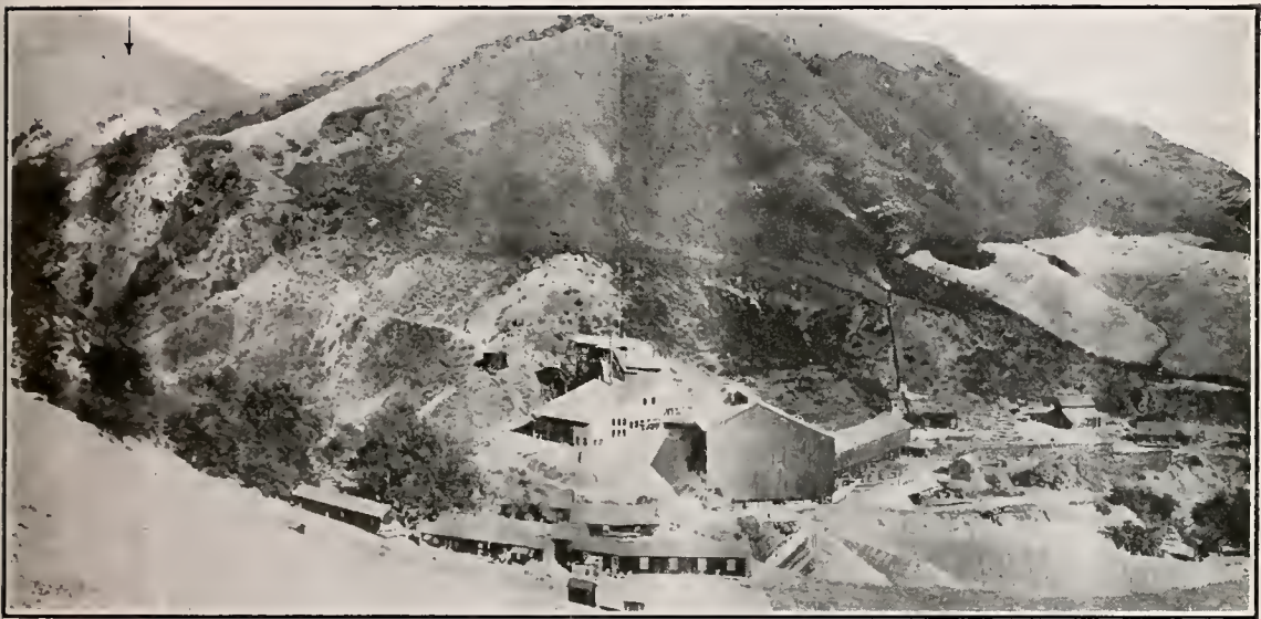
Photo No. 31. Plant of Oceanic Mine, San Luis Obispo County. The light streak below the arrow is the line of the open cuts.
