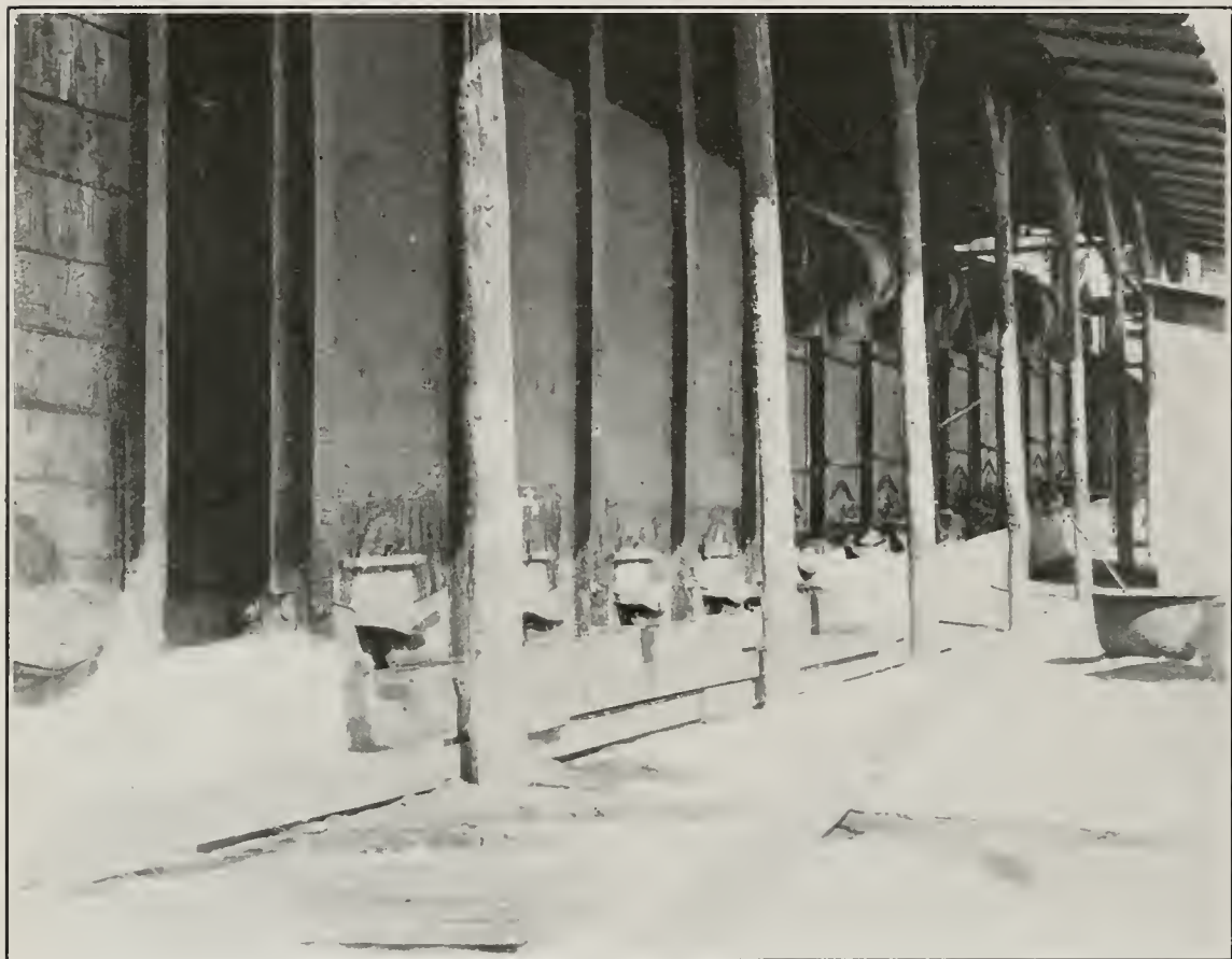
Photo No. 64. Condensers and Vitrified-pipe Flues at Aetna Mine, Napa County.
