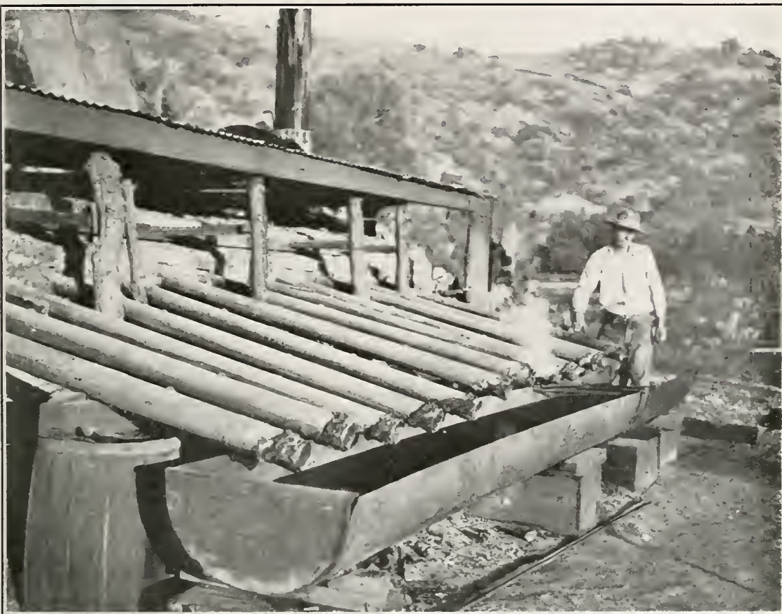
Photo No. 62. Condenser Pipes of Johnson-McKay Retorts at Patriquin Mine, Monterey County.
