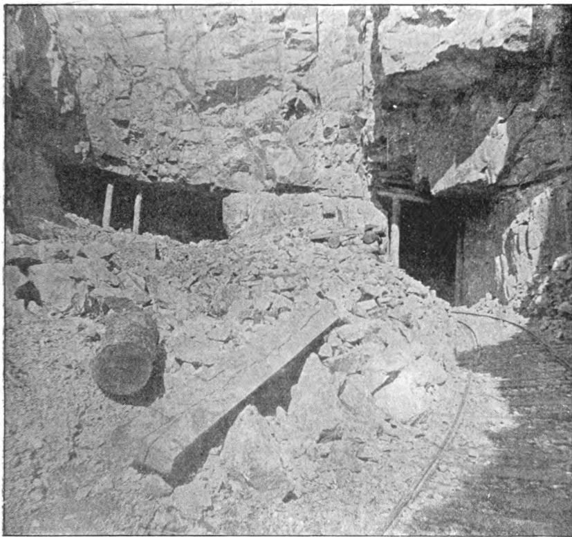
FIG. 29.—View of open cut at Pilot Knob, Mo., showing the bedded character of the iron ore. From a photograph by J. F. Kemp, 1888.
