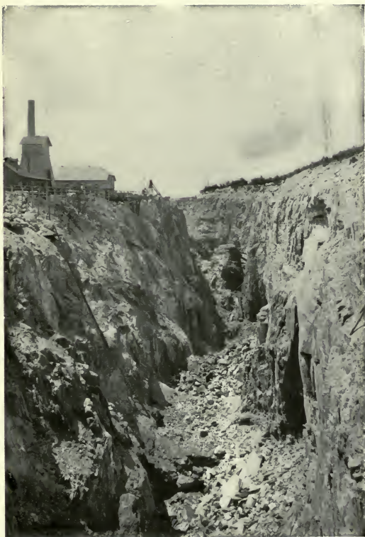
FIG. 37.—Open cut at Minnesota Iron Company's Mine, Soudan, near Tower, in south view looking west. Photograph by J. F. Kemp, 1894.
