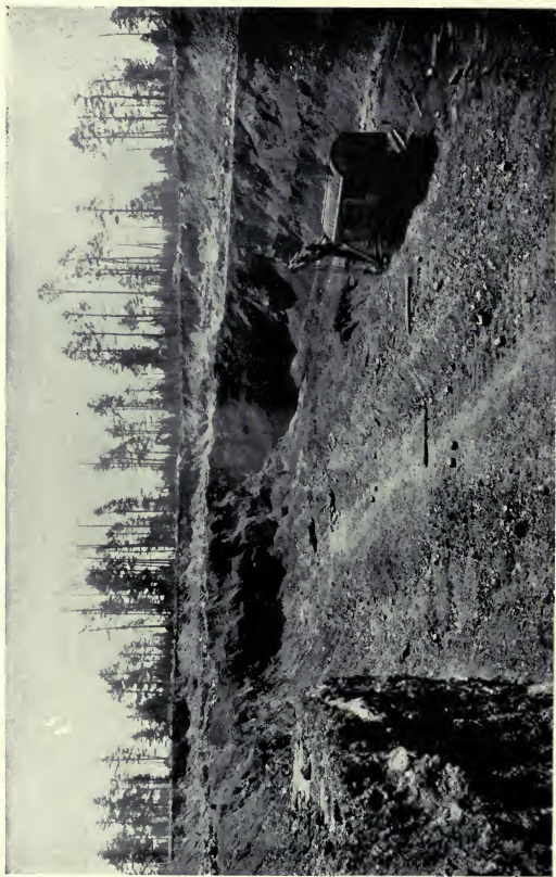
FIG. 41.—View of the Mesaba Mountain or Oliver Mine, Virginia, Minn., looking southeast. The view shows the overlying gravels and the ore. From a photograph by J. F. Kemp, 1894.
