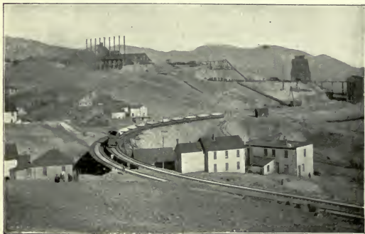
FIG. 61.—View of the Anaconda Mine (with the nine stacks), Butte, Mont. From a photograph by Alexander Brown, E. M., 1896.
