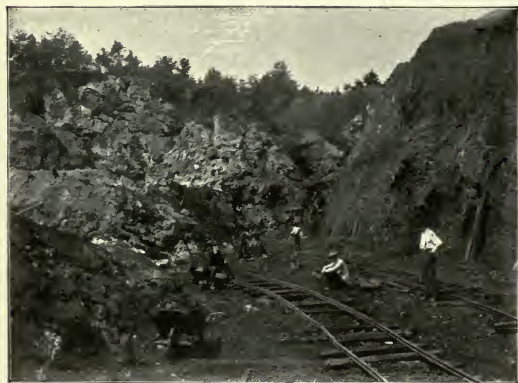
FIG. 83.—View of open cut in the Wythe Zinc Mines, Va. From a photograph by J. F. Kemp, 1895.
