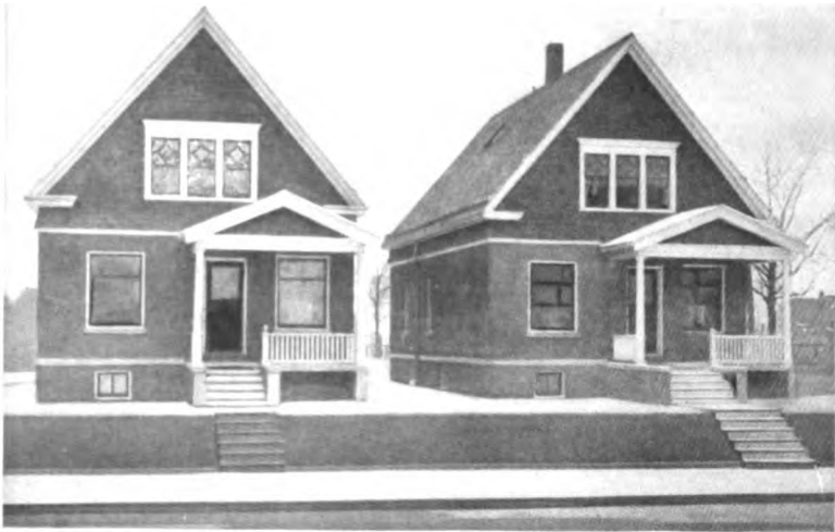
WORKINGMEN'S HOUSES BUILT OF SOLID REINFORCED CONCRETE.
