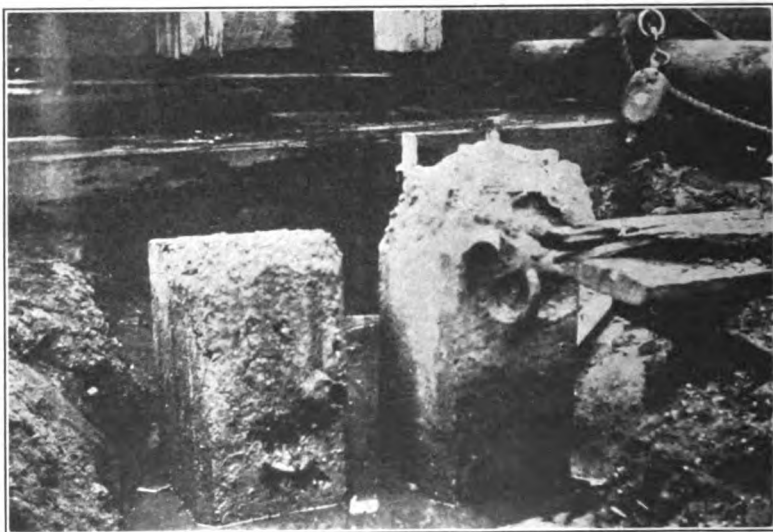
FIG. 194.—Completed piles after driving.
