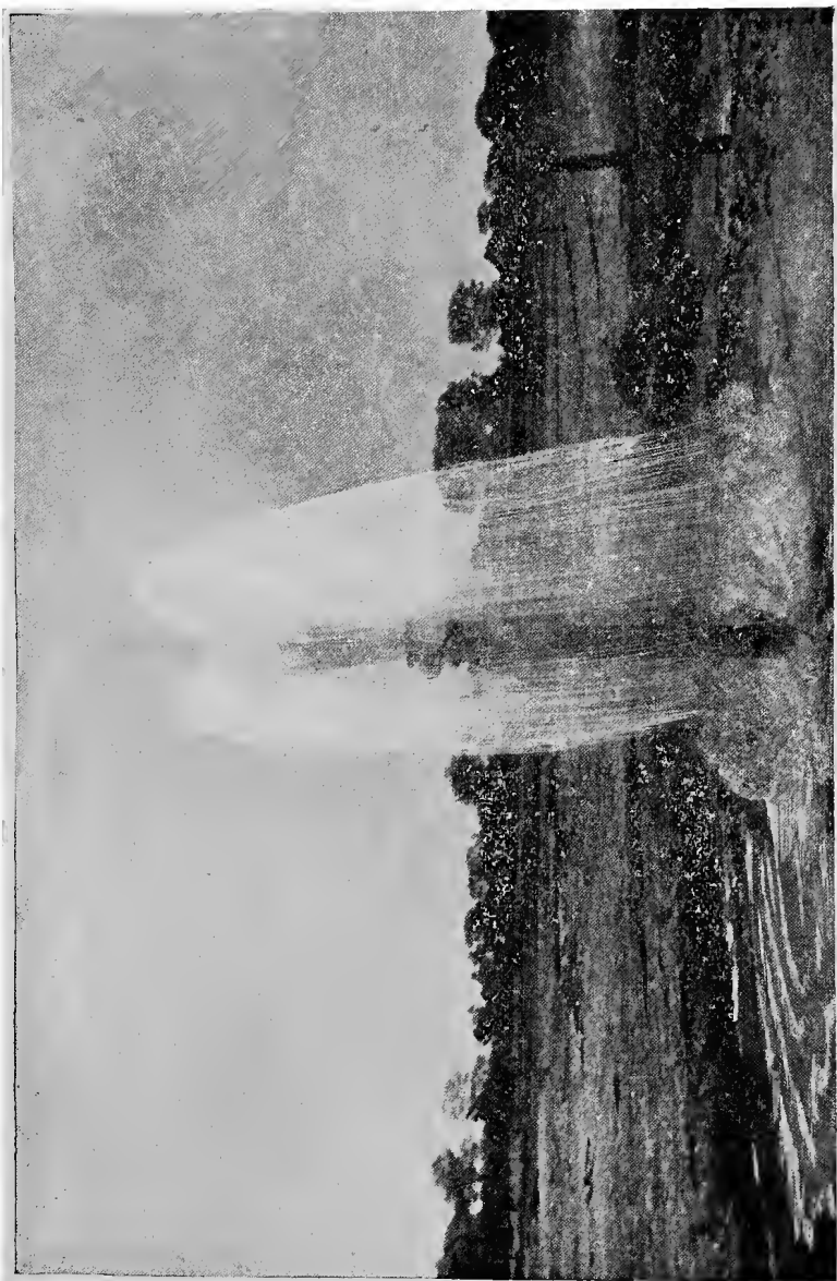
KERRIBREE, BOURKE DISTRICT, NEW SOUTH WALES. DEPTH, 1,840 FEET; FLOW, 1,700,000 GALLONS DAILY; TEMP., 100 DEG. FAH.
