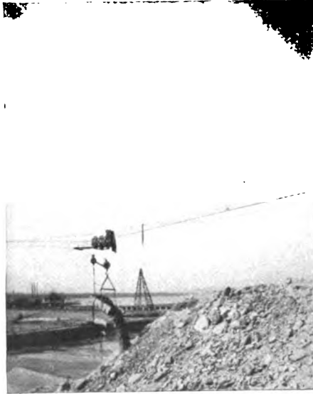
FIG. 48.—Detroit River Cofferdam.
