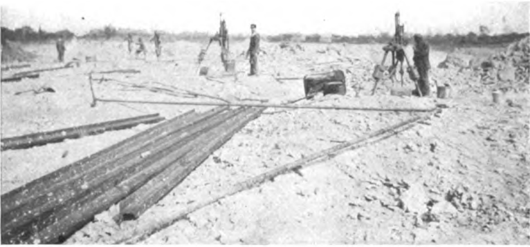
FIG. 72.—Drilling Top Holes—Thornton Quarry.
