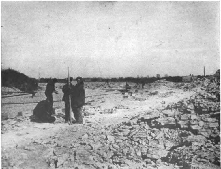
FIG. 73.—Loading Top Holes—Thornton Quarry.
