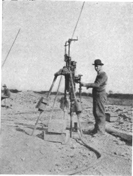
FIG. 70.—Drilling Top Holes—Thornton Quarry.
