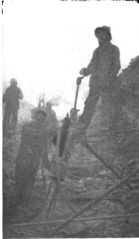
FIG. 55.—Tripod Drill at Vail, N. J.
