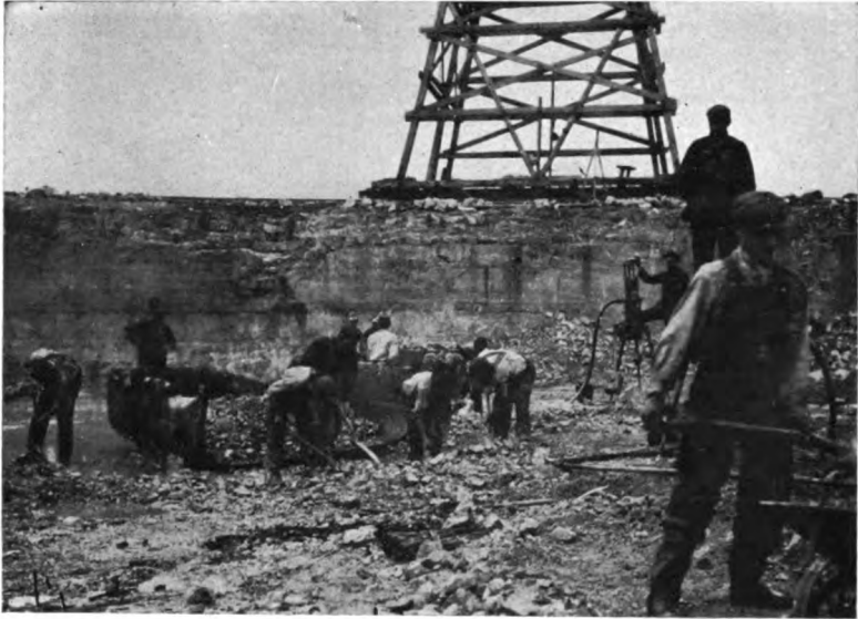
FIG. 46.—Loading by Hand into Skip.
