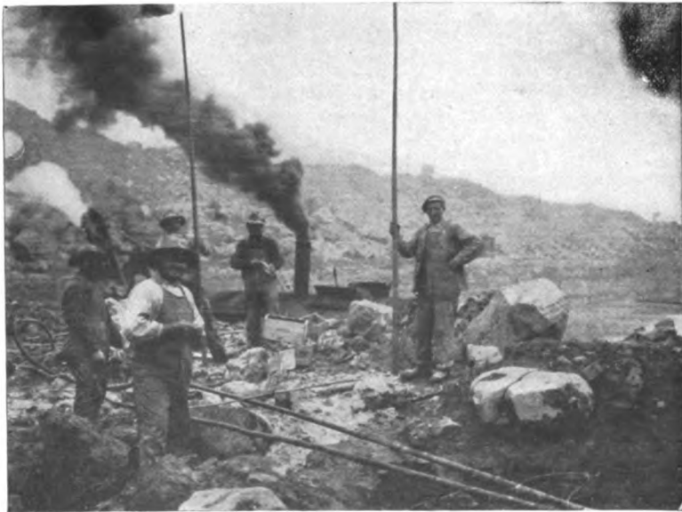
FIG. 41.—Loading Holes for Blasting, Livingstone Improvement.
