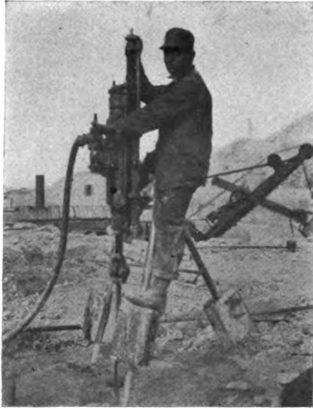
FIG. 36.—Drill at Cofferdam B.
