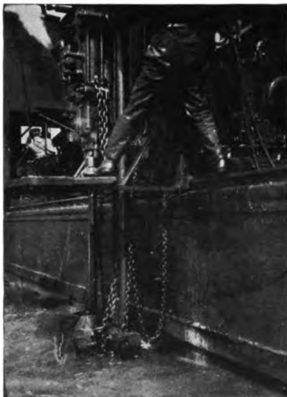
FIG. 115.—Foot of Drill Frame: Buffalo Boat No. 5.
