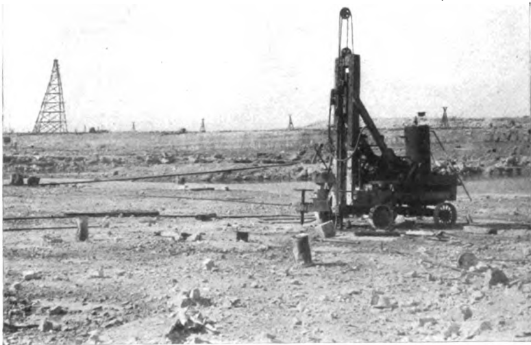
FIG. 43.—Traction Drill.
