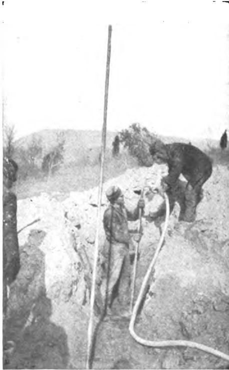
FIG. 67.—Blowing Out Holes.
