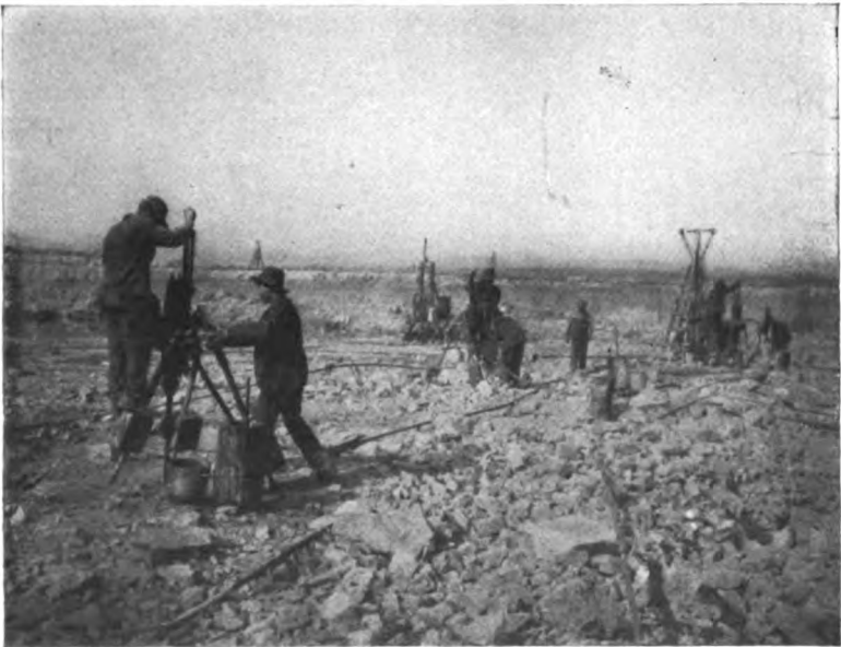
FIG. 37.—Drilling at Cofferdam B.
