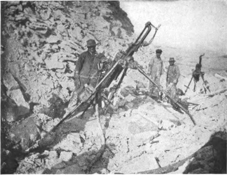
FIG. 68.—Drilling Toe Holes—Thornton Quarry.
