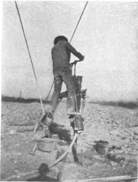
FIG. 71.—Drilling Top Holes—Thornton Quarry.
