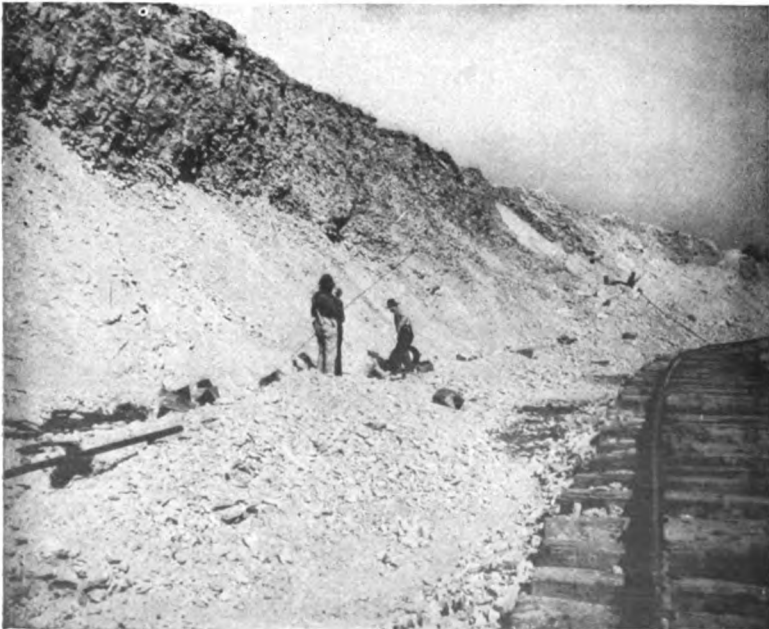
FIG. 69.—Loading Toe Holes—Thornton Quarry.
