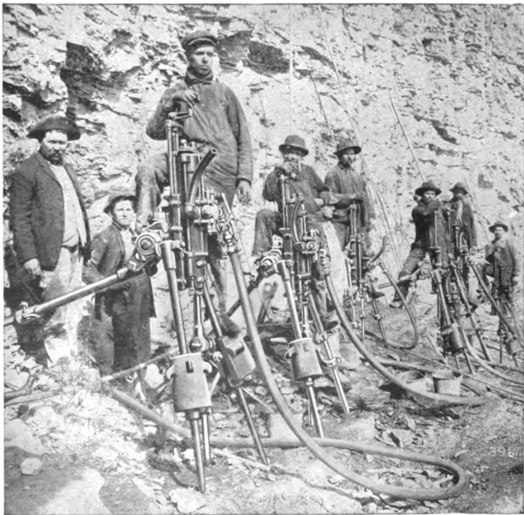
FIG. 5a. Power is conveyed to these rock drills by means of compressed air transmitted through pipe lines. The Ingersoll-Rand Co.
