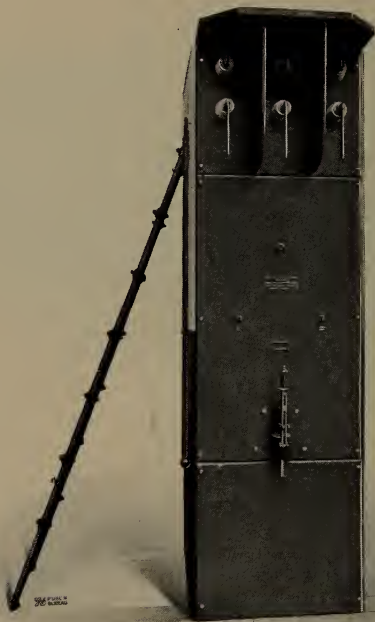
Fig. 7 FRONT OF HIGH TENSION FLOOR PANEL
