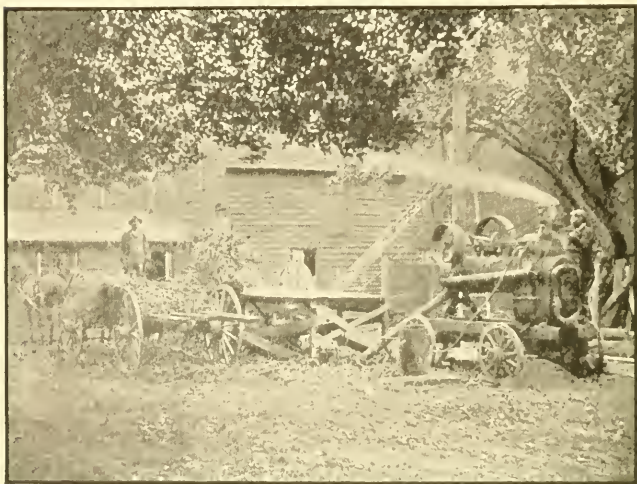
Fig 39—Filling the Silo
