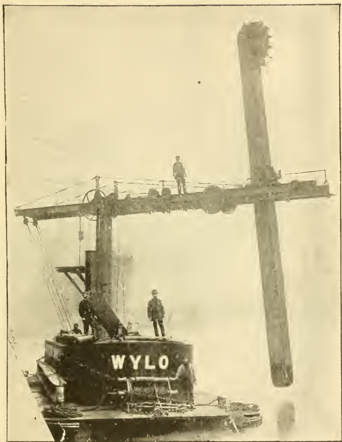
Fig 57—Floating Grain Elevator Used to some extent at English seaports
