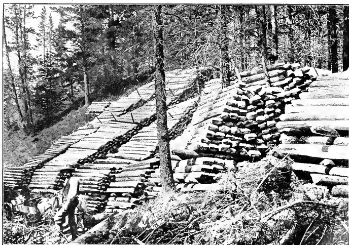
FIG. 2.—TIE PILES AT THE FLUME.
