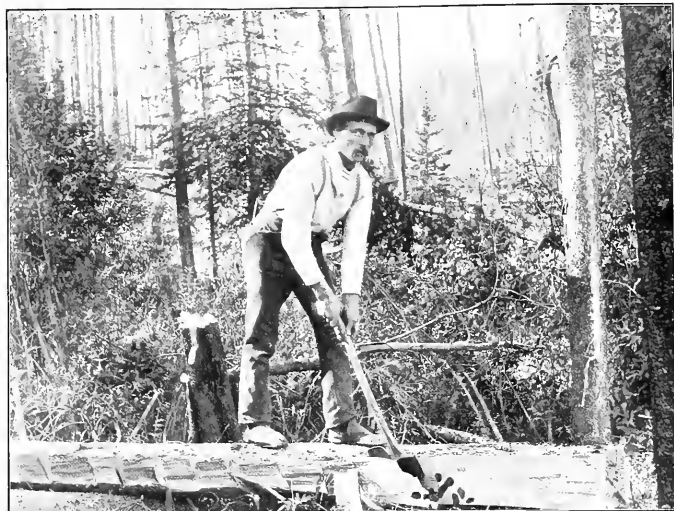
FIG. 1.—TIE CHOPPER MAKING TWO STRAIGHT FACES ON THE STICK.
