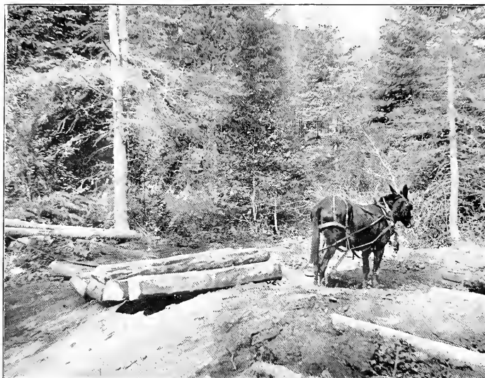
FIG. 1.—DRAGGING TIES TO THE FLUME.
