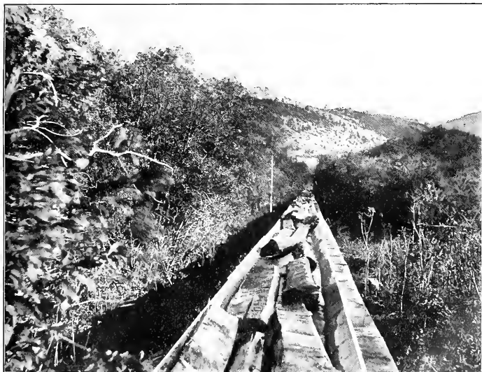
FIG. 2.—ANOTHER VIEW OF FLUME.
