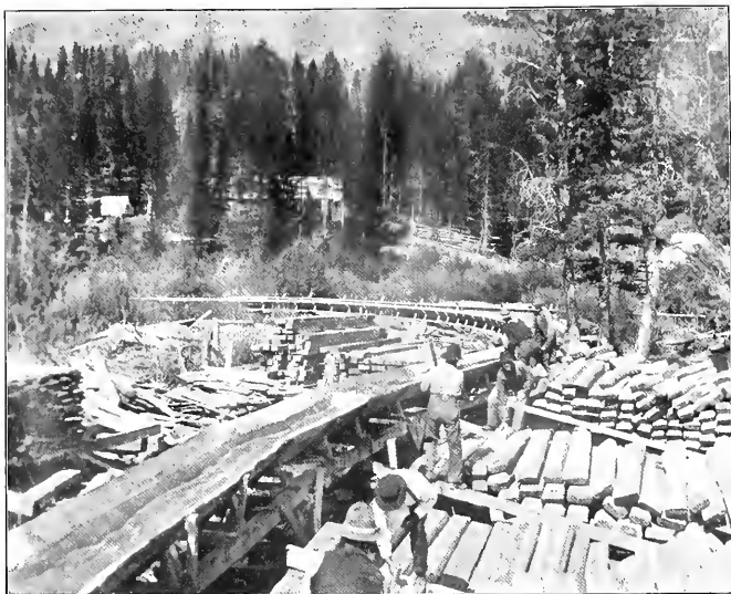
FIG. 1.—THROWING TIES INTO THE FLUME.
