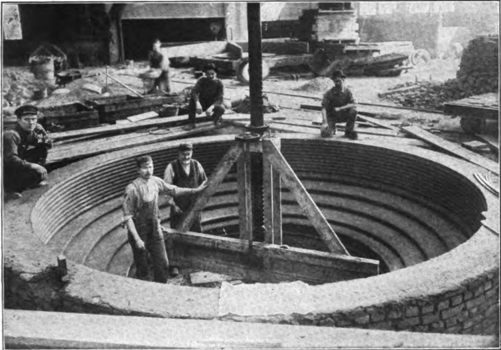
FIG. 13. MOLD WITH SWEEPING RIG IN PLACE.
