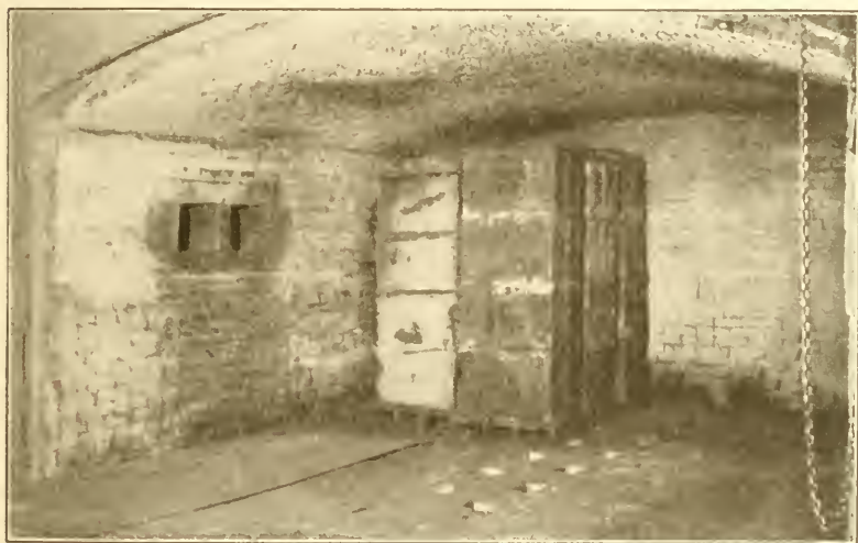
Fig. 168. Interior View of Annealing Oven
