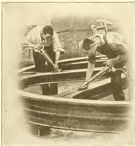
Fig. 140. Pneumatic Chisel for Cutting Risers and Fins
