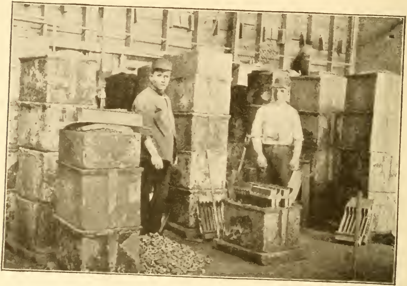
Fig. 166. Packing Annealing Boxes
