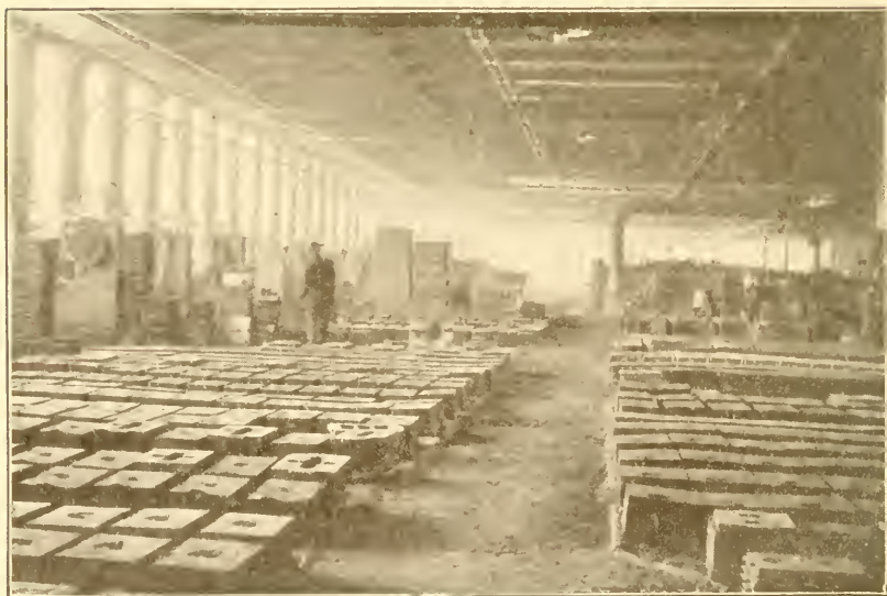
Fig. 154. Molds in Position for Pouring
