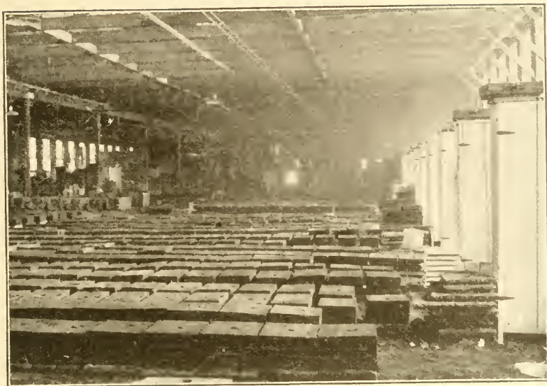
Fig. 155. View of Molding Floor, Fig. 154, Taken from Opposite End of Plant
