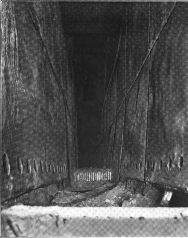
FIG. 5. — Washoe Blast Furnace. (Interior.)
