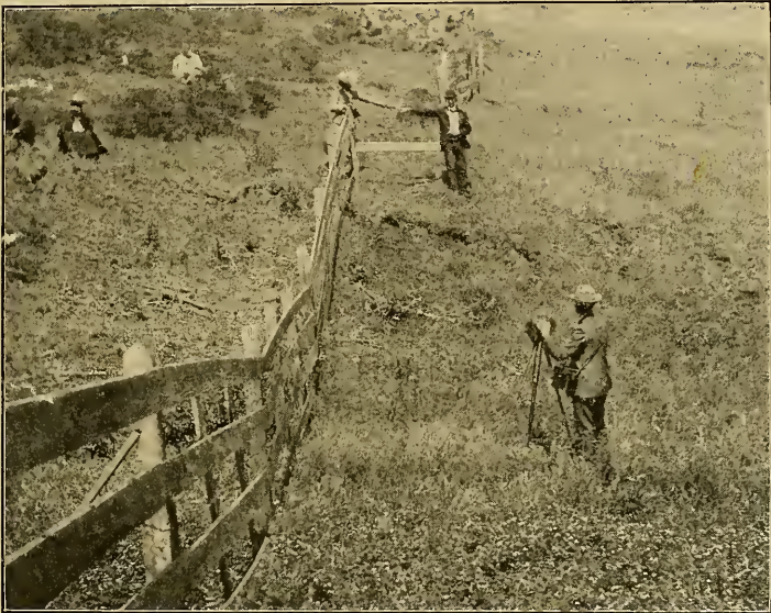
LATERAL DISPLACEMENT, SAN FRANCISCO EARTHQUAKE
