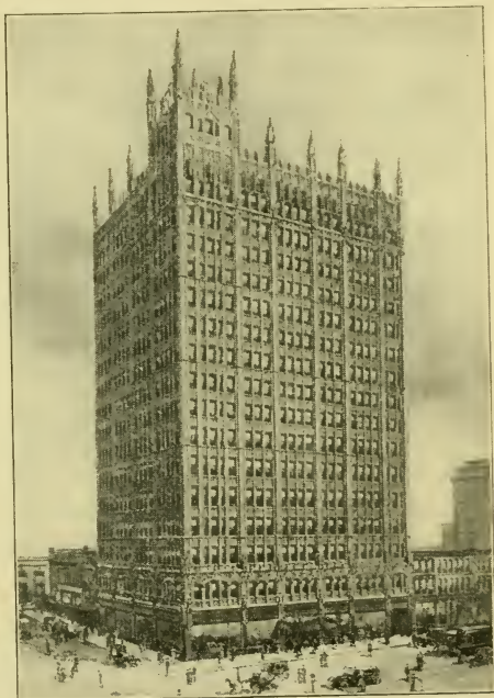
FIG. 105. THE BUSCH BUILDING, DALLAS Eighteen stories high
