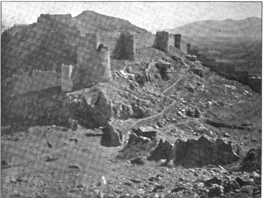
FIG. 240. Outer wall of Kabul, capital of Afghanistan.
