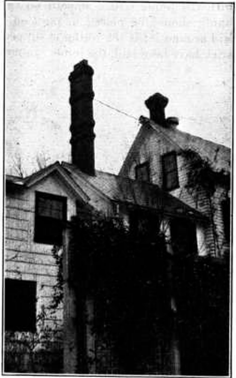
FIG. 3.—Extensions to the chimney required in order that it might draw properly.
