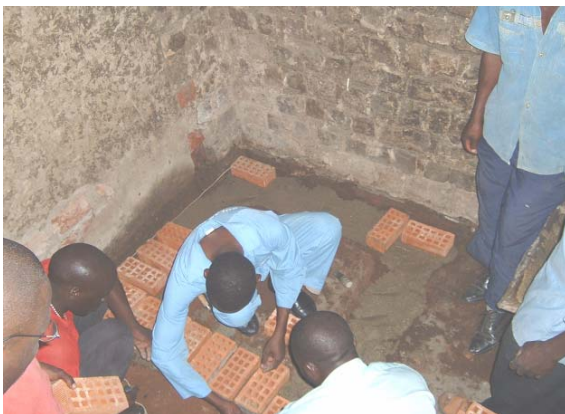
Photo 5: Construction of the foundation
