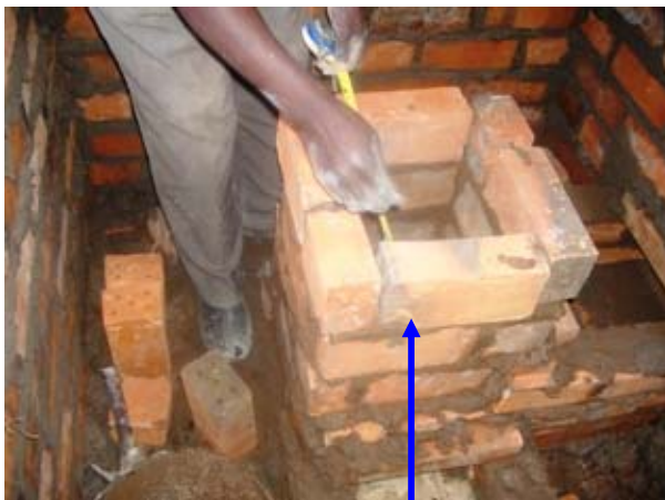
Photo 8: Combustion chamber construction
