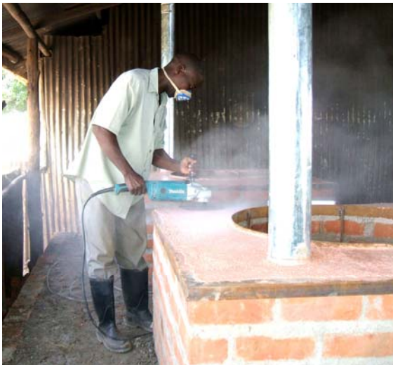
Photo 18: Grinding a stove with a terrazzo finish
