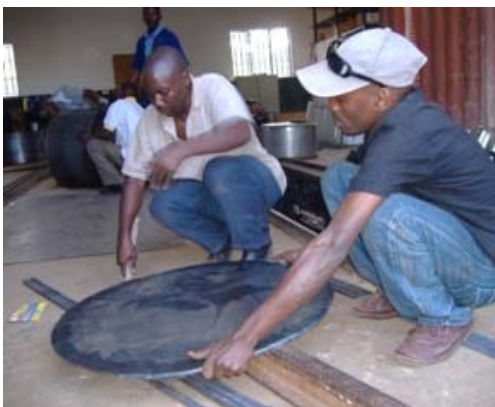
Photo 26: Bending a base plate
