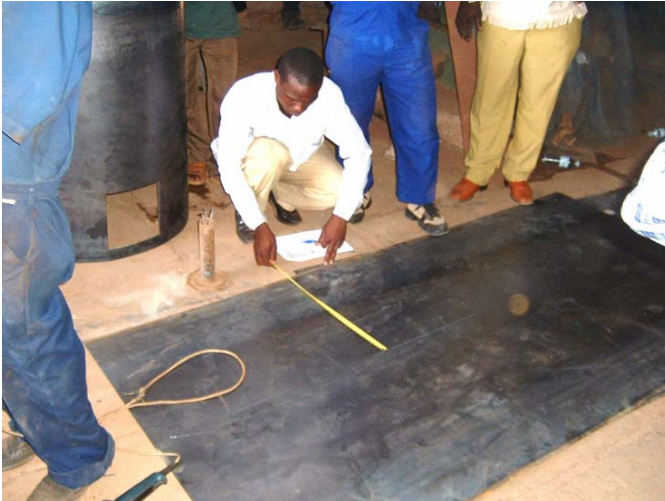
Photo 19: Marking off measurements
