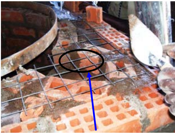
Photo 15: The provision of the chimney
