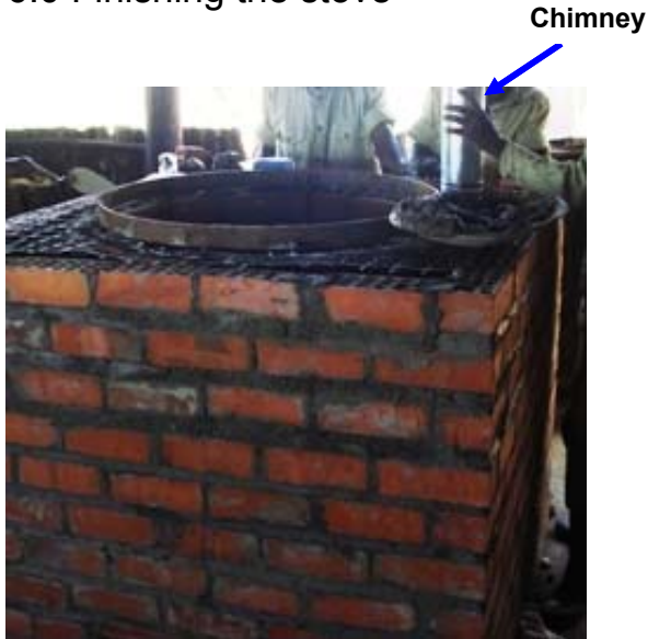
Photo 16: Fixing the chimney pipe
