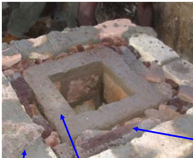
Photo 9: combustion chamber building
