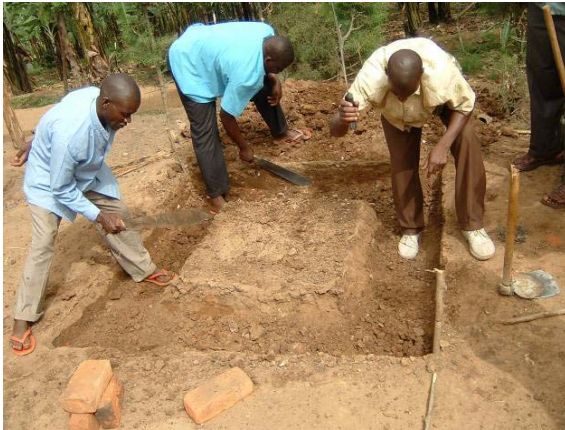
Photo 4: Digging the foundation
