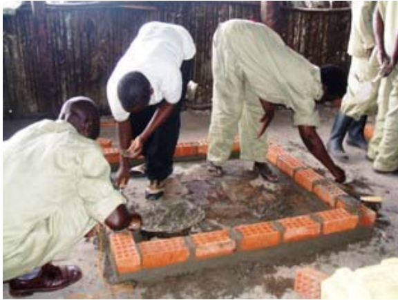
Photo 6: construction out on a concrete slab
