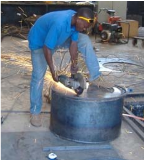
Photo 28: Using an angle grinder with a metal cutting disc to cut out a hole in the base plate
