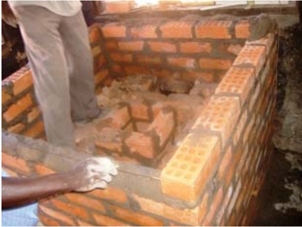
Photo 9: combustion chamber building
