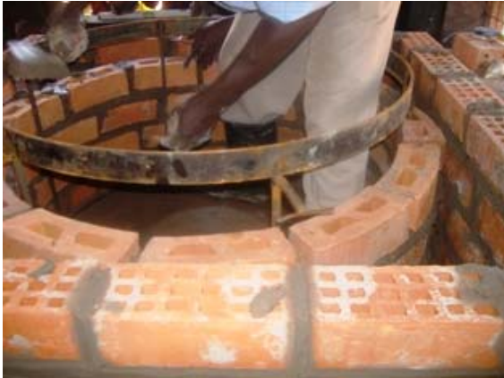
Photo 14: Construction of the saucepan skirt
