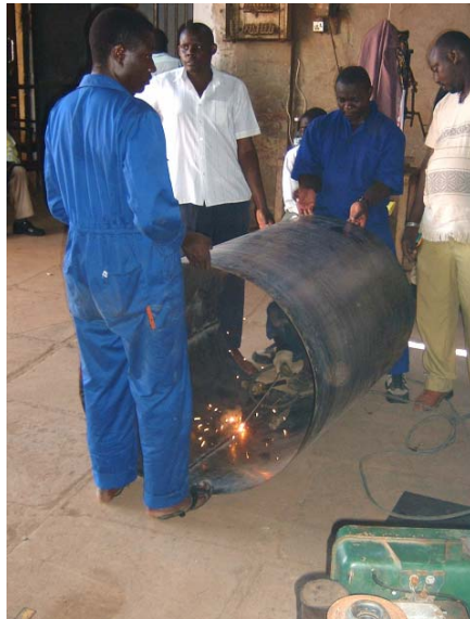
Photo 23: Welding the rolled metal sheet
