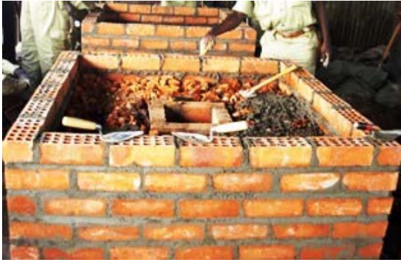
Photo 11: filling the stove body with debris
