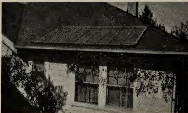
Fig. 21.—A commercial-type solar heater absorber. This absorber was mounted on the south side of the house, in a place where it was protected from winds and free from shade.
