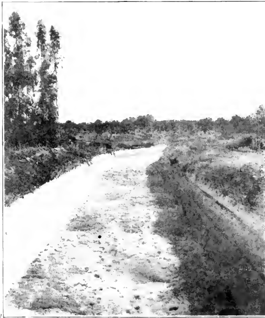
Fig. 148. Riverside Canal, California. Sand deposit left on bottom after a year's service. Courtesy of "Engineering News."
