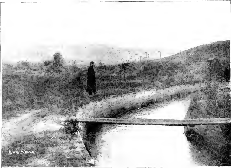
Fig. 147. Santa Ana Canal, California. Gravel concrete lining.
